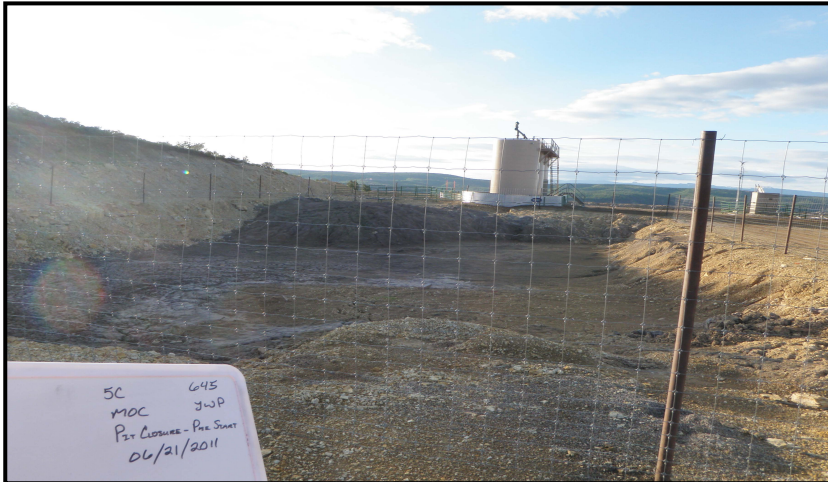
Photo 1 – 696-5C reserve pit containing drill cuttings.
