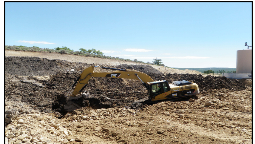
Photo 4 – Track hoe mixing pit contents with clean material within pit.
