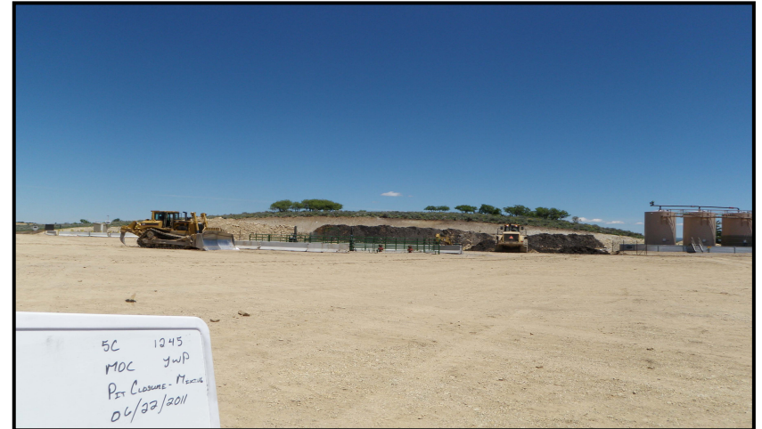
Photo 2 – Loader providing clean fill material from SW corner to track hoe for mixing.
