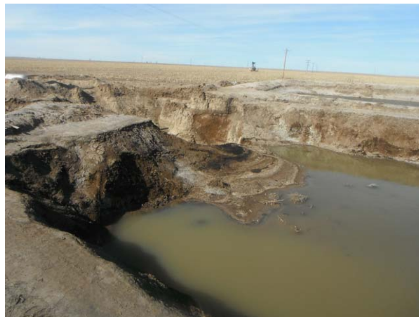
Breached wall and existing evaporation pit
