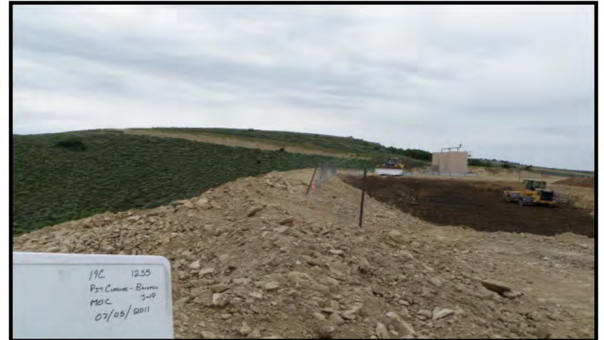
Photo 6 – Pit during backfilling operations.
