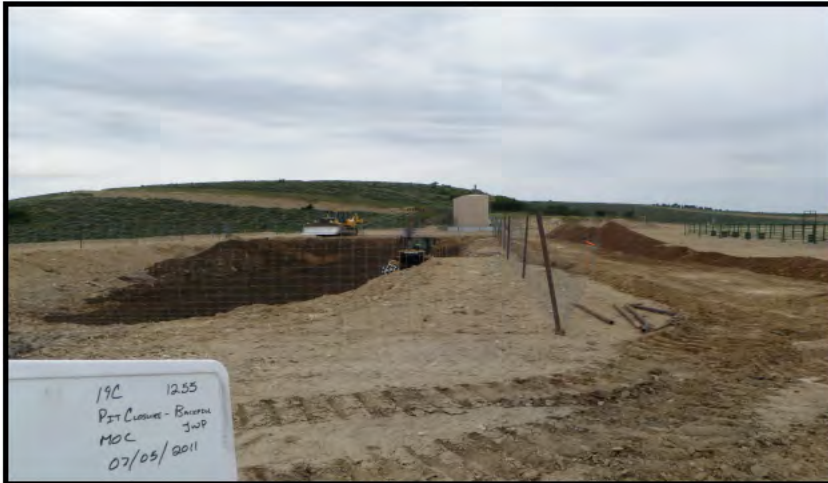
Photo 5 – Compactor and D8 rolling material while backfilling to achieve homogenous mixture.
