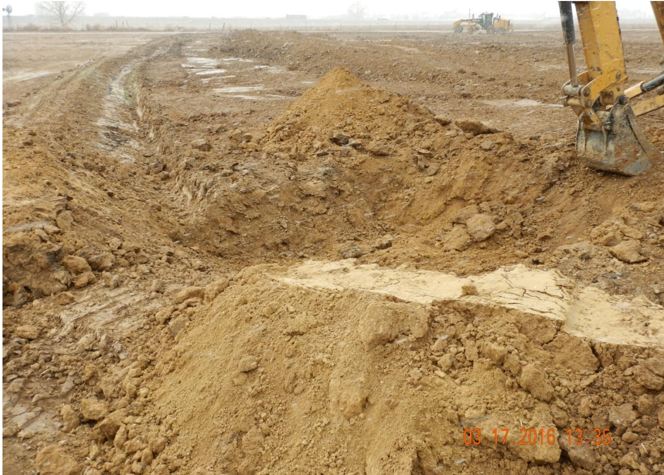
Photo 1. Photo taken from southeast location, facing West. Stormwater and sediment control BMPs installed in center of photo (berm and ditch). Sediment trap under construction.
