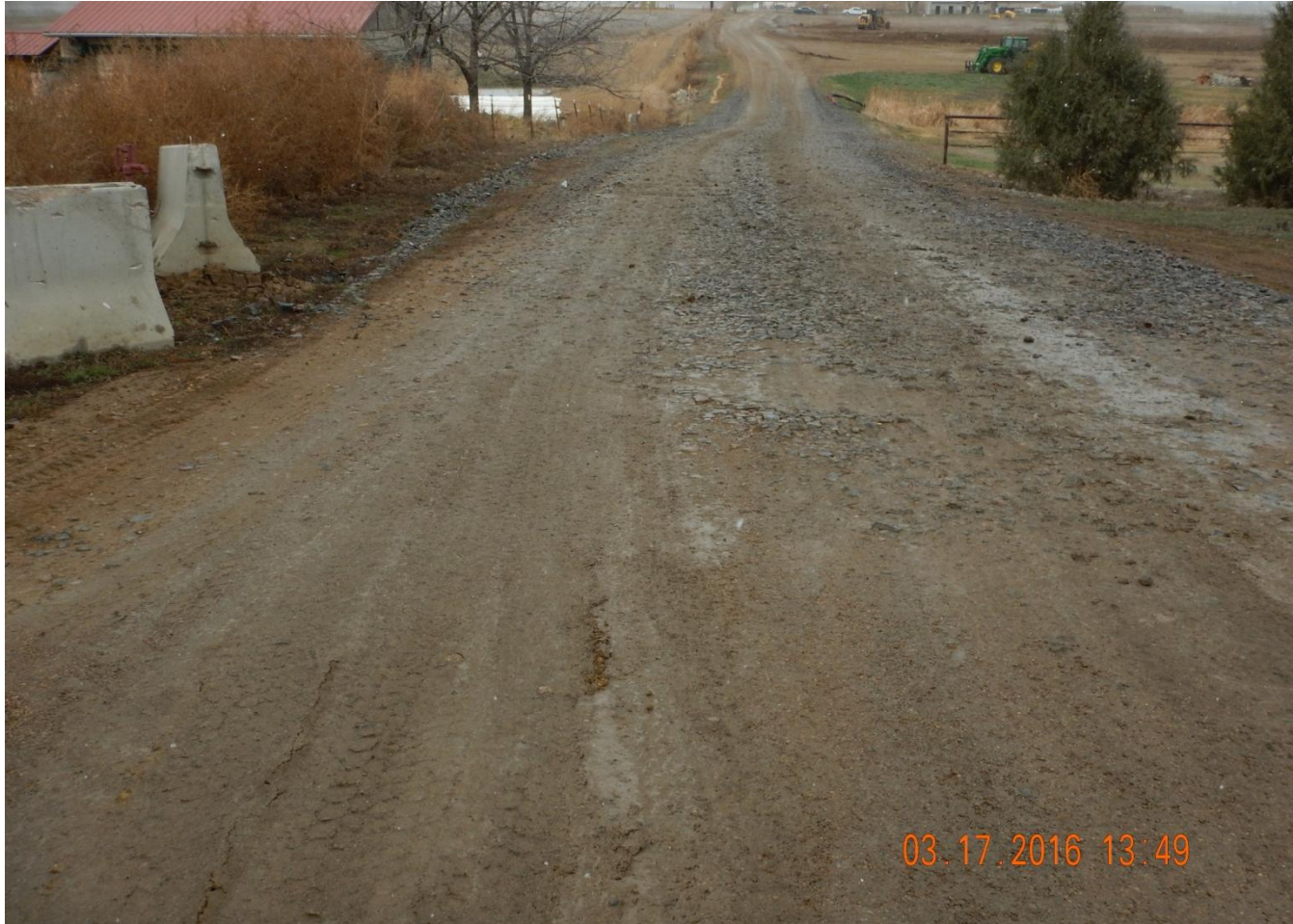
Photo 8. Photo taken from entrance of location, facing North. Vehicle tracking pad in place. May need to fluff vehicle tracking pad to minimize sediment leaving location.
