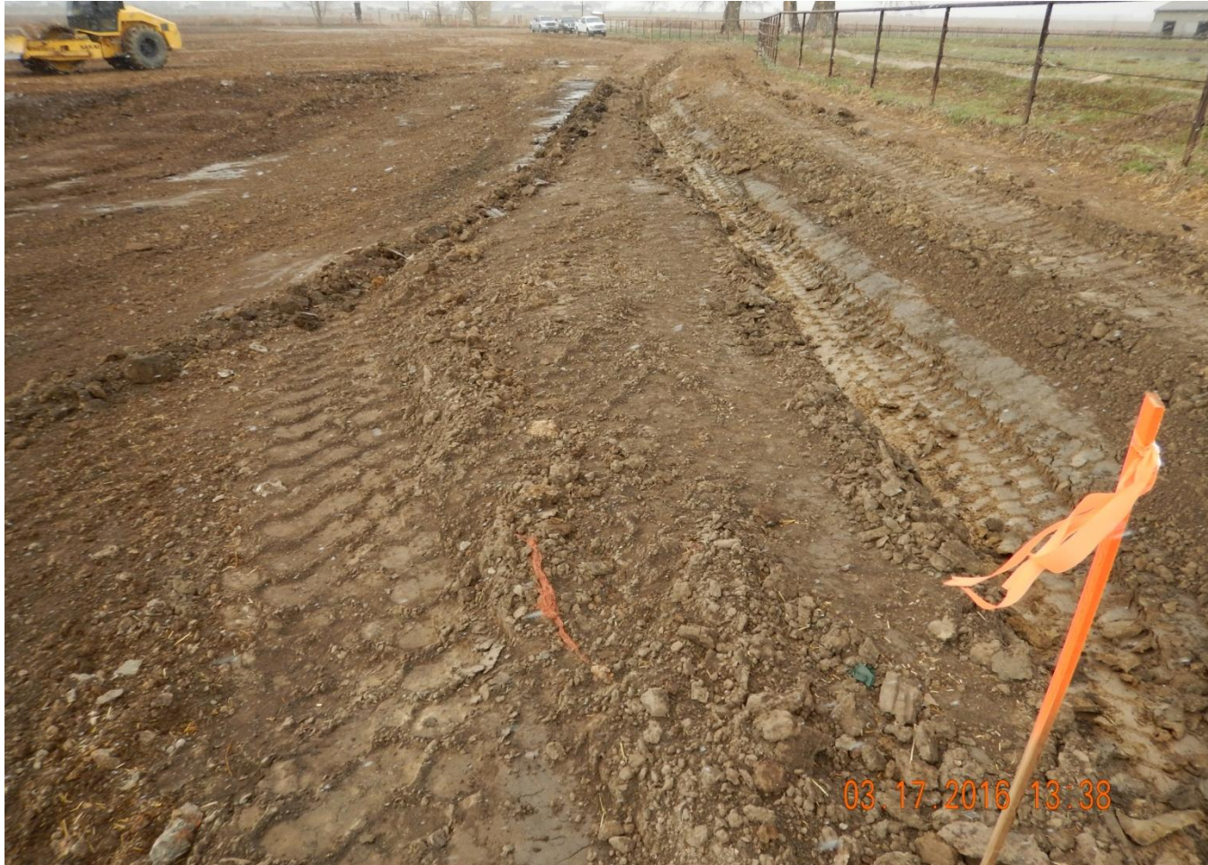
Photo 4. Photo taken from northeast location, facing West. Stormwater and sediment control BMPs installed in center of photo (berm and ditch).
