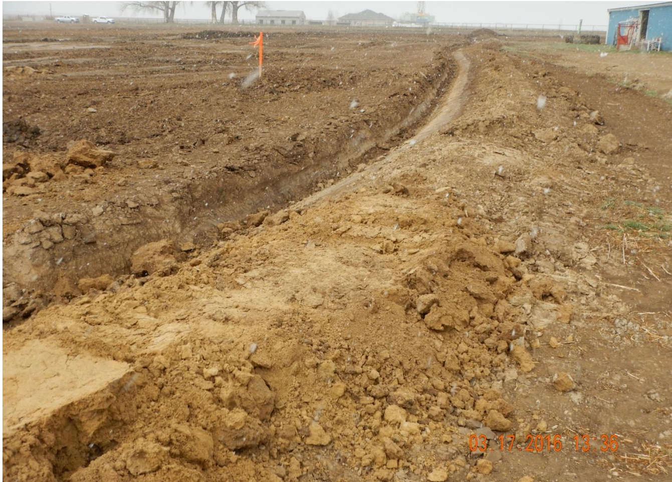
Photo 2. Photo taken from southeast location, facing North. Stormwater and sediment control BMPs installed in center of photo (berm and ditch).
