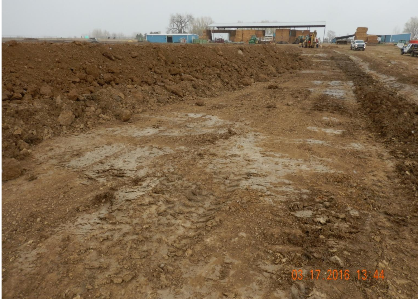
Photo 7. Photo taken from southwest location, facing Northeast along topsoil stockpile. Need to stabilize topsoil stockpile upon completion of construction activities.
