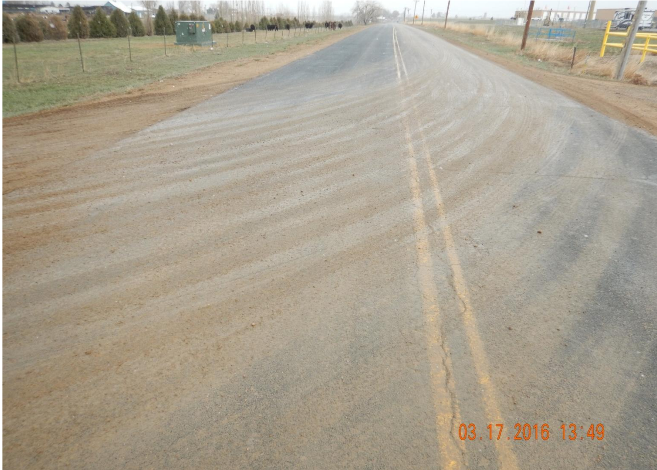
Photo 9. Photo taken from entrance of location, facing East along Adams Avenue. May need to fluff vehicle tracking pad to minimize sediment leaving location and/or street sweeper to control potential sediment discharges if sediment accumulates on Adams Avenue.
