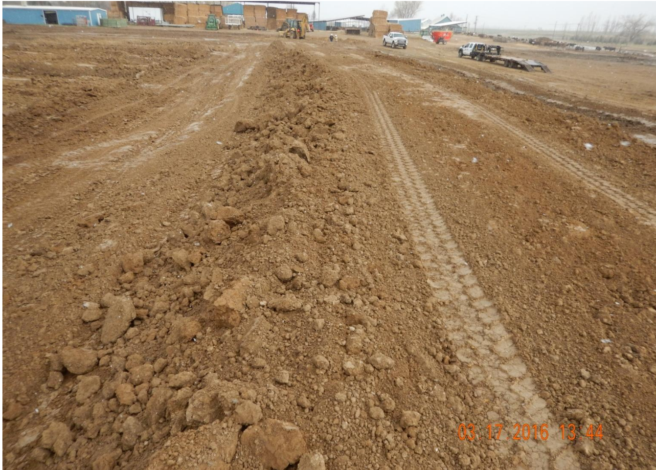
Photo 6. Photo taken from southwest location, facing East along topside of topsoil stockpile. Need to stabilize topsoil stockpile upon completion of construction activities.
