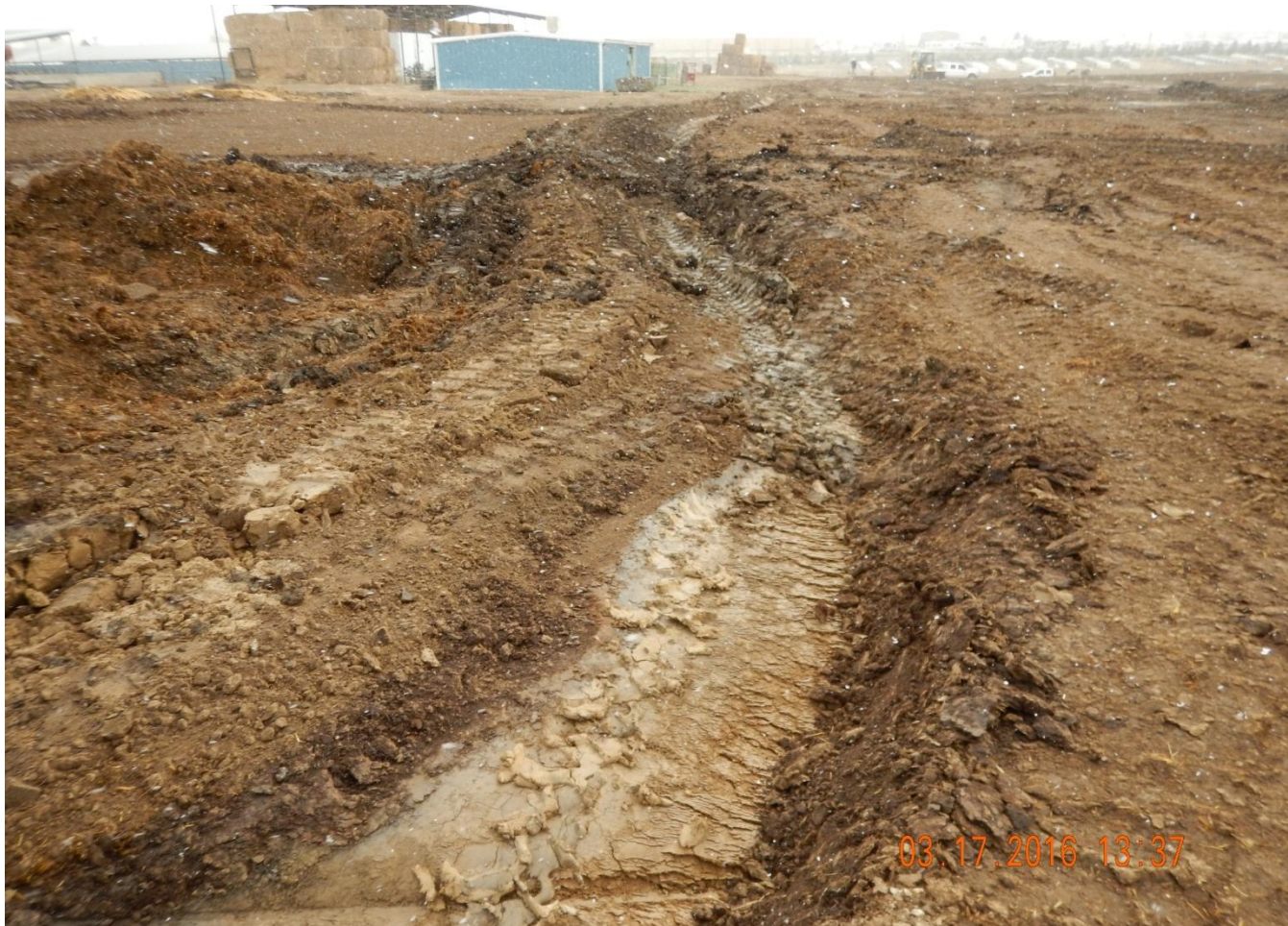
Photo 3. Photo taken from northeast location, facing South. Stormwater and sediment control BMPs installed in center of photo (berm and ditch).
