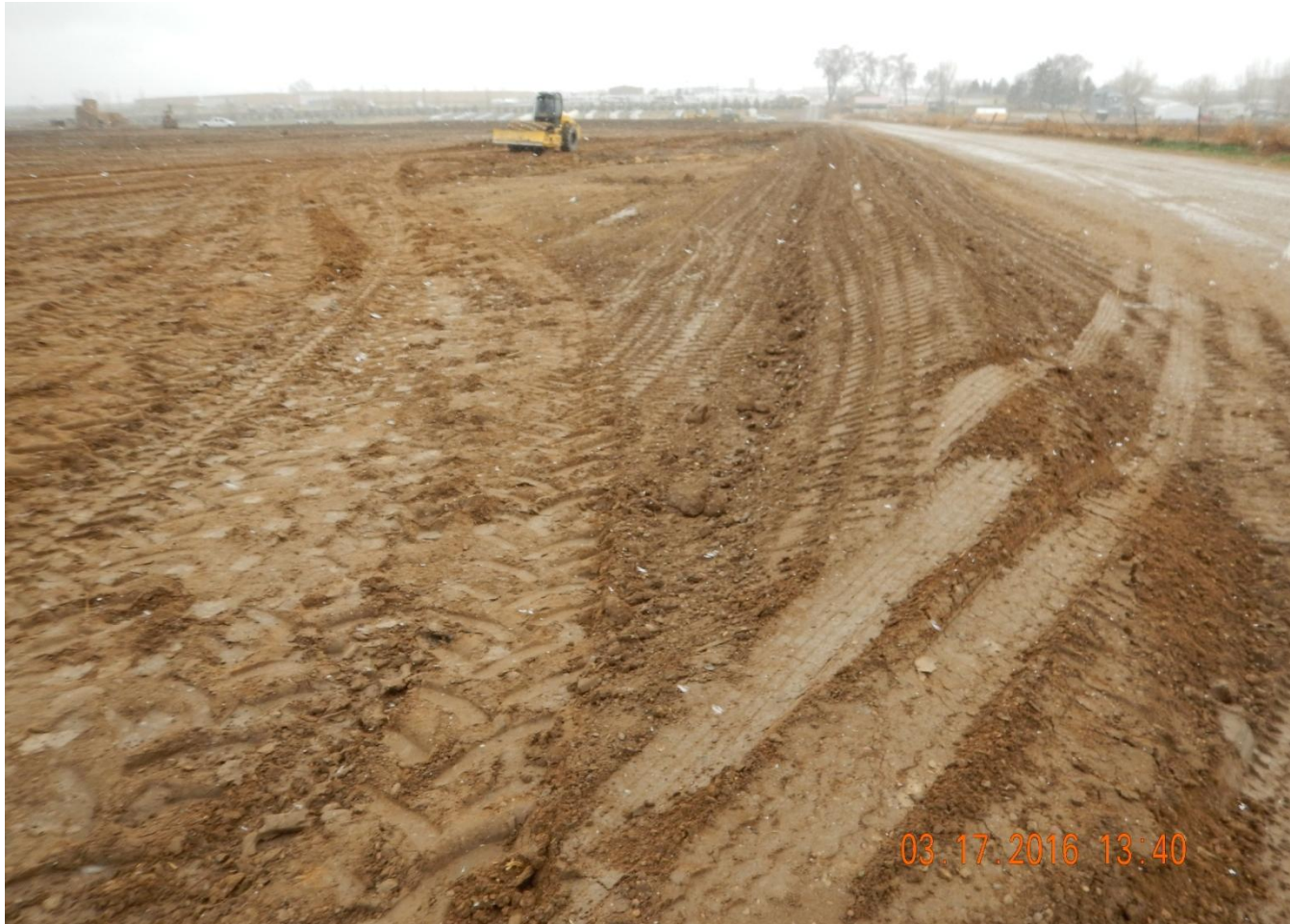
Photo 5. Photo taken from northwest location, facing South. Stormwater and sediment control BMPs installed in center of photo (berm and ditch).
