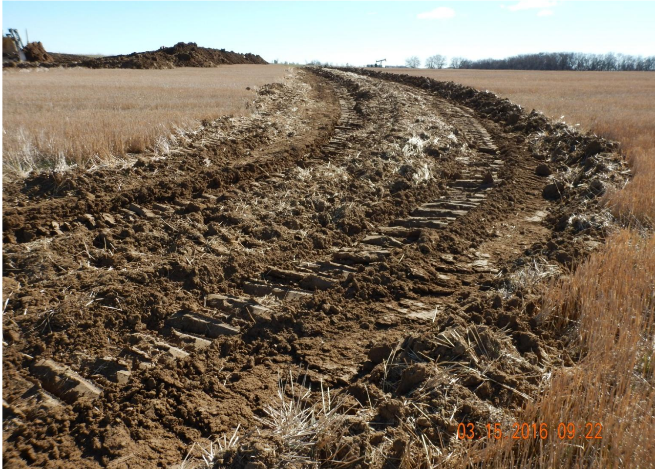
Photo 4. Photo taken from southwest location, facing East. Stormwater and sediment control BMPs installed in center of photo (ditch/berm and surface roughening).
