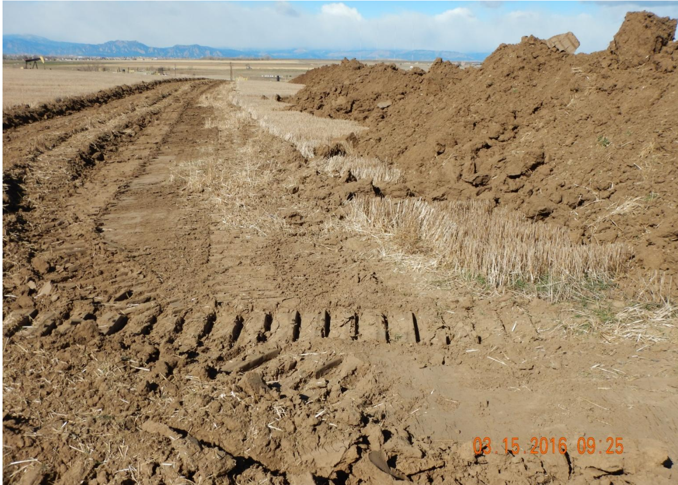
Photo 5. Photo taken from southeast location, facing West. Stormwater and sediment control BMPs installed in center of photo (ditch/berm and surface roughening).
