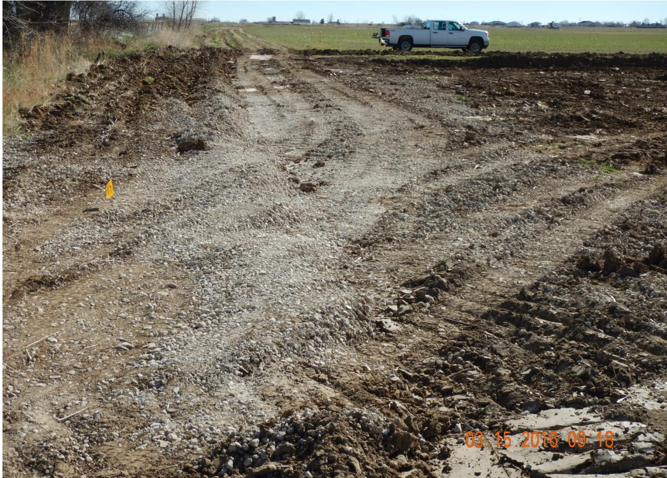
Photo 1. Photo taken from northern location (entrance), facing East. Stormwater and sediment control BMPs installed in center of photo (surface roughening).
