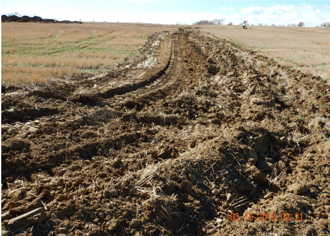
Photo 3. Photo taken from northwest location, facing South. Stormwater and sediment control BMPs installed in center of photo (ditch/berm and surface roughening).
