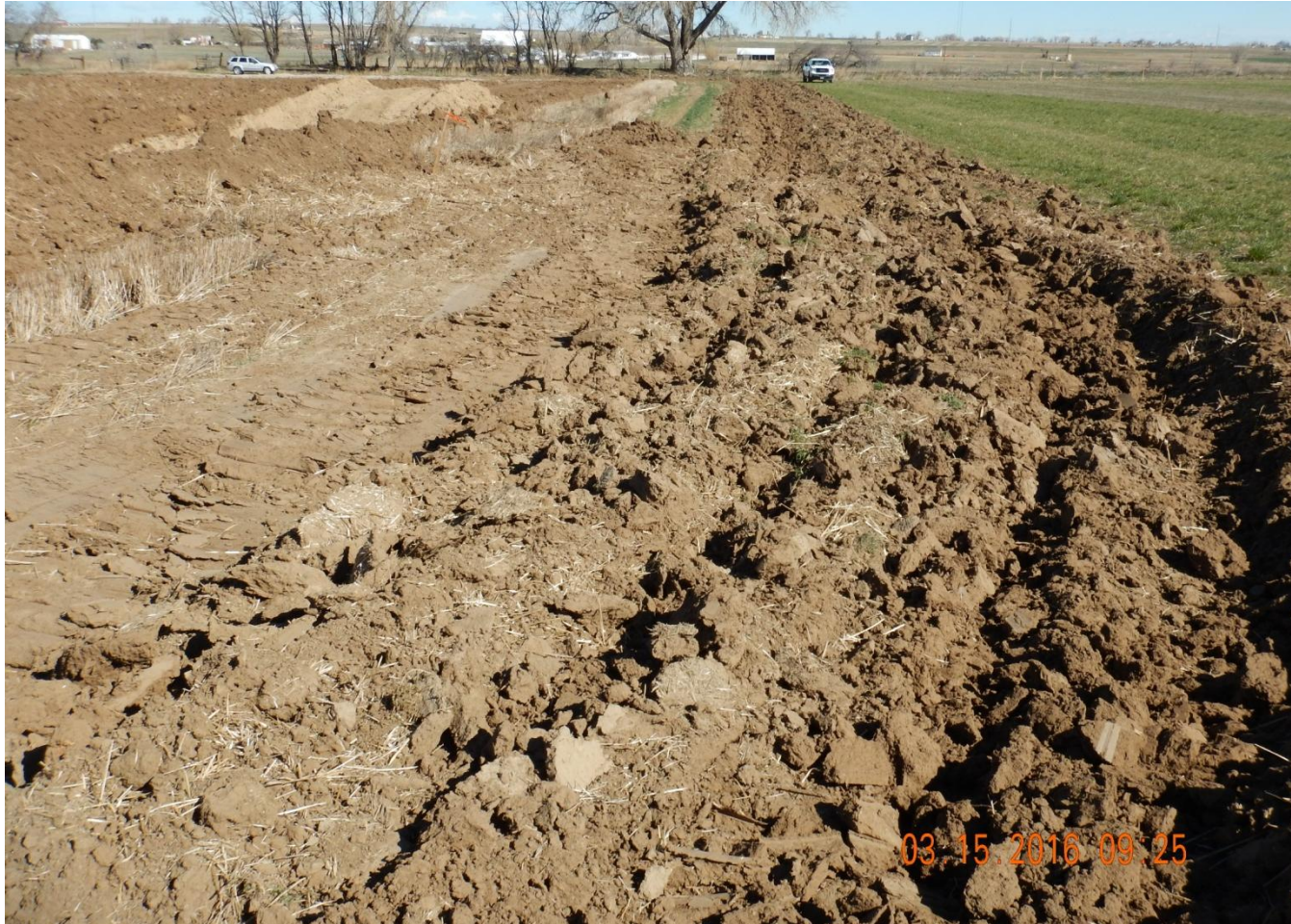
Photo 6. Photo taken from southeast location, facing North. Stormwater and sediment control BMPs installed in center of photo (surface roughening).
