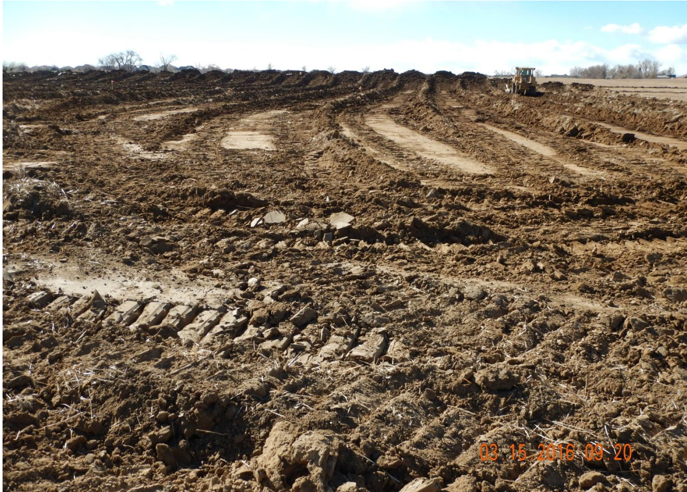
Photo 7. Photo taken from northern location, facing South. Topsoil salvage in process.
