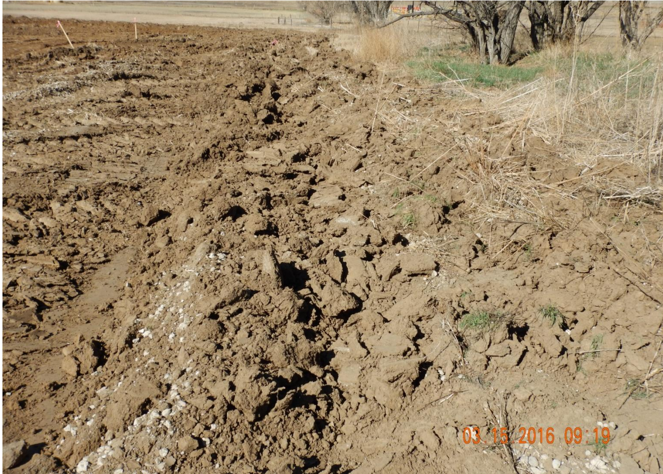
Photo 2. Photo taken from northern location (entrance), facing West. Stormwater and sediment control BMPs installed in center of photo (surface roughening).
