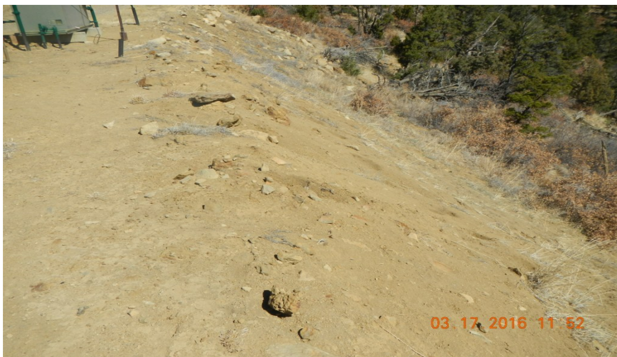
photo 4: East side of the location. The slope is not well stabilized in this area and may need additional BMP's installed.
