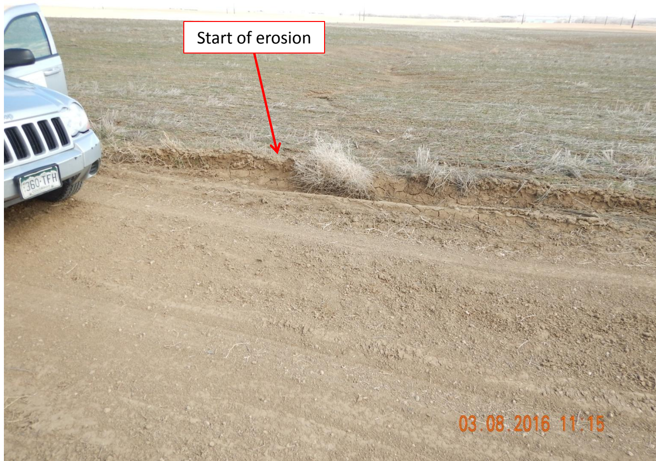
Photo 1. Photo taken from lease road, facing East. Need to control stormwater runoff that minimizes erosion and transport of sediment offsite per Rule 1002. Erosion and transport of sediment is occurring east, offsite, onto cropland.
