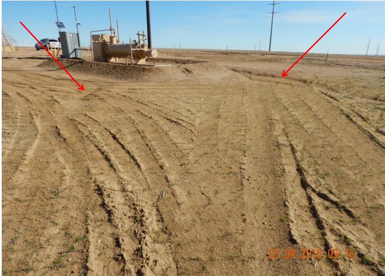
Photo 3. Photo taken from the southern tank battery location, facing Northeast. Need to control stormwater runoff that minimizes erosion and transport of sediment offsite per Rule 1002. Erosion and transport of sediment is occurring south, offsite, onto cropland.
