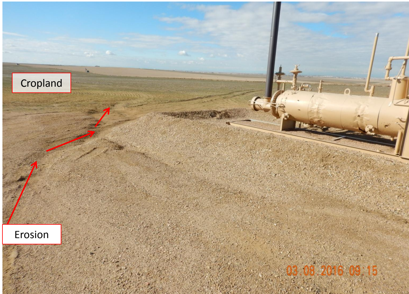
Photo 2. Photo taken from the southern tank battery location, facing Southwest. Need to control stormwater runoff that minimizes erosion and transport of sediment offsite per Rule 1002. Erosion and transport of sediment is occurring south, offsite, onto cropland.
