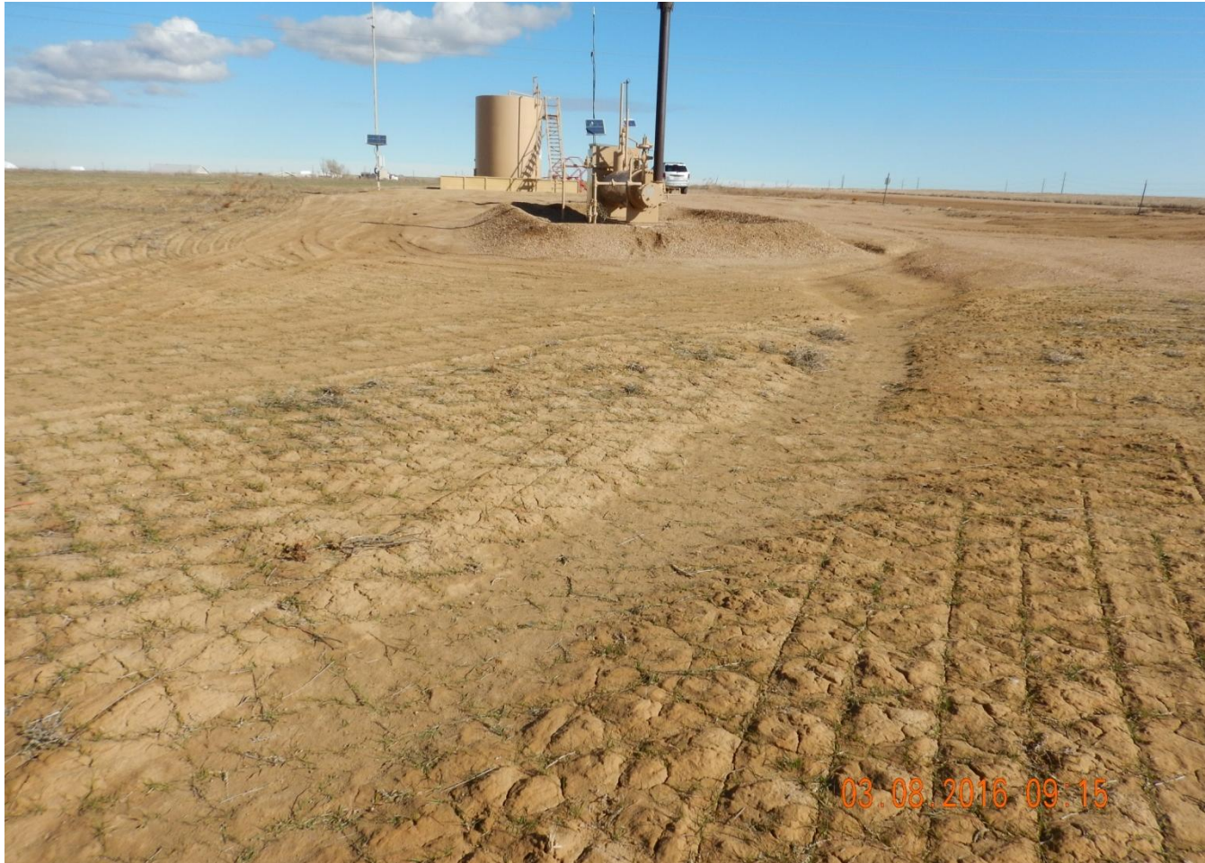
Photo 4. Photo taken from the south of tank battery location, facing North. Need to control stormwater runoff that minimizes erosion and transport of sediment offsite per Rule 1002. Erosion and transport of sediment is occurring south, offsite, onto cropland.
