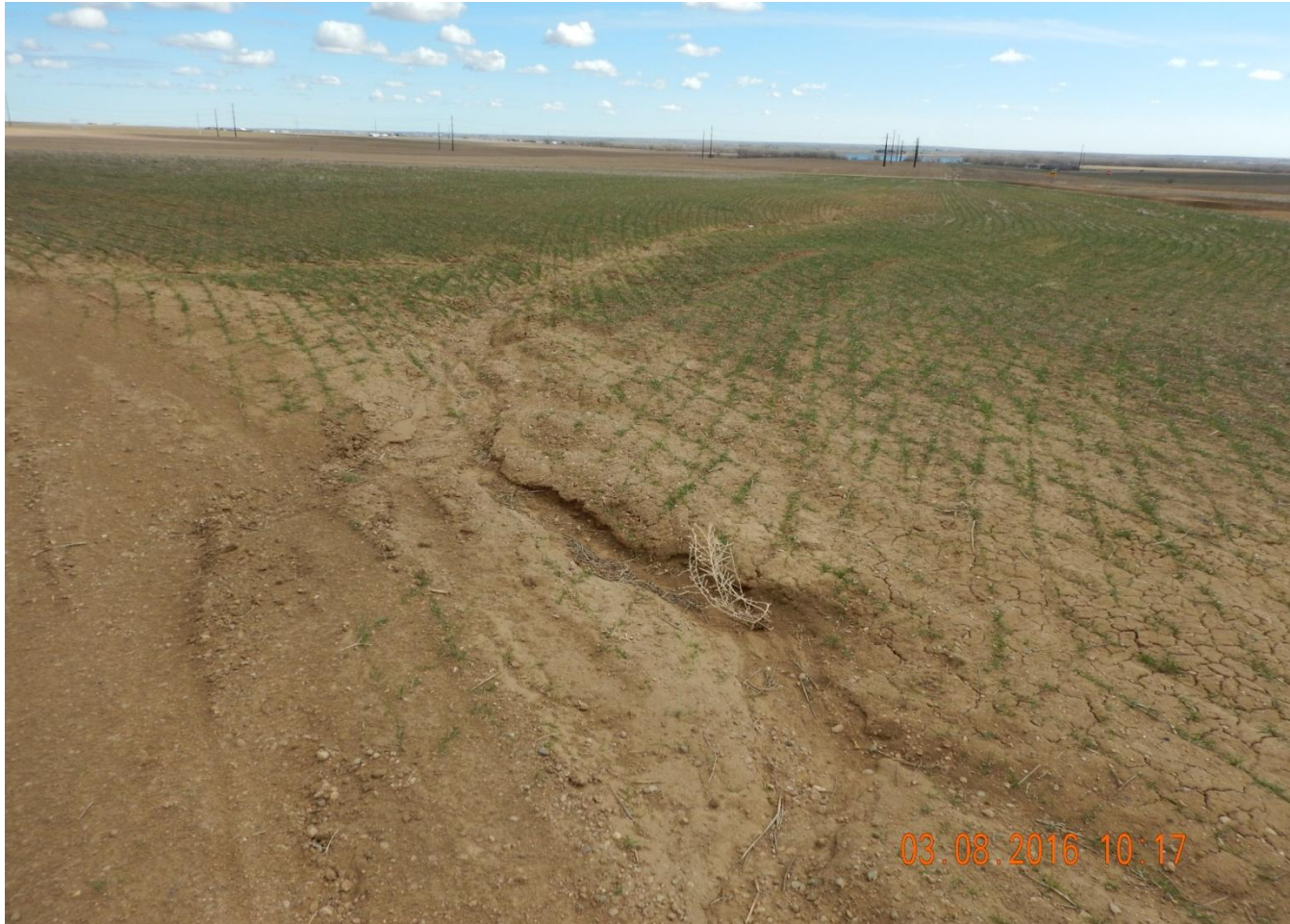
Photo 2. Photo taken from the southeast tank battery location, facing East. Need to control stormwater runoff that minimizes erosion and transport of sediment offsite per Rule 1002. Erosion and transport of sediment is occurring east, offsite, onto cropland. Refer to following photos illustrating erosion and transport of sediment on cropland.
