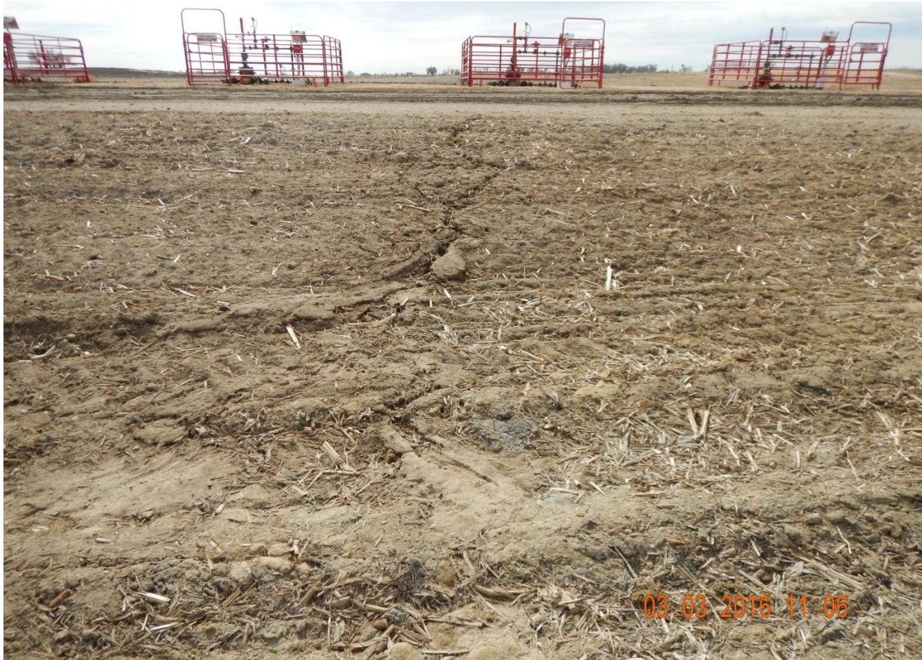
Photo 7. Photo taken from the northern location, facing South. Interim reclamation area needs to be stabilized to minimize erosion while vegetative growth establishes. Erosion is occurring along portions of the eastern and northern interim reclamation area.
