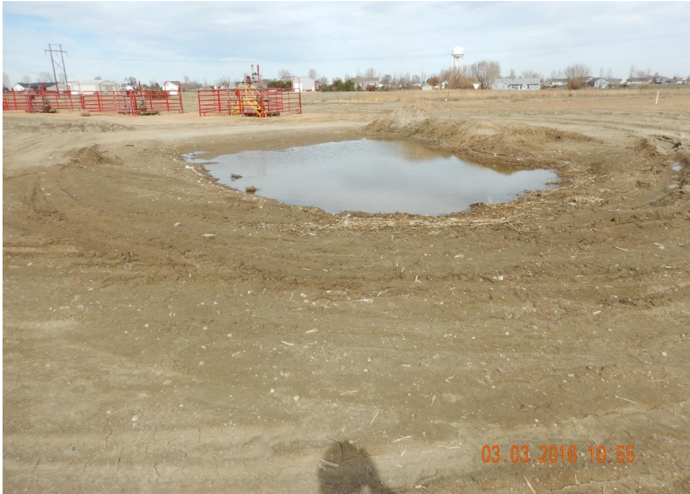
Photo 3. Photo taken from southeast location, facing North. Need to address ponding water. This is only causing additional runoff onto eastern interim reclamation area.
