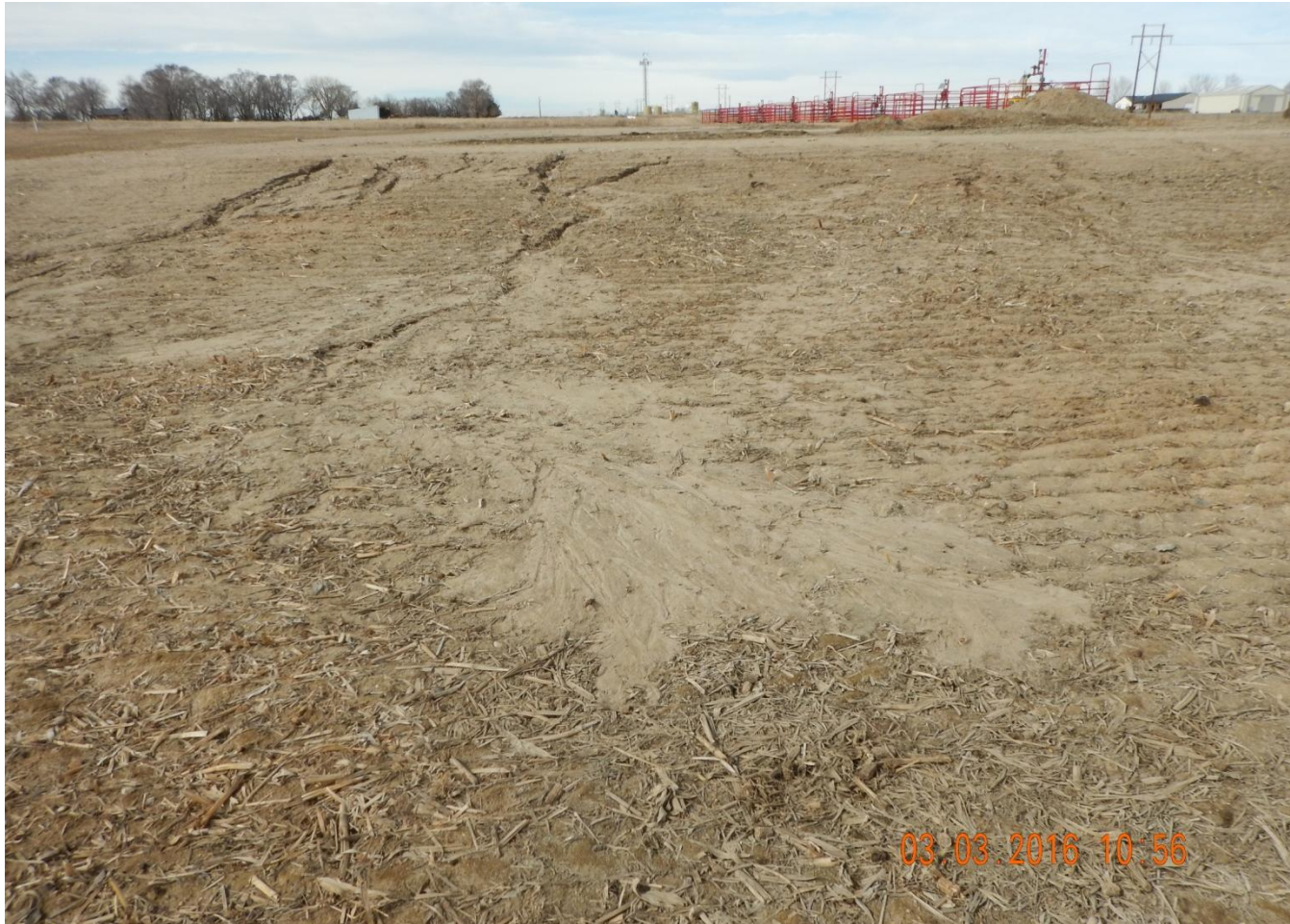
Photo 4. Photo taken from the eastern location, facing West. Interim reclamation area needs to be stabilized to minimize erosion while vegetative growth establishes. Erosion is occurring along portions of the eastern and northern interim reclamation area.
