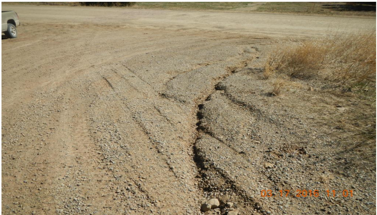
photo 2: An erosion channel has developed which is directing sediment towards the county road.
