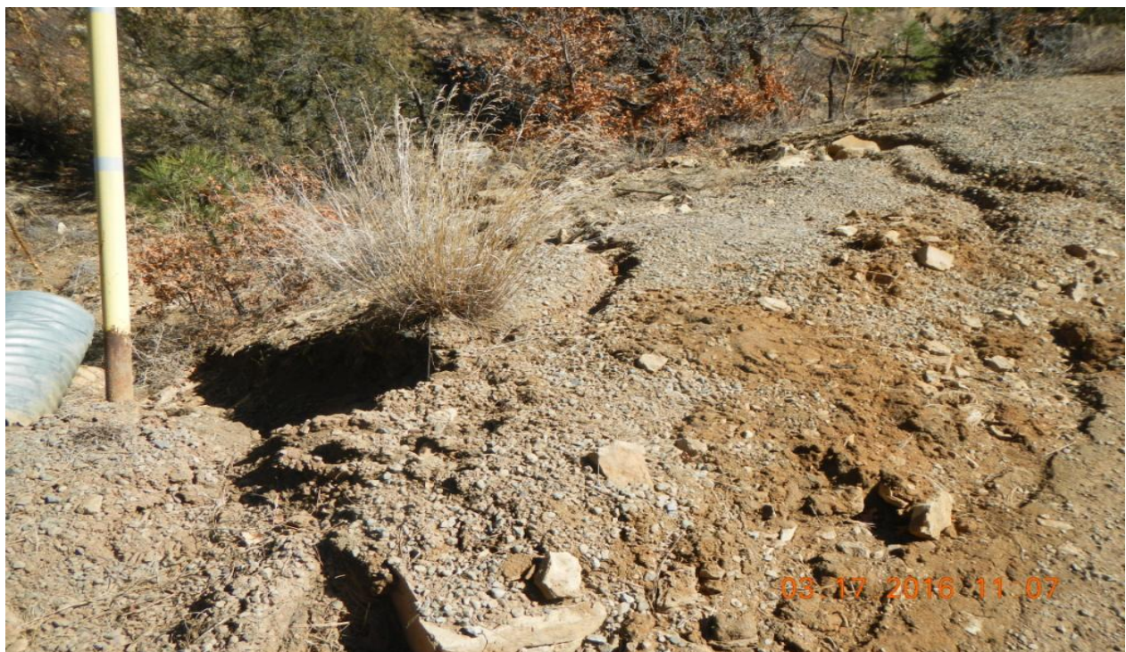
photo 4: Signs of erosion developing off the access road.
