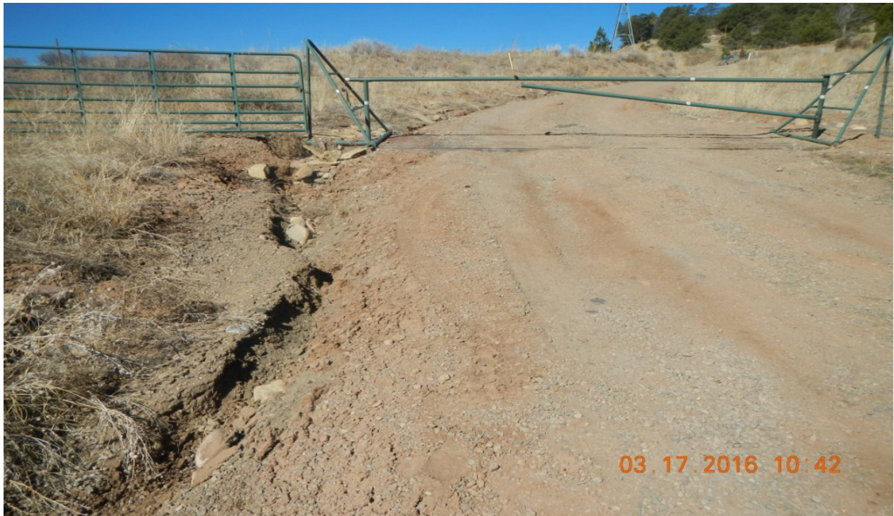
photo 5: Signs of erosion near the gate.
