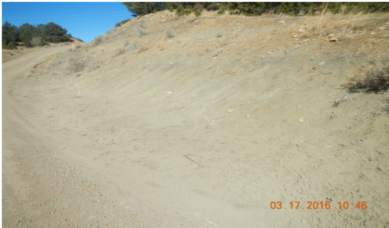
photo 9: Facing toward the northwest cut slope side of the pad, which is not adequately stabilized.
