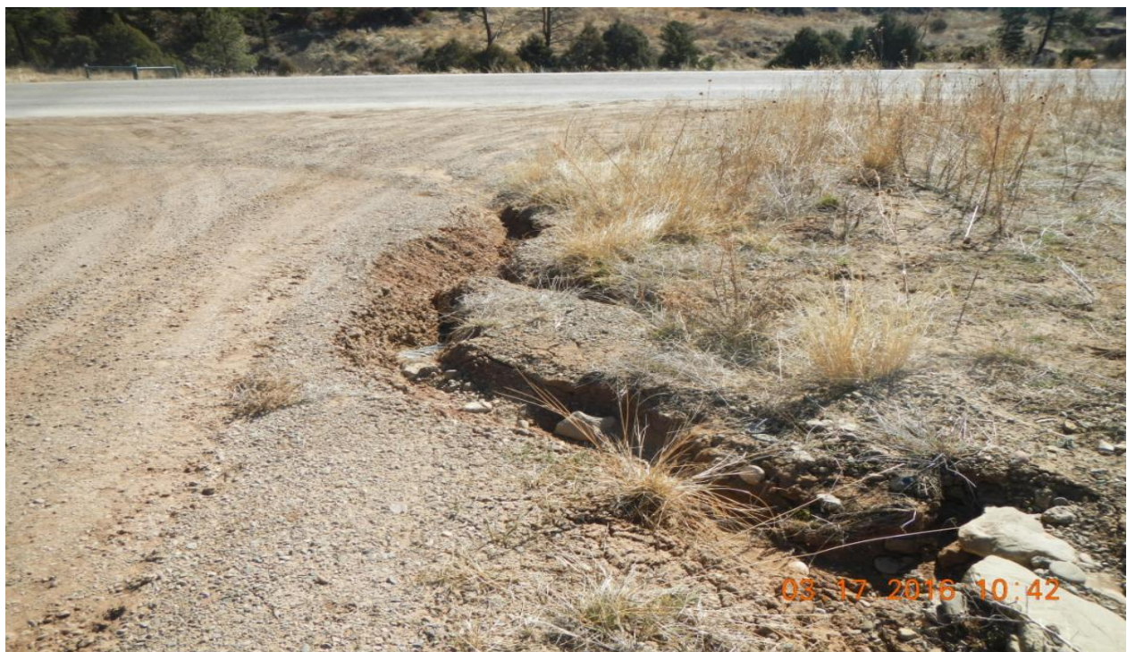
photo 4: An erosion channel has developed which is directing sediment towards the county road.
