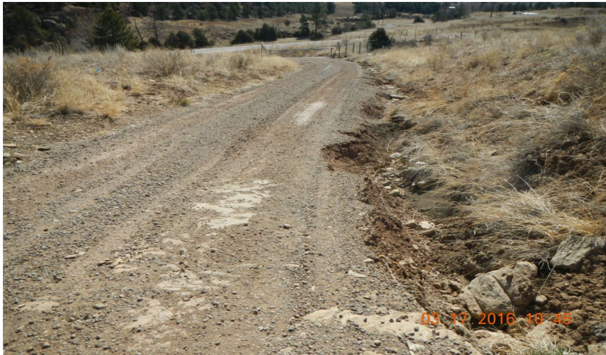
photo 7: Facing back toward the east, there are signs of erosion along the access road.
