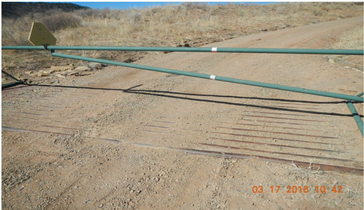
photo 6: Sediment has filled in the cattle guard.
