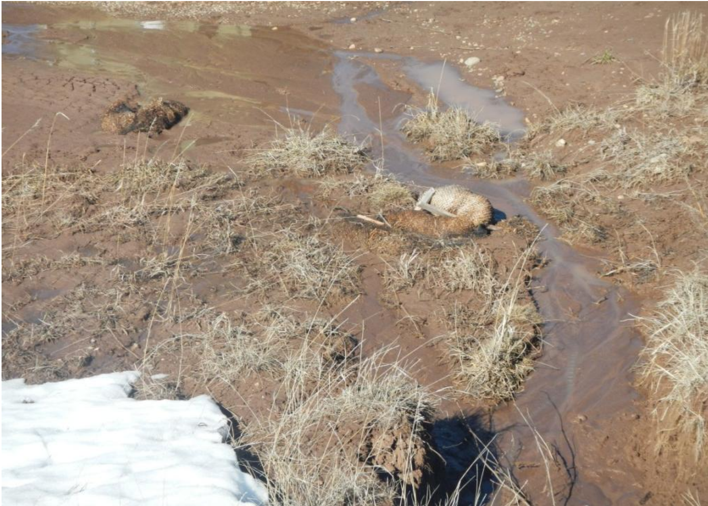
Photo 6. View of straw wattle in the southern portion of the project area that is no longer functioning.
