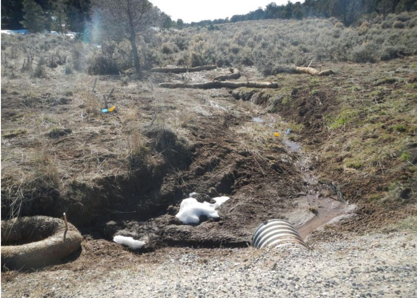
Photo 7. View of wattles at the entrance to the project area facing upstream. Many of these wattles appear to be functioning. Some need maintenance and/or replacement. Wattles may not be sufficiently de-energizing stormwater flows coming off of well pad (on left).
