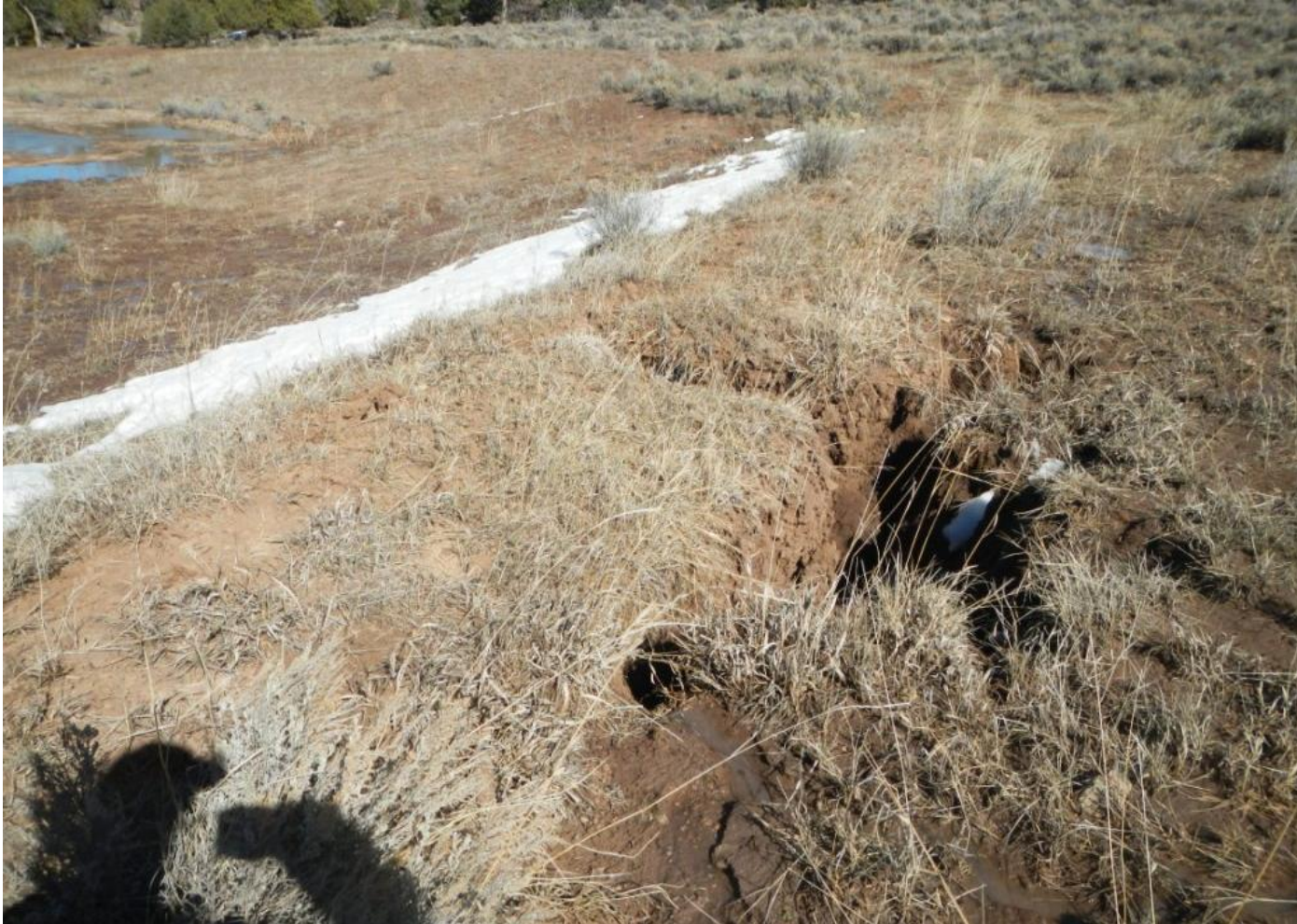
Photo 5. View of head-cut upstream from erosional channels shown in Photo 4. An approximately 6-foot-deep and 3-foot-wide-hole has eroded through the well pad here. This area needs stabilization and repair measures.
