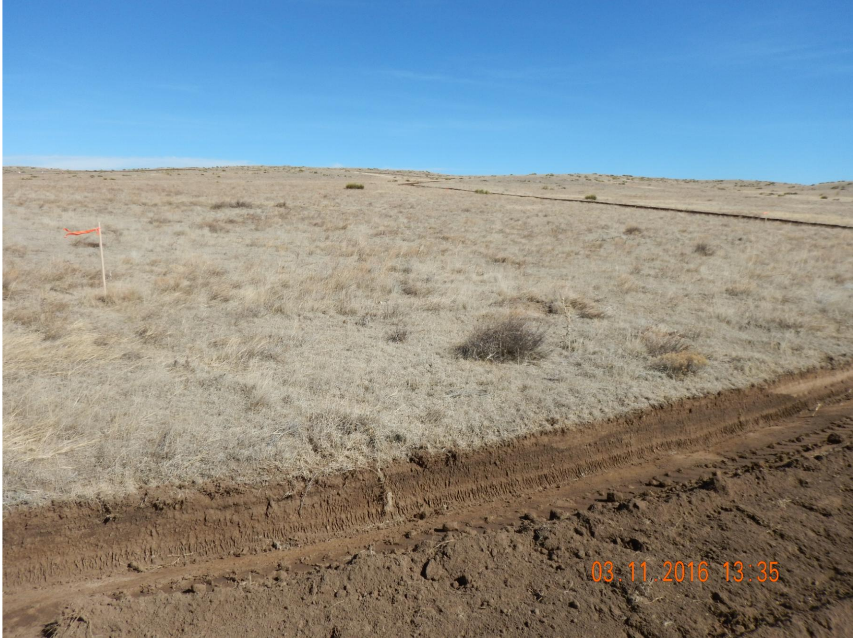
Figure 5: Photo taken from the southwest corner of the location, facing east. Photo shows stormwater control ditch BMP installed on perimeter of location.
