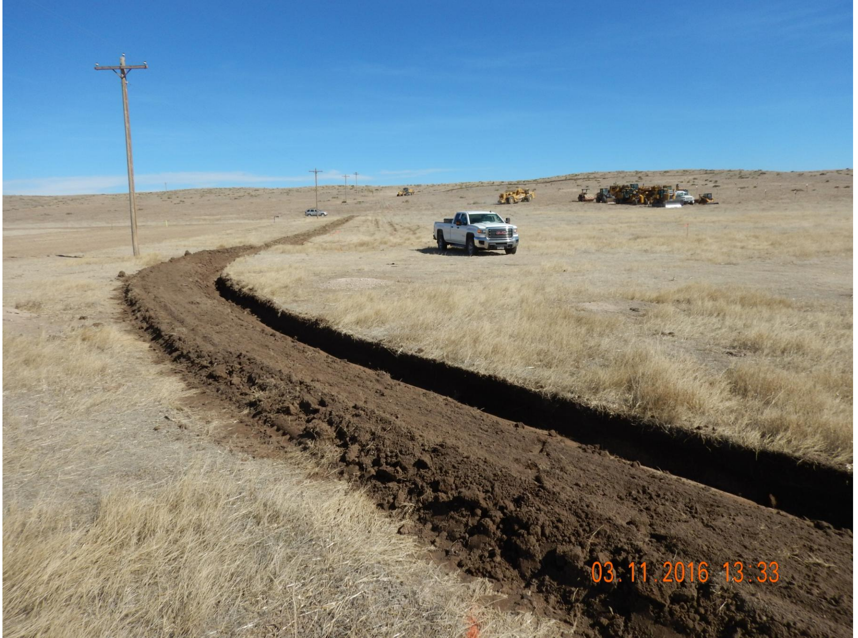
Figure 3: Photo taken from the northwest corner of the location, facing east. Photo shows stormwater control ditch BMP installation in process.
