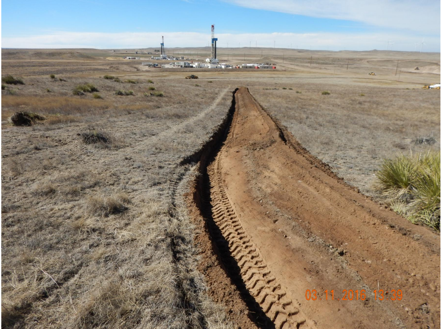
Figure 6: Photo taken from the southeast corner of the location, facing west. Photo shows stormwater control ditch BMP installed on perimeter of location. Note the grade of the slope, velocity checks are advised in areas with steeper grades.
