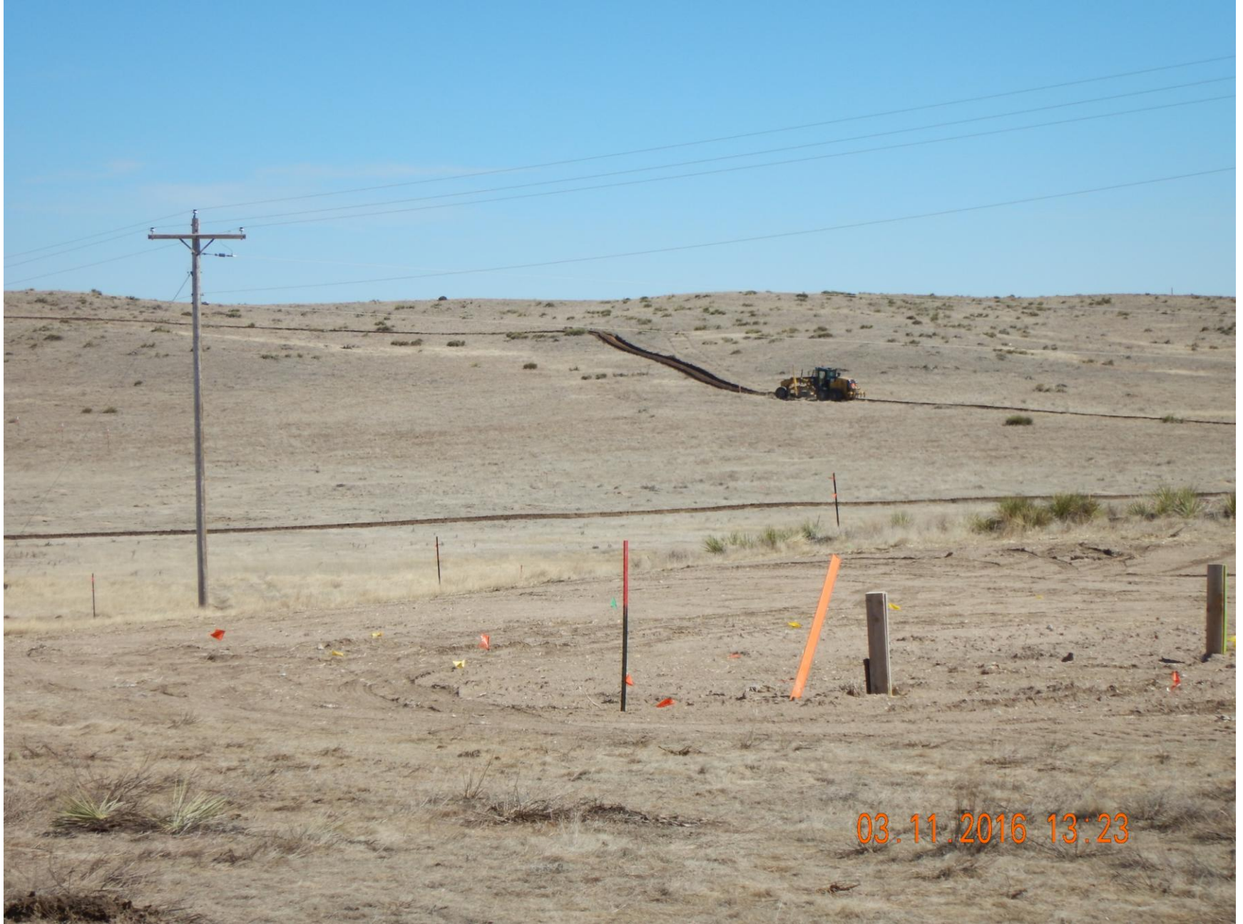
Figure 2: Photo taken from access road, northwest of location, facing southeast. Photo shows stormwater and sediment control ditch construction in process on perimeter of location.
