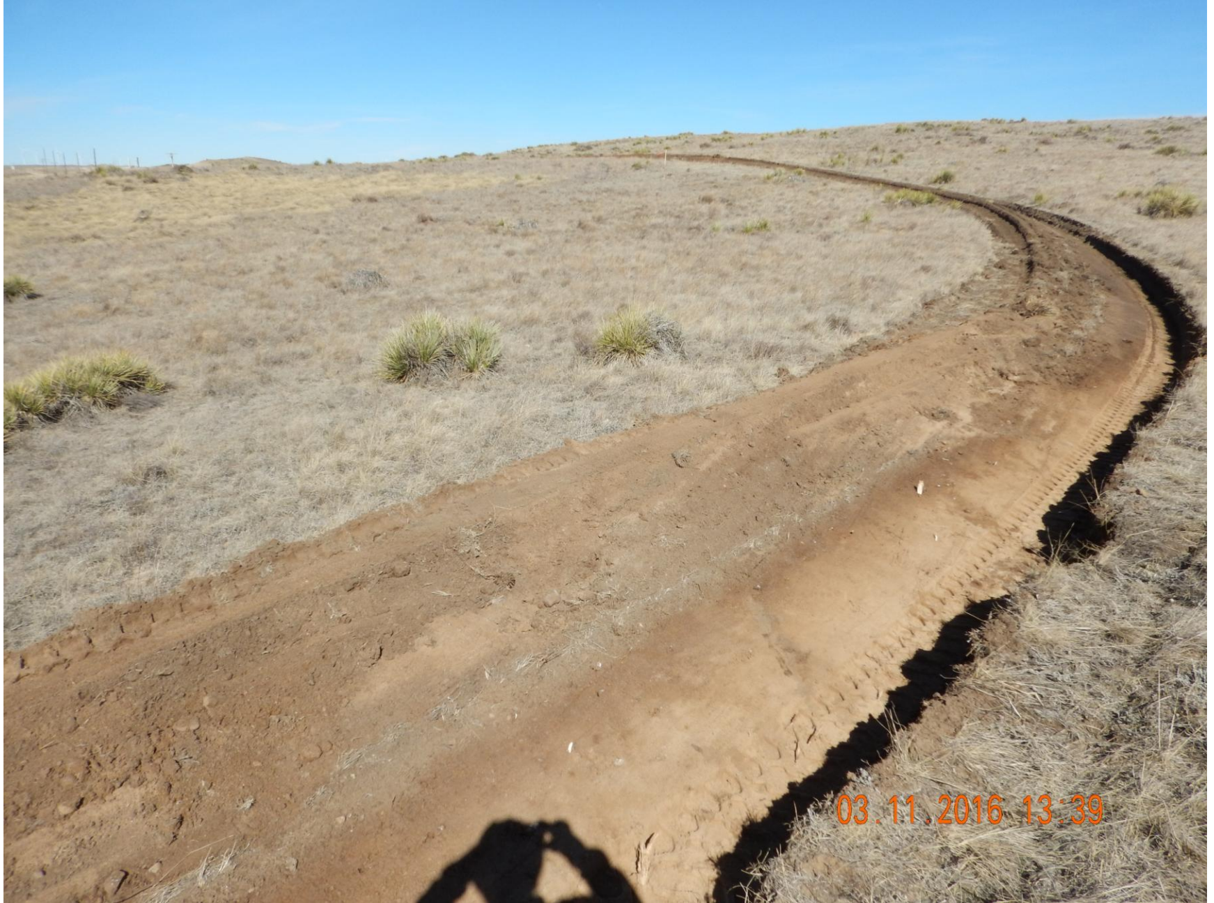
Figure 7: Photo taken from the southeast corner of the location, facing northeast. Photo shows stormwater control ditch BMP installed on perimeter of location. Note the grade of the slope, velocity checks are advised in areas with steeper grades.
