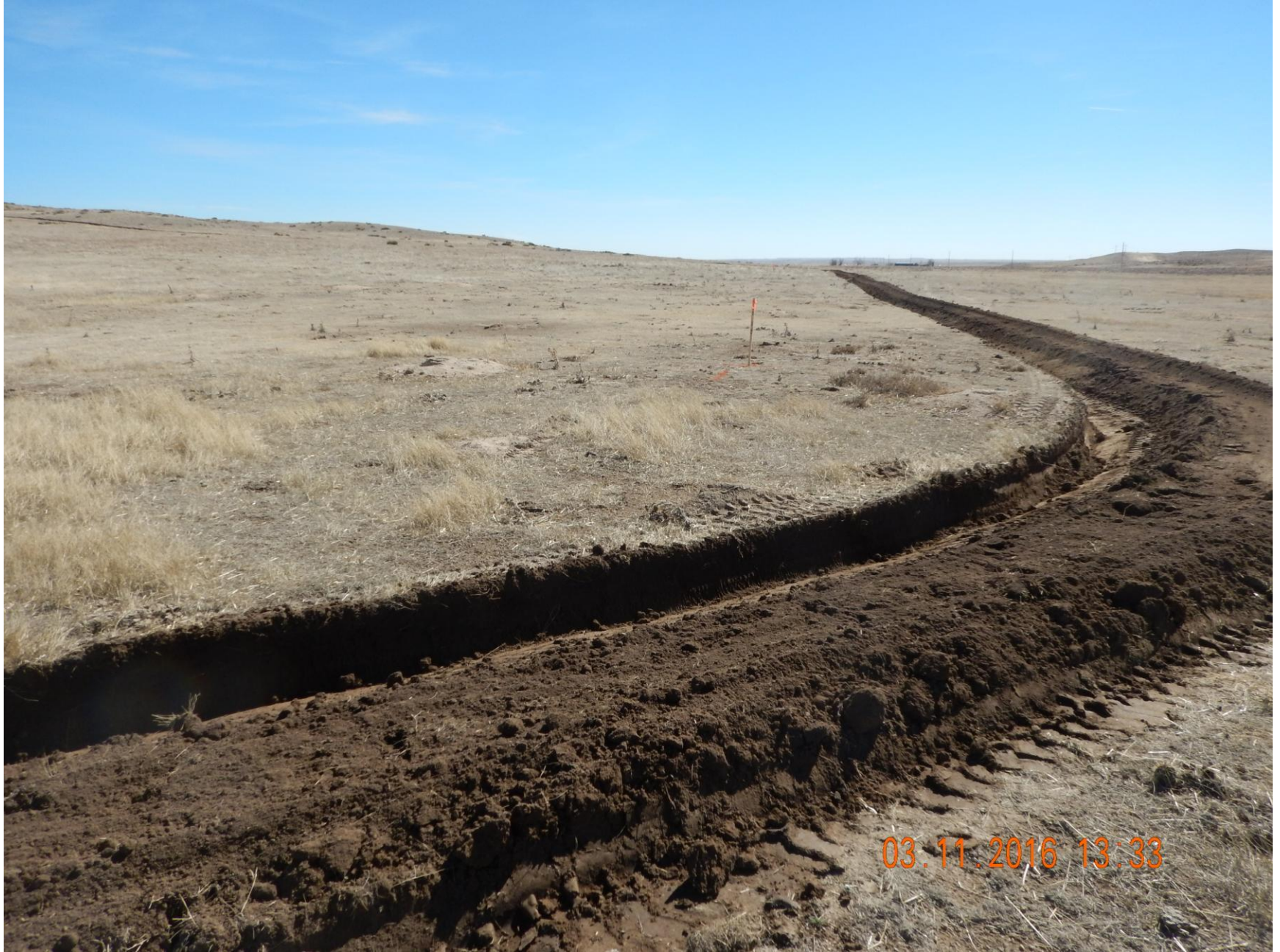
Figure 4: Photo taken from the northwest corner of the location, facing south. Photo shows stormwater control ditch BMP installed on perimeter of location.
