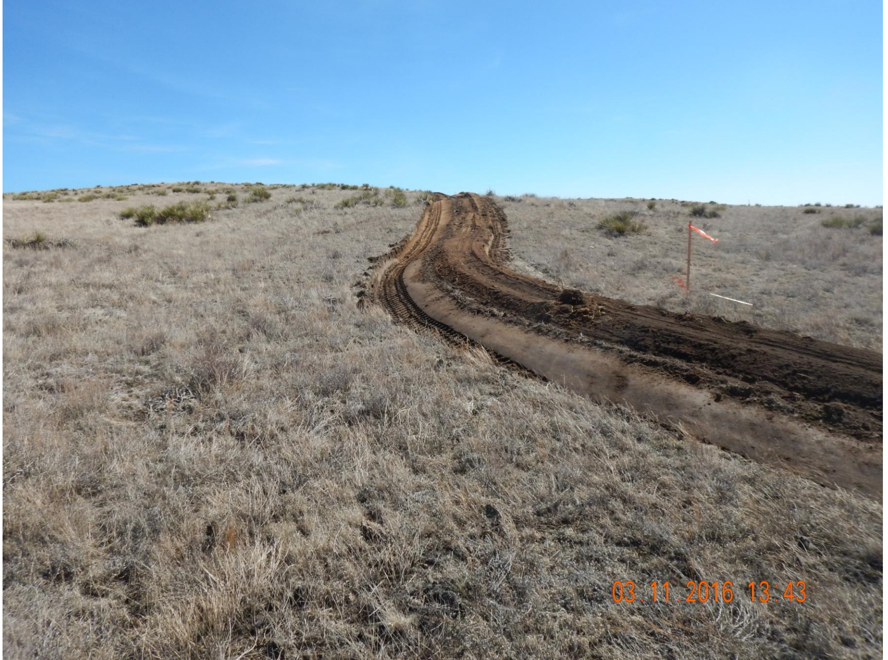
Figure 11: Photo taken from the northeast corner of the location, facing southeast. Photo shows stormwater control ditch BMP installed on perimeter of location. Note the grade of the slope, velocity checks are advised in areas with steeper grades.
