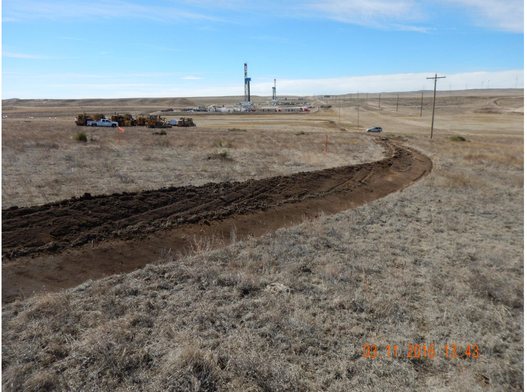
Figure 12: Photo taken from the northeast corner of the location, facing west. Photo shows stormwater control ditch BMP installed on perimeter of location.
