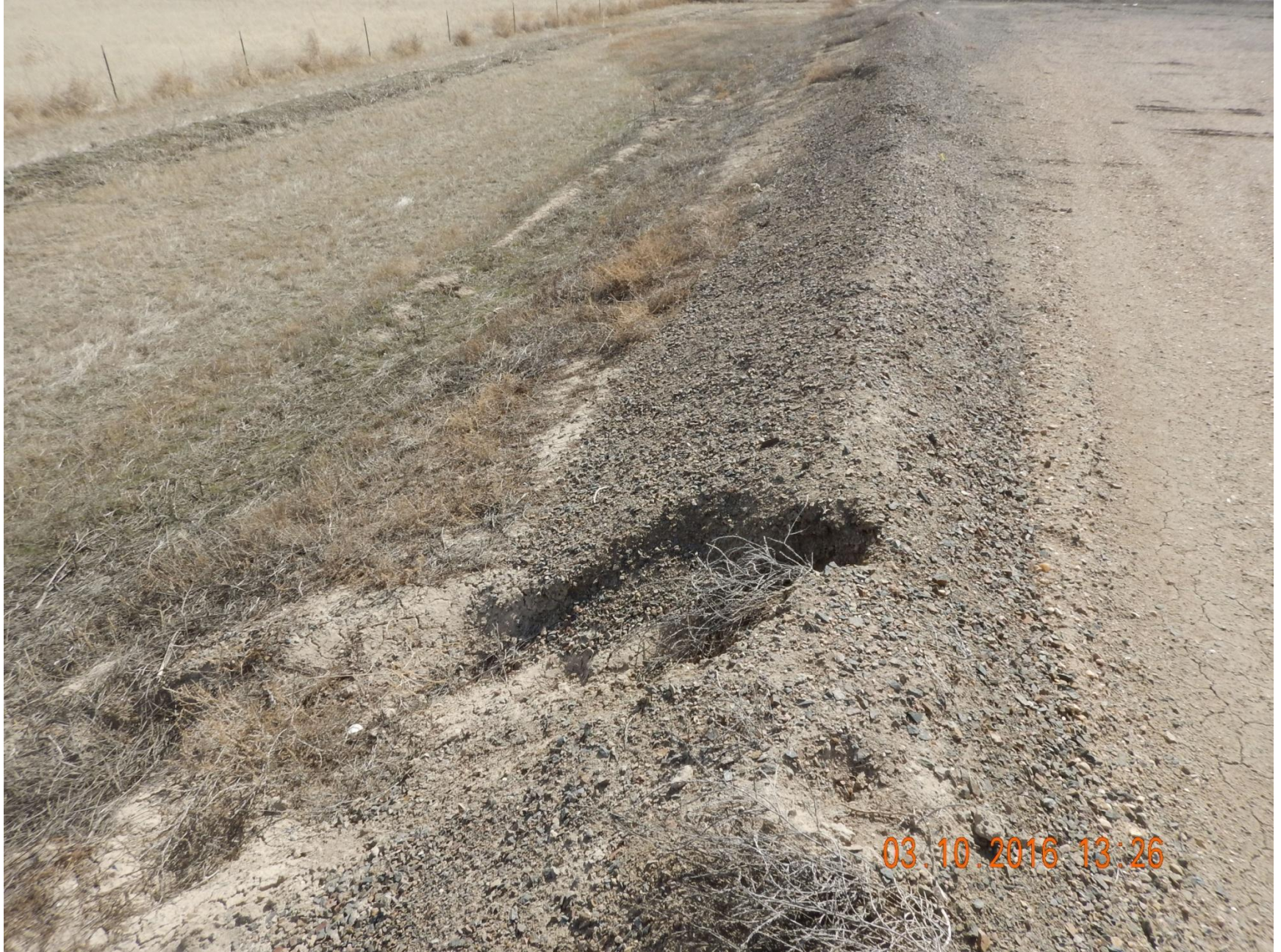
Figure 5: Photo taken from the east end of the location, facing south. Photo shows erosion occurring at perimeter control berm.
