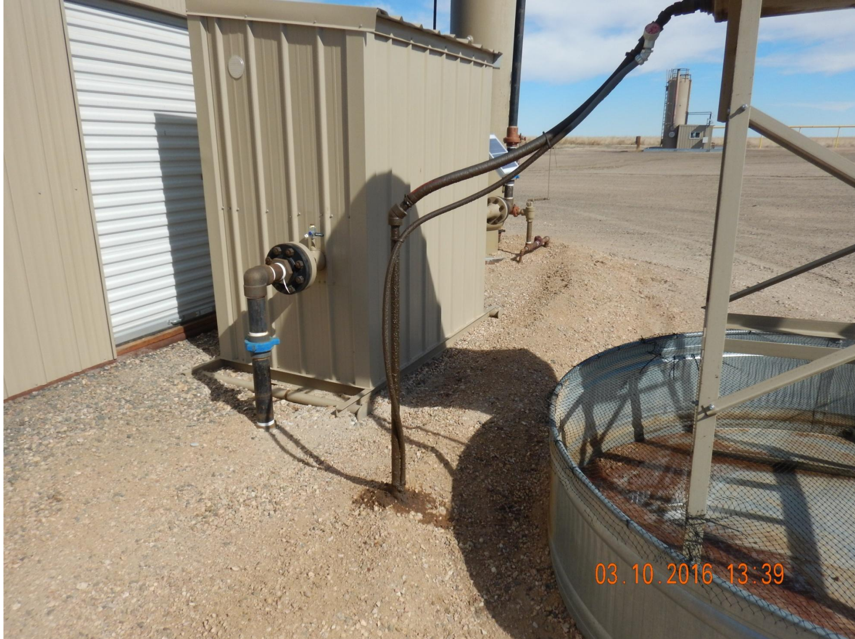
Figure 24: Photo taken from gas lift engine facility on the north end of the location. Photo shows pipe covered in oil, and stained soil.
