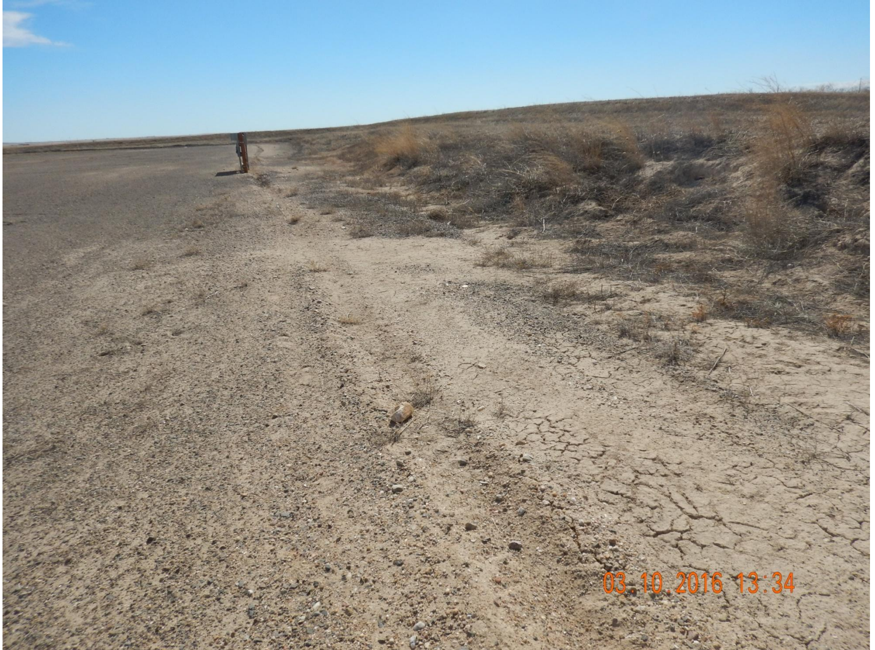
Figure 13: Photo taken from the western end of the project area, facing southwest. Photo shows erosion occurring on location.
