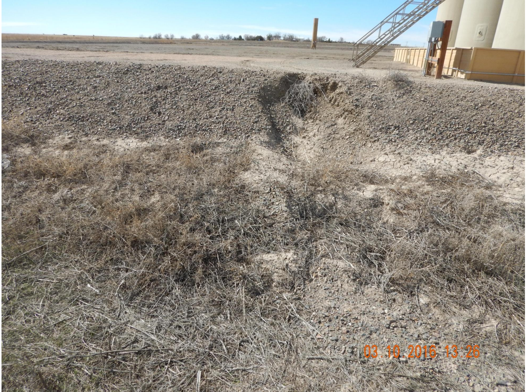
Figure 4: Photo taken from the east end of the location, facing west. Photo shows erosion occurring at perimeter control berm.
