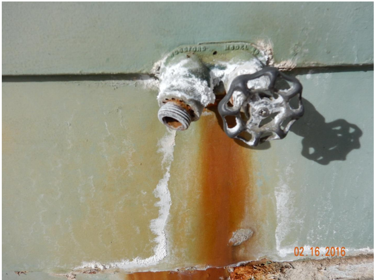
Figure 2 - External spigot located at front porch with aerator, scale-buildup, and rust-staining.
