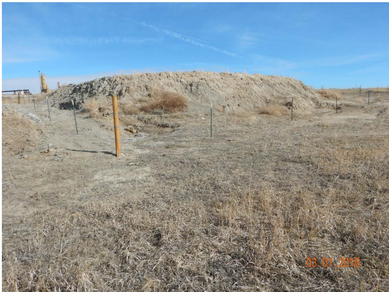
Figure 10 - View of southwest corner of the pit. Note sediment runoff and stressed vegetation outside of fenced-in area at southeast and southwest corners.
