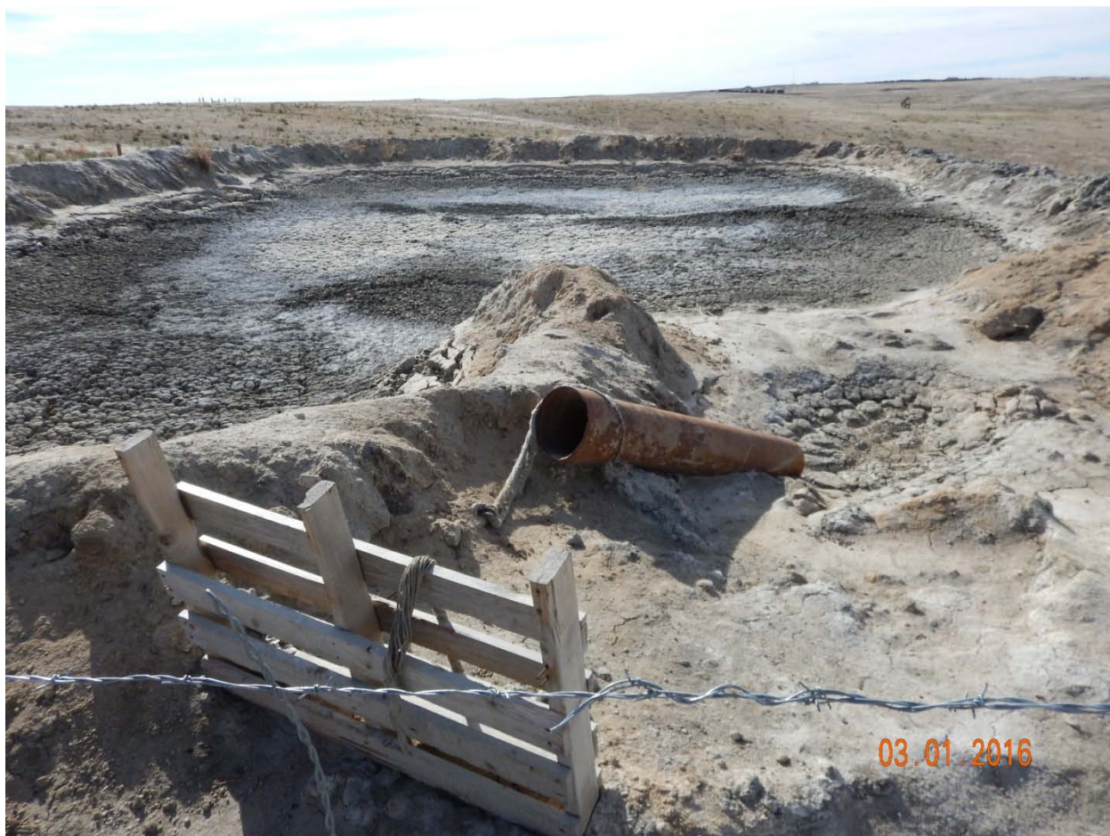
Figure 8 - View of unpermitted pit from the north, pit measured approximately 50'x50' and contained E&P waste. Southeast corner located at 39.577958 N, 104.568864 W.
