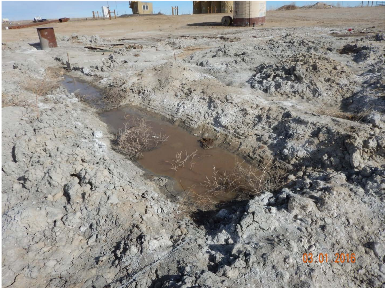
Figure 13 - View of ditch leading from abandoned wellhead to pit. Note presence of water and vegetation.
