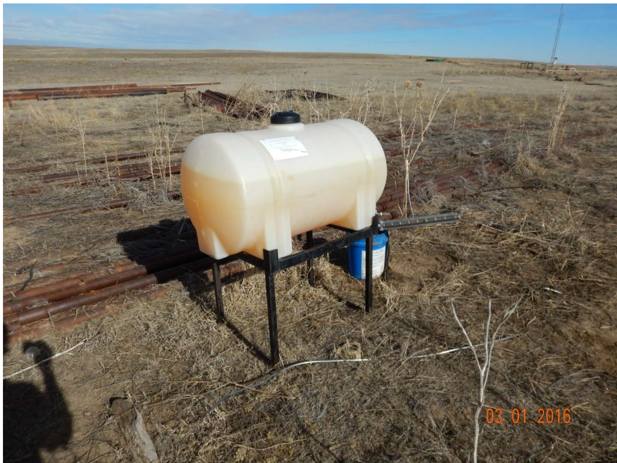
Figure 3 - Chemicals stored on-location lacking secondary containment.
