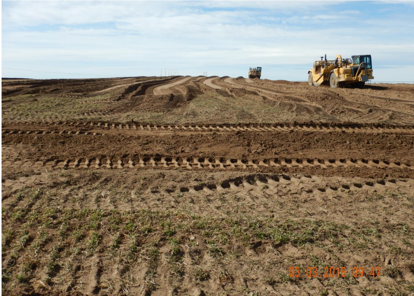
Photo 10. Photo taken from eastern location, facing West. Topsoil salvage in process.
