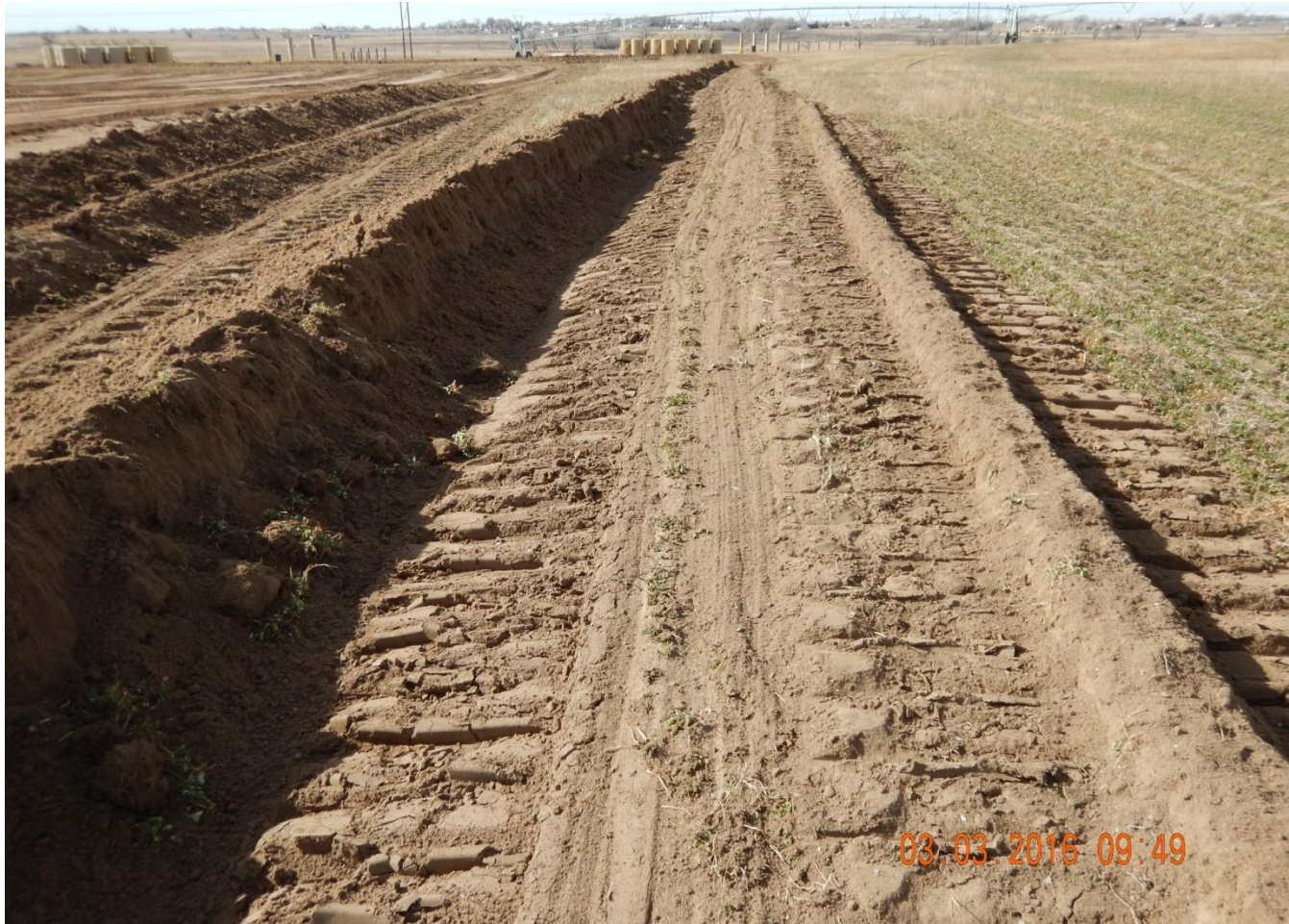
Photo 4. Photo taken from northwest location, facing South. Stormwater and sediment control BMPs installed in center of photo.
