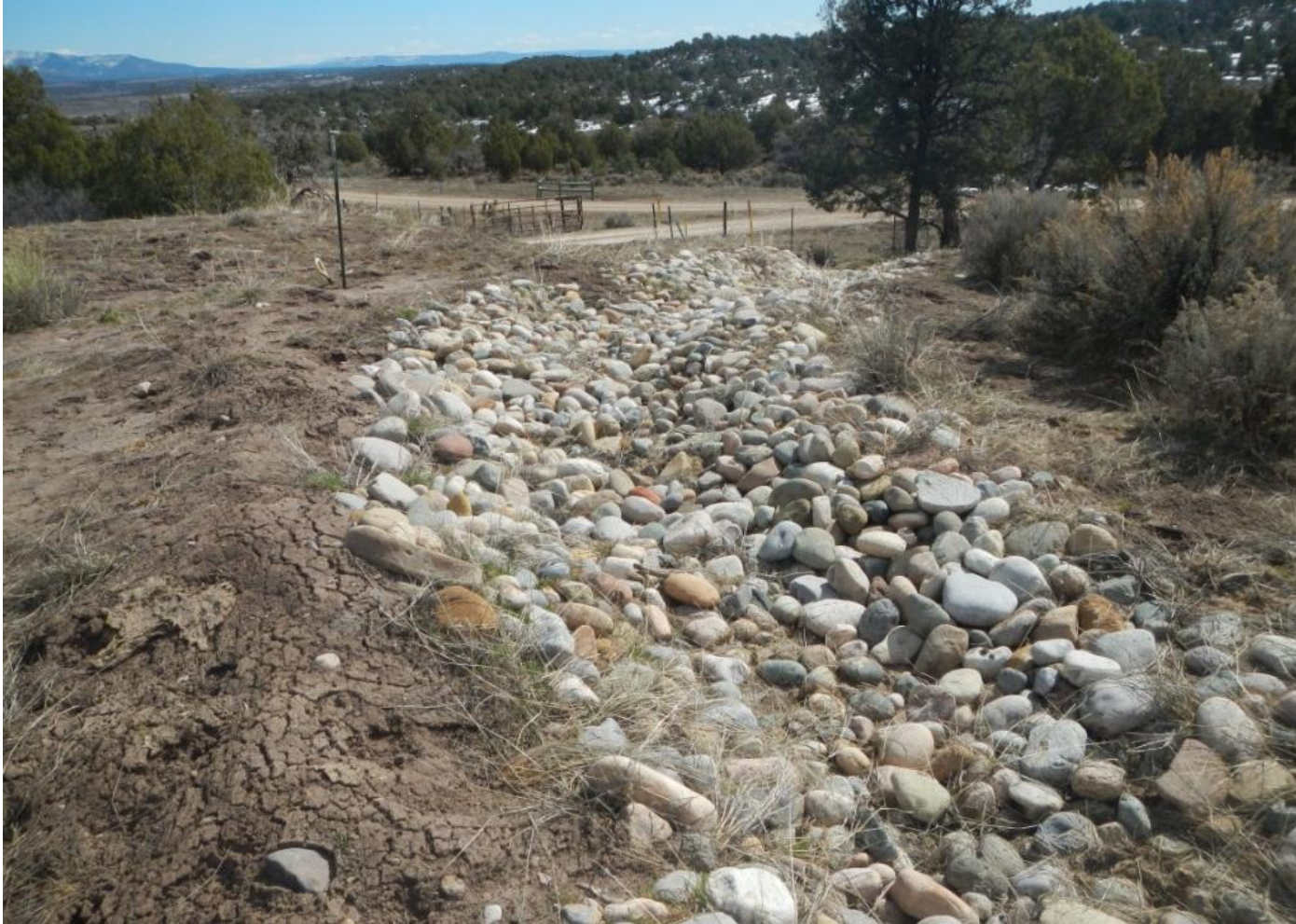
Photo 5. View of cobble BMP in the southern portion of the project area that appears to be functioning.
