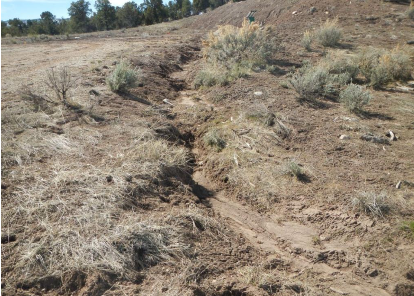
Photo 3. View of erosion occurring where stormwater flows off of the northeastern edge of the project area where it flows onto the adjacent well pad and then forms a gully (Photo 4).
