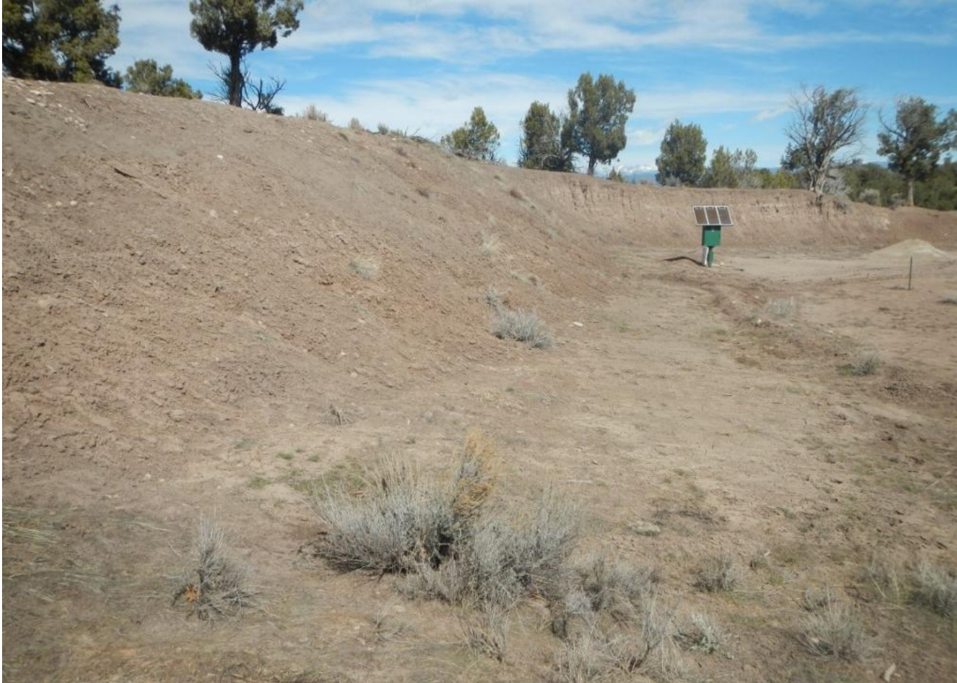
Photo 6. View of the western portion of the project area from the southwestern corner facing northward. Revegetation does not appear to be progressing on the slopes and revegetation may be needed.
