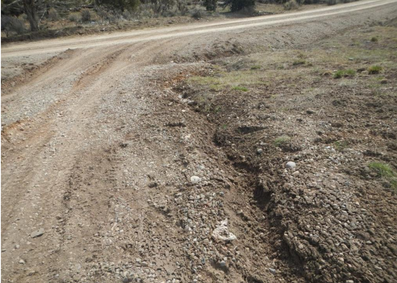
Photo 1. View of erosion occurring along the access road to the well pad. Erosional channel is approximately 18 inches wide and 15 inches deep.
