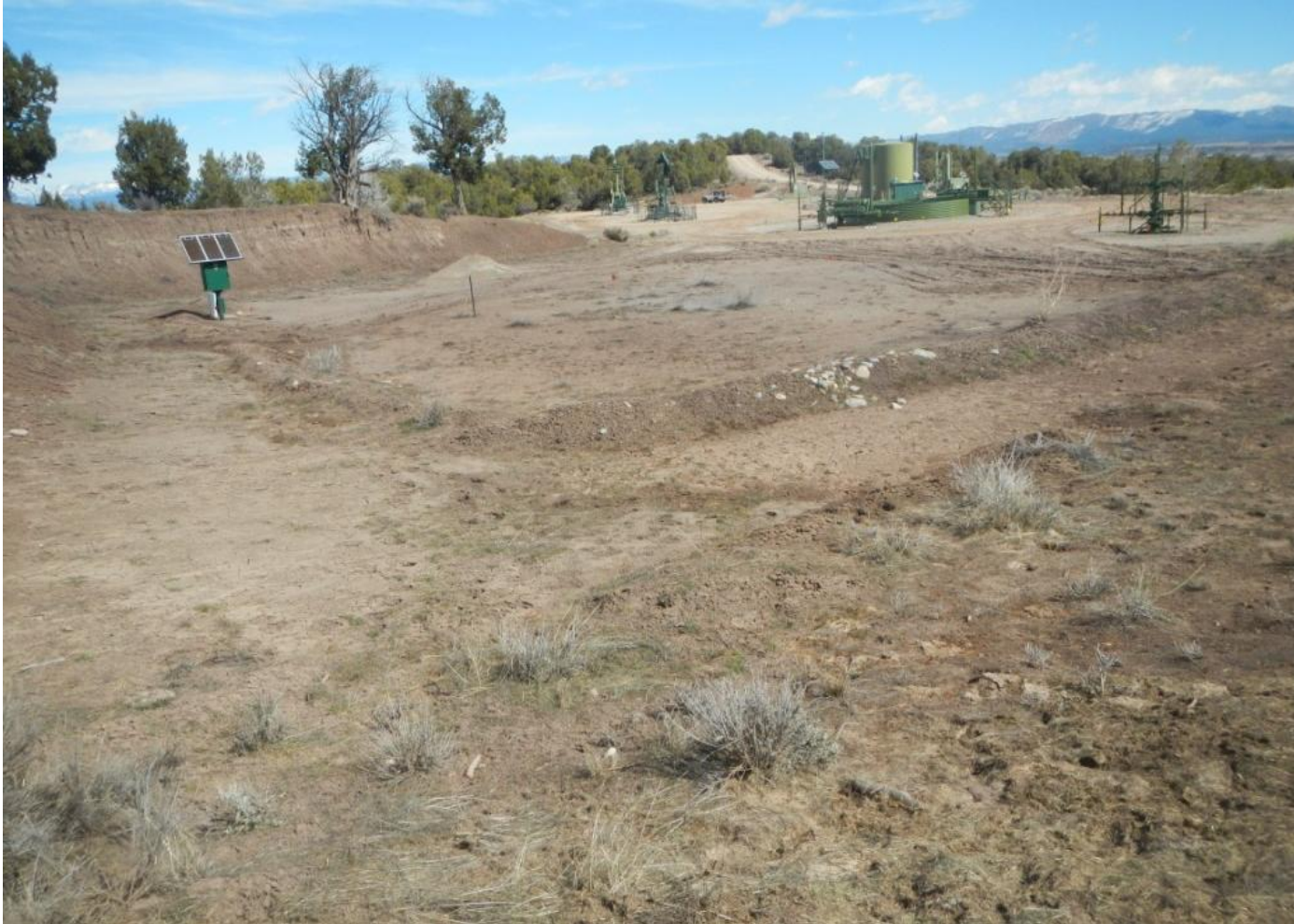
Photo 7. View of project area from the southeastern corner facing center. Poor revegetation in the western portion on flat areas that do not appear necessary for production operations. These areas should be revegetated in fall 2016 if vegetative cover does not increase during the growing season.
