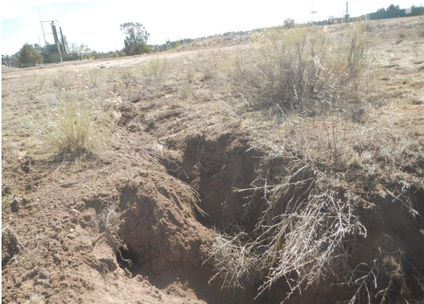
Photo 4. View of gully forming in northern edge of the adjacent well pad.
