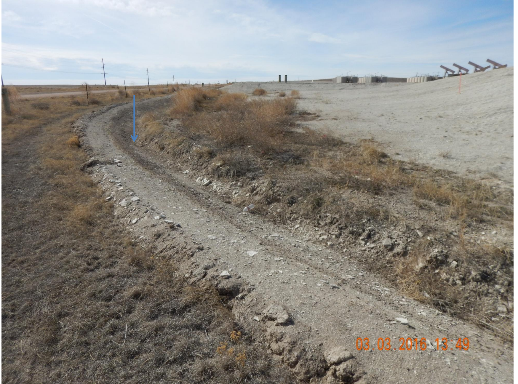
Figure 14: Photo taken from the southeast corner of the interim area facing west. Photo shows stormwater diversion ditch.
