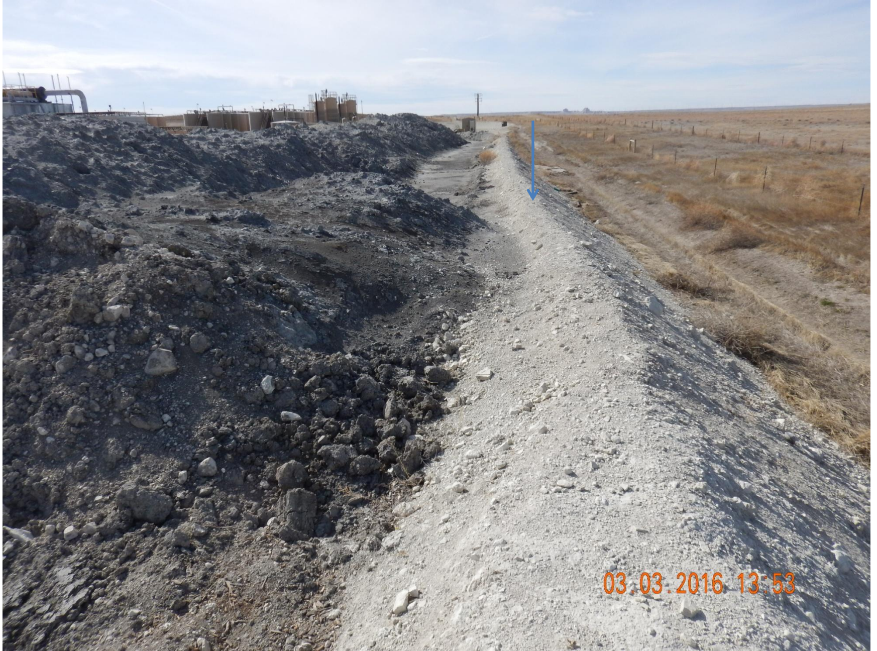
Figure 20: Photo taken from the northeast corner of the project area, facing west. Photo shows containment berm on the northern perimeter of the location, and the drill cuttings.
