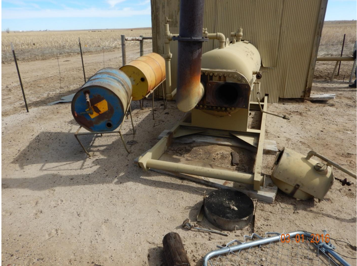
Figure 15 - Partially-dismantled separator with unused equipment and storage drums lacking secondary containment at separator shed.
