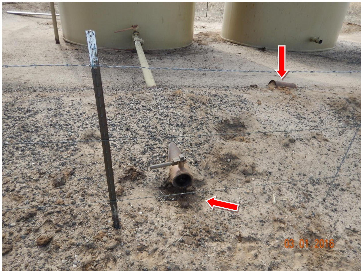
Figure 4 - Oil-stained soil at tank loadout and inside of containment berm, note unused equipment/trash present behind berm.
