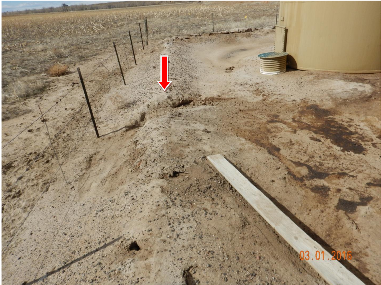
Figure 5 - Oil stained soil inside of tank battery and gap in berm.
