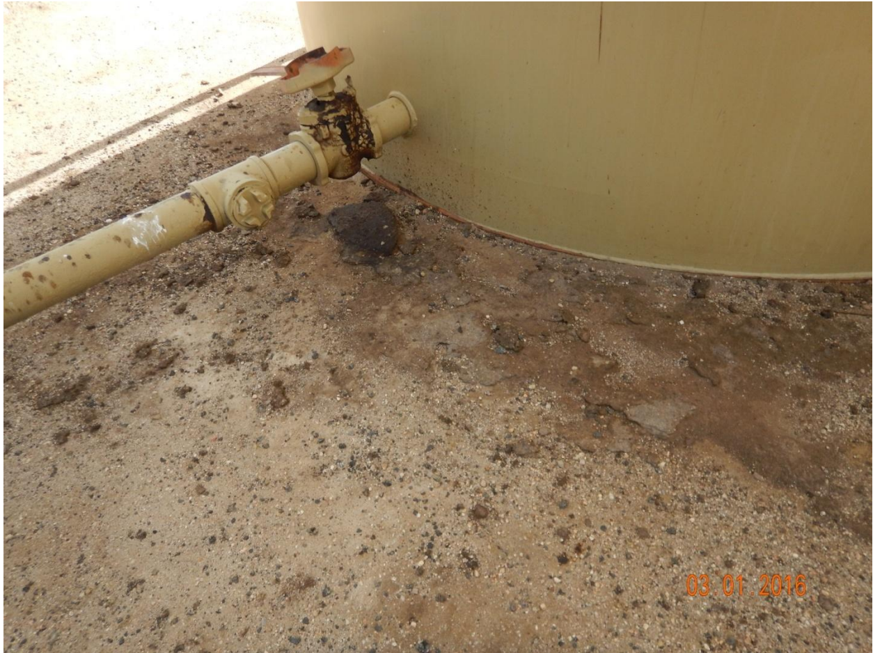
Figure 11 - Oil-stained soil beneath leaking valve on crude oil AST.
