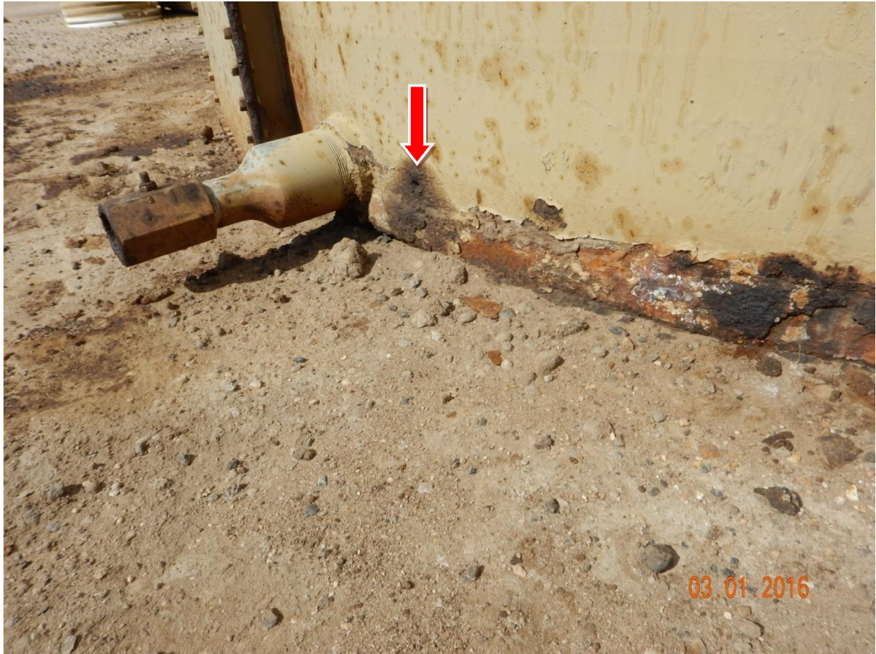
Figure 7 - Oil-stained soil, corrosion, and small hole in crude oil AST.
