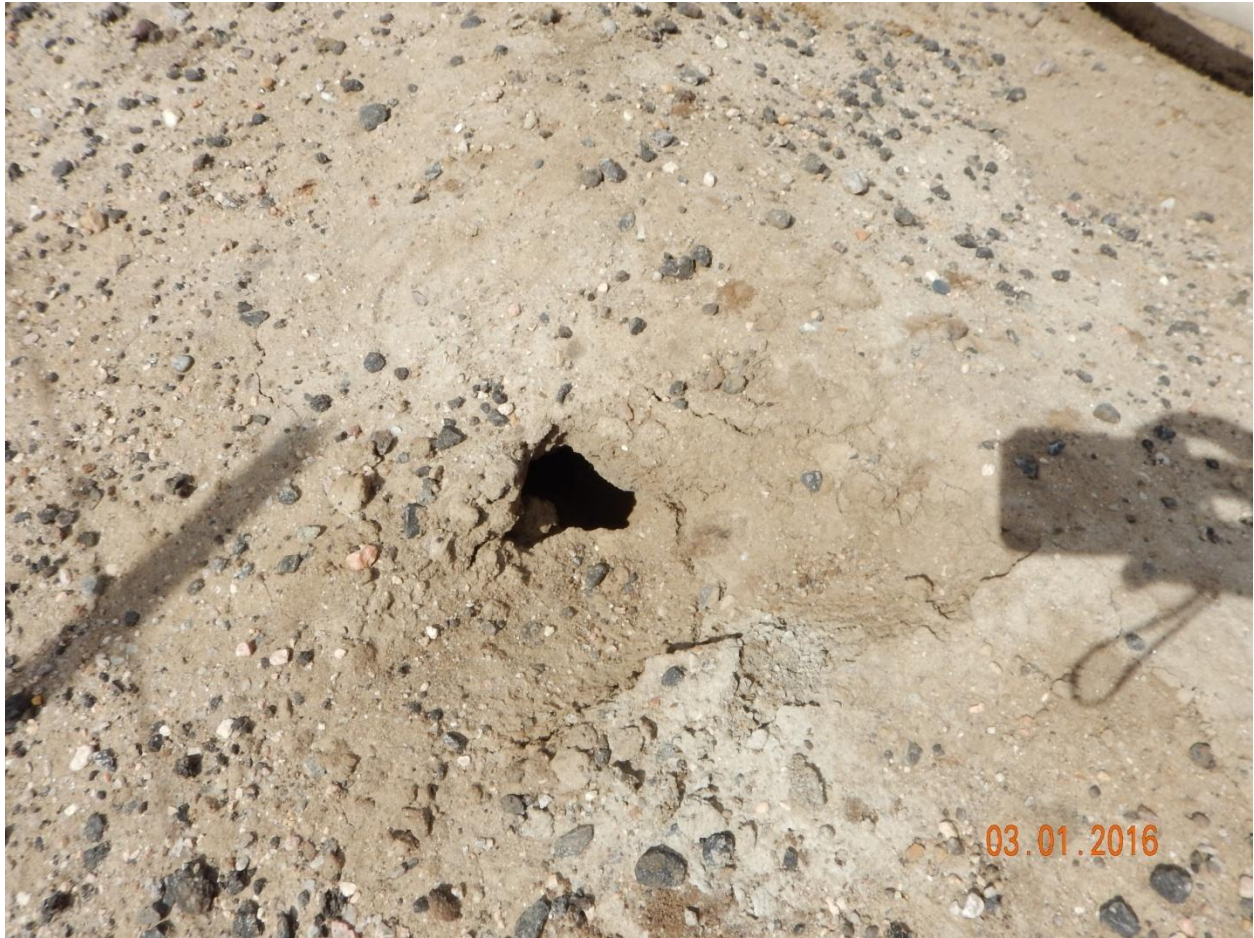
Figure 9 - Burrow observed in tank battery berm.
