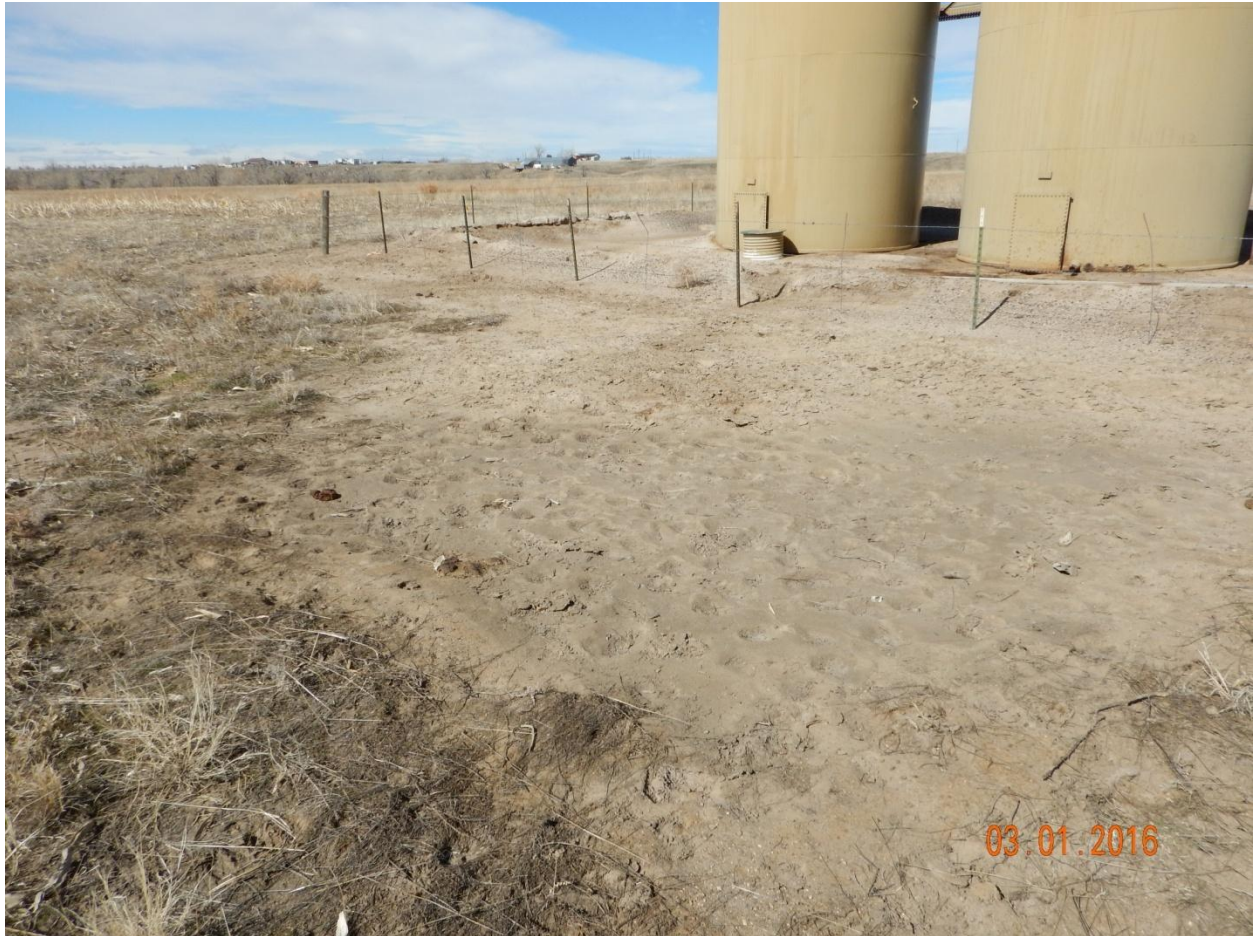
Figure 6 – Absence of vegetation south of tank battery and gap in berm.
