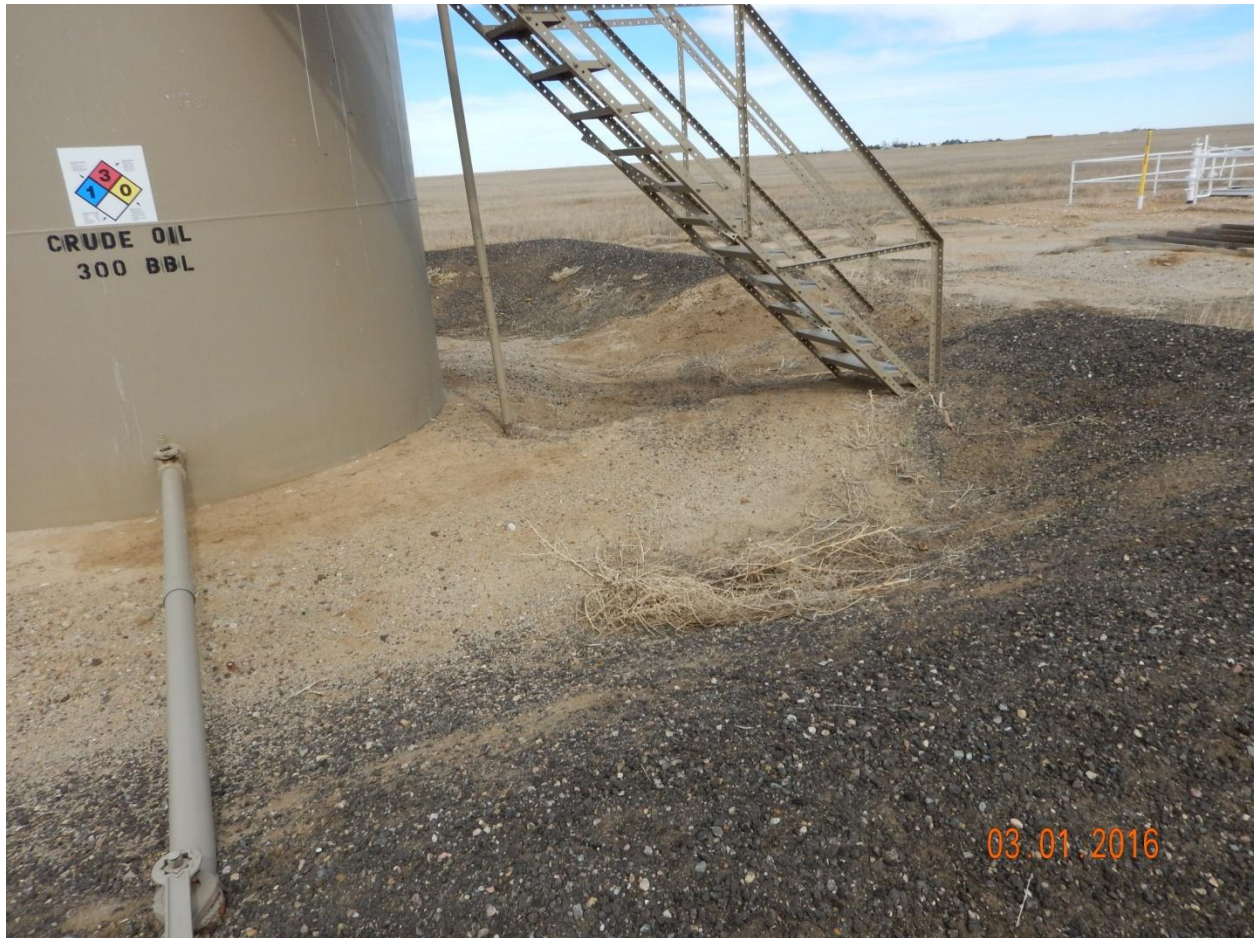
Figure 2 – Vegetation growth inside of tank battery berm.
