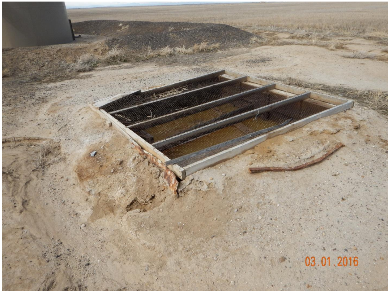
Figure 3 – Stained soil, maintenance issues, and gaps in wildlife protection at skim pit.
