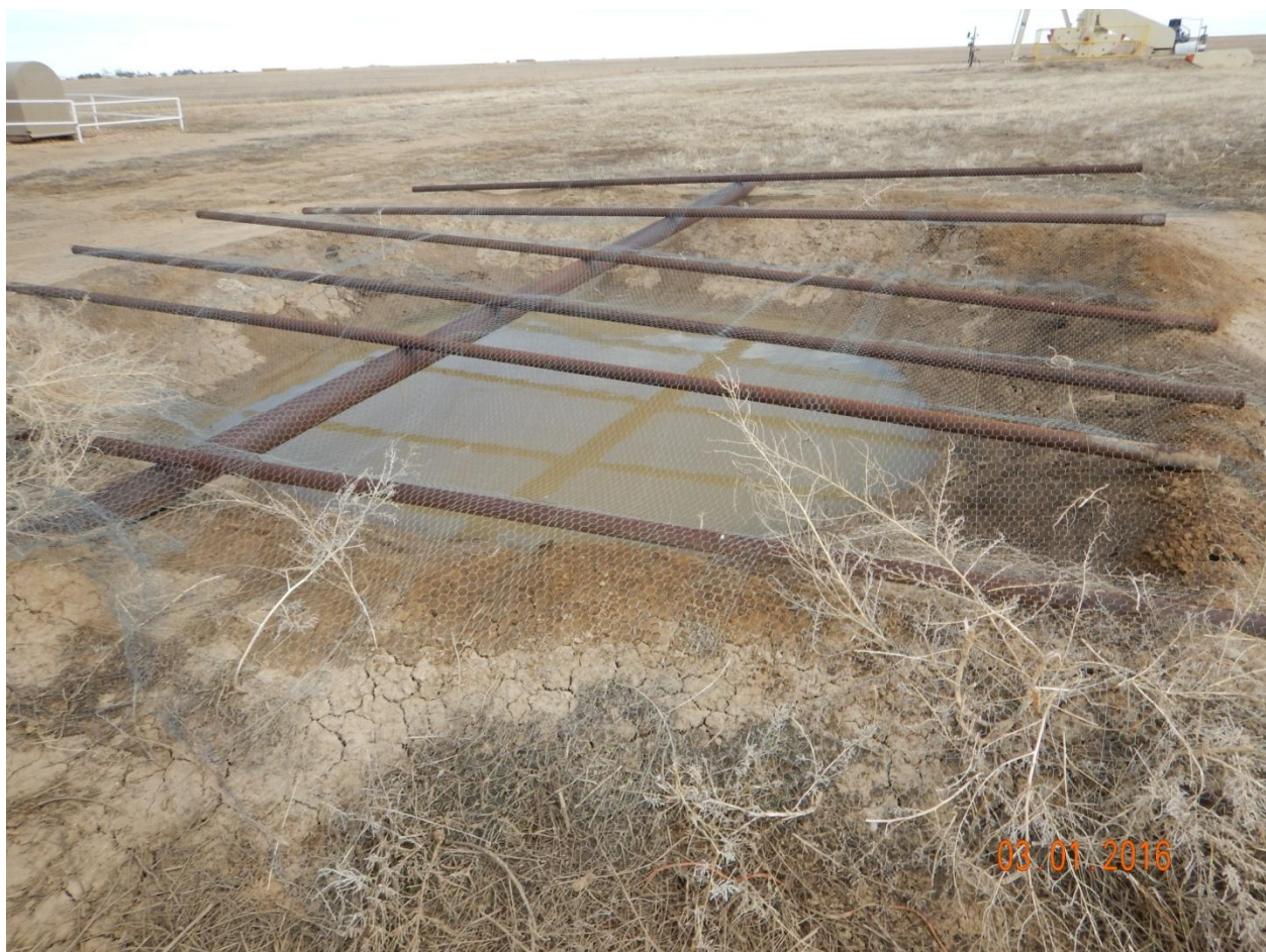
Figure 6 – Oil-stained soil inside of pit (along south and west walls), vegetation growth and wind-blown weeds accumulating outside of pit along west wall.
