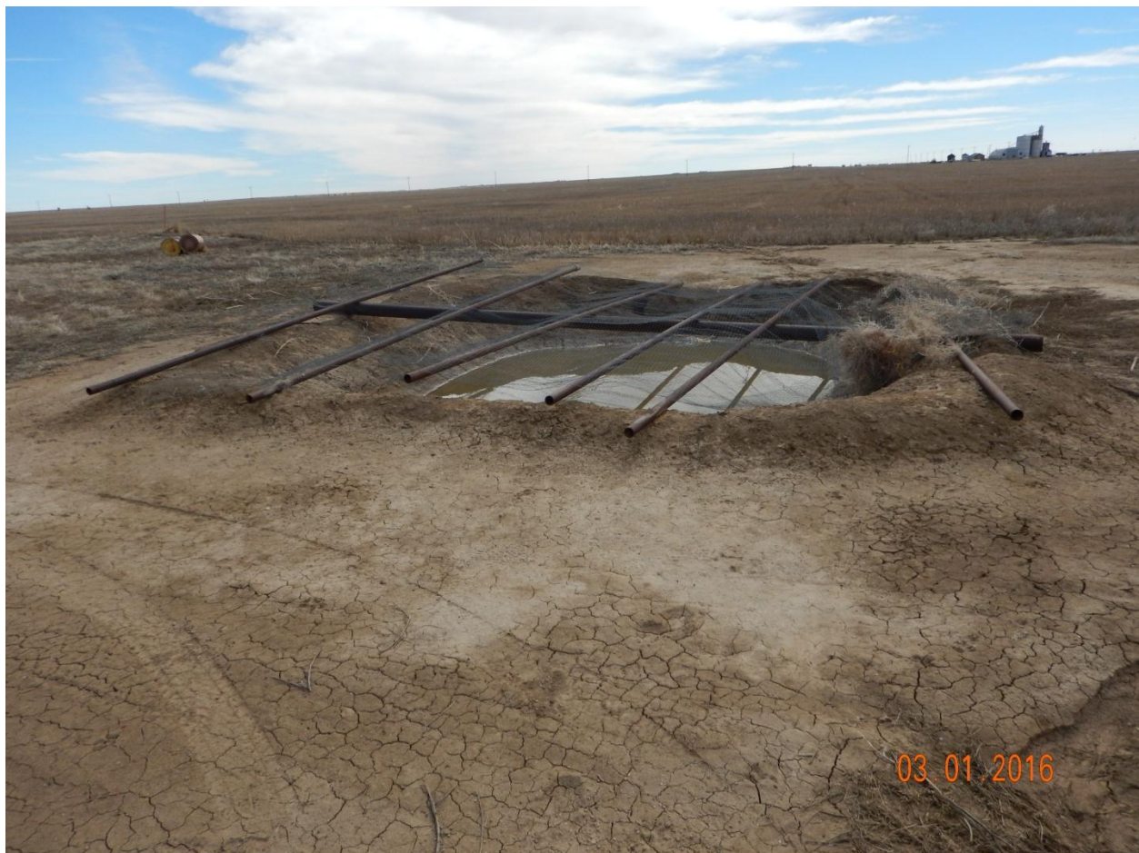
Figure 4 - View of produced water pit from northwest corner. Note sagging wildlife protection mesh and tumbleweeds encroaching on pit from the west.
