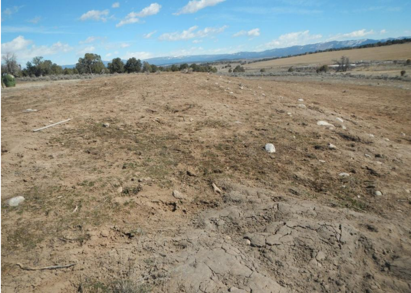
Photo 2. View of the southern portion of the project area from the southwestern corner facing eastward. Poor revegetation observed on this slope needs to be monitored and re-seeded in 2016 if vegetative cover is not increasing.
