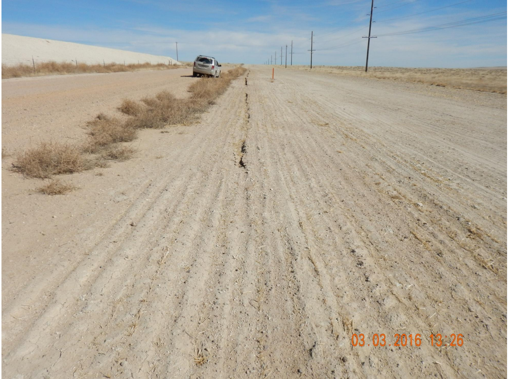
Figure 44: Photo taken from pipeline reclamation project, south of location facing east. Photo shows either subsidence or stormwater erosion occurring on pipeline.
