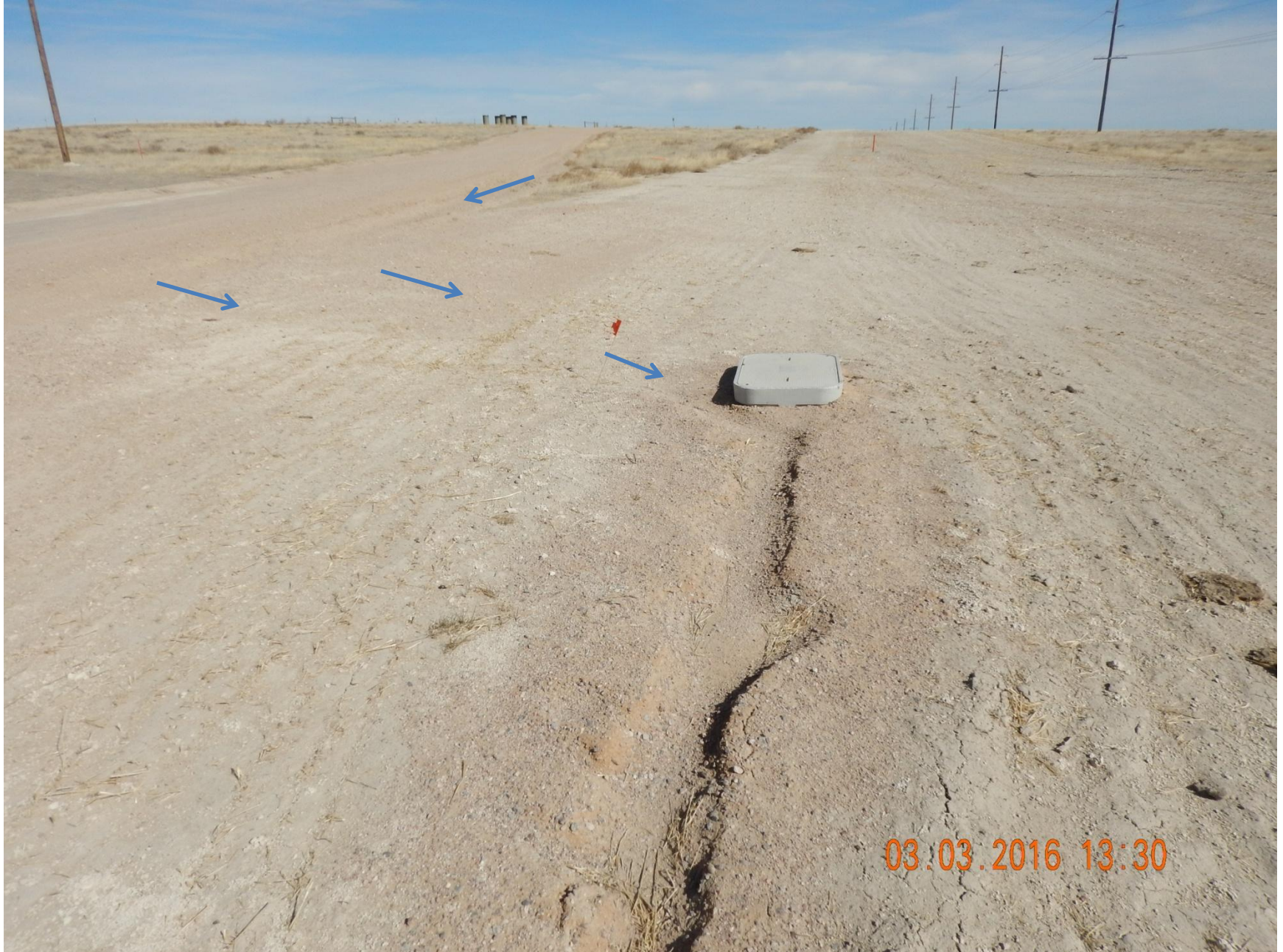
Figure 50: Photo taken from pipeline reclamation project, south of location facing east. Photo shows either subsidence or stormwater erosion occurring on pipeline. Note stormwater movement patterns off access road ditch leading into reclamation project.
