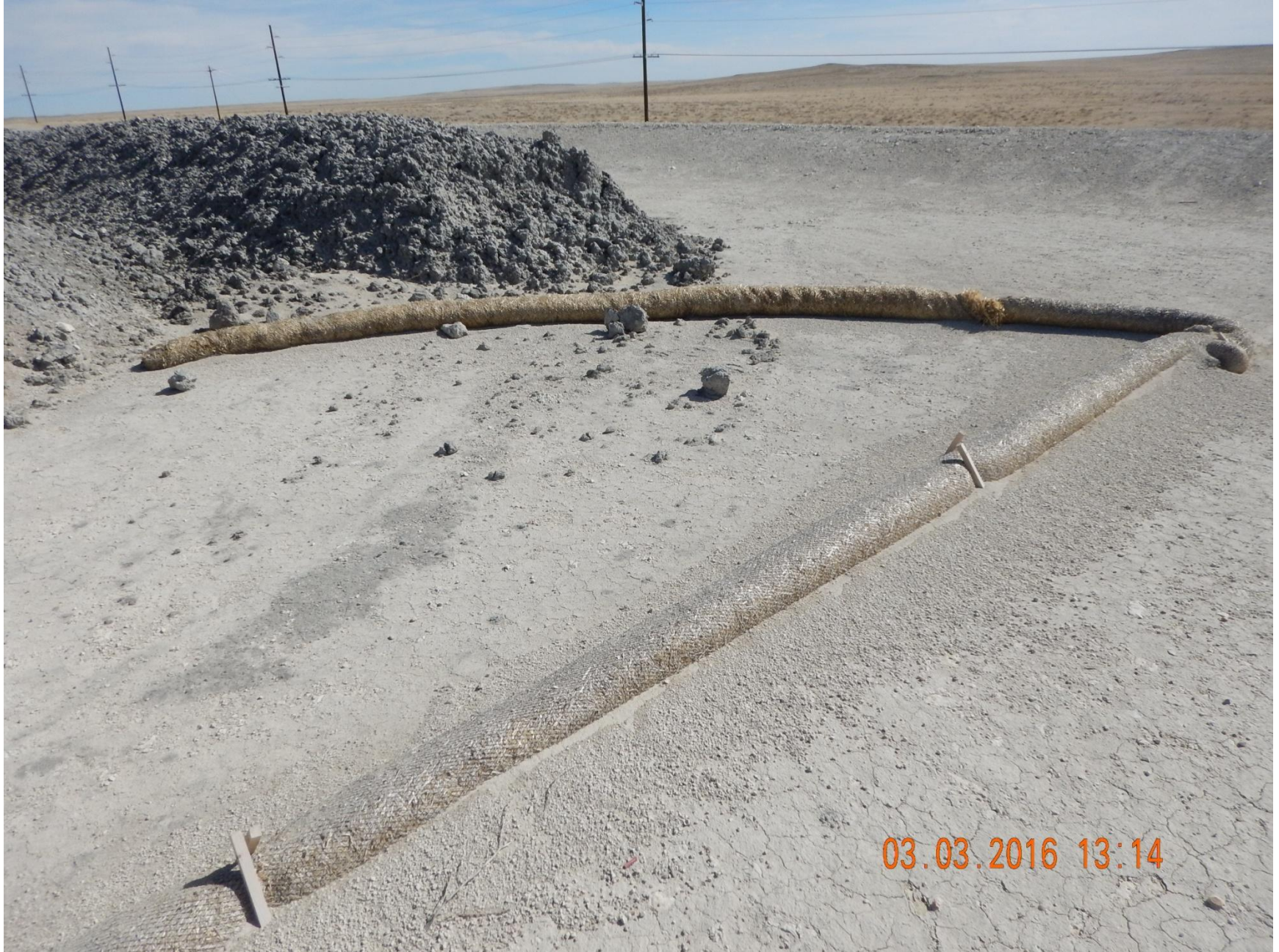
Figure 29: Photo taken from the southern end of the location, facing south. Photo shows straw wattles used as a stormwater and sediment control BMP around drill cuttings in disrepair.
