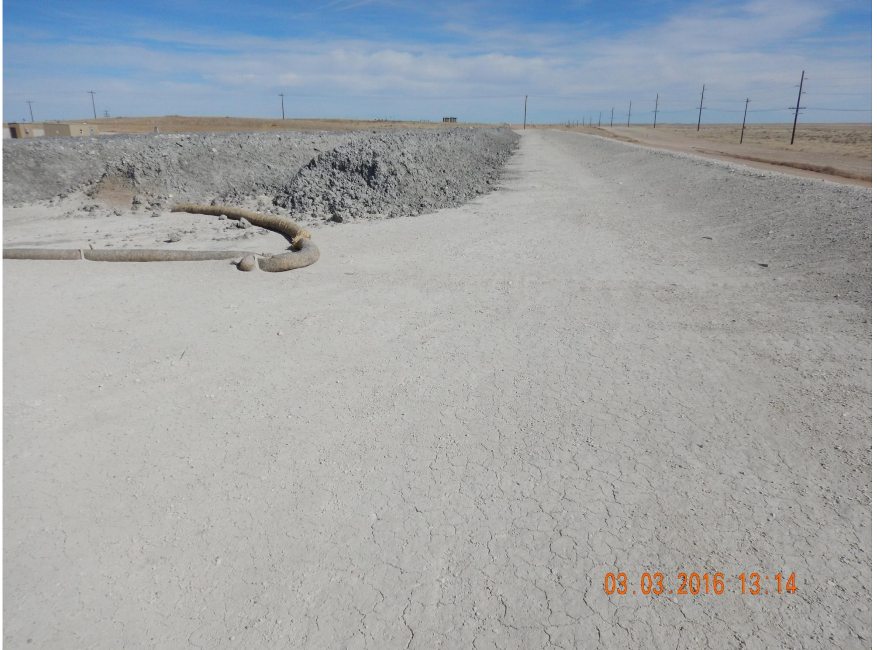
Figure 30: Photo taken from the southern end of the location, facing east. Photo shows straw wattles used as a stormwater and sediment control BMP around drill cuttings in disrepair.
