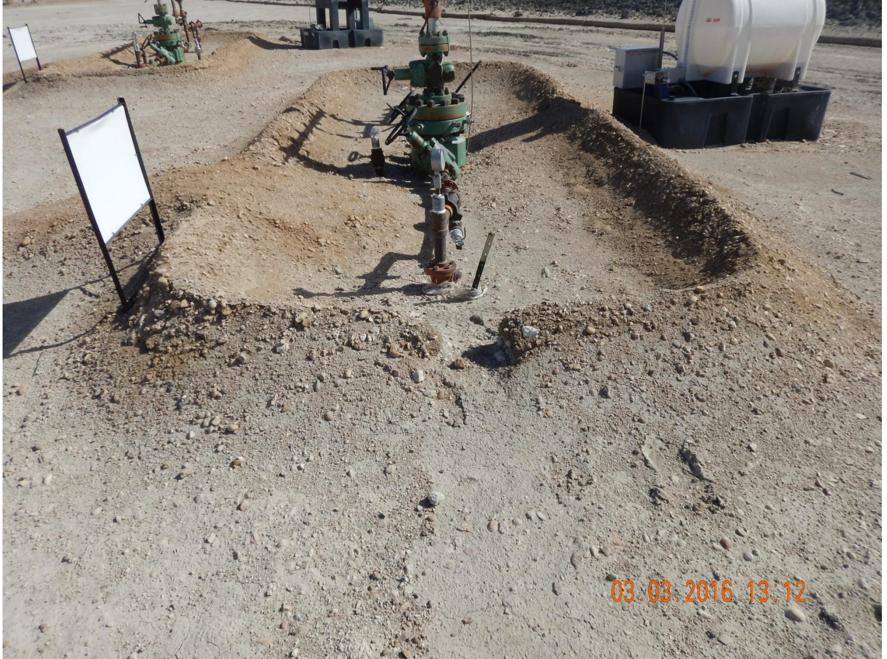
Figure 8: Photo taken from well #123-38060. Photo shows containment berm around well head in disrepair.
