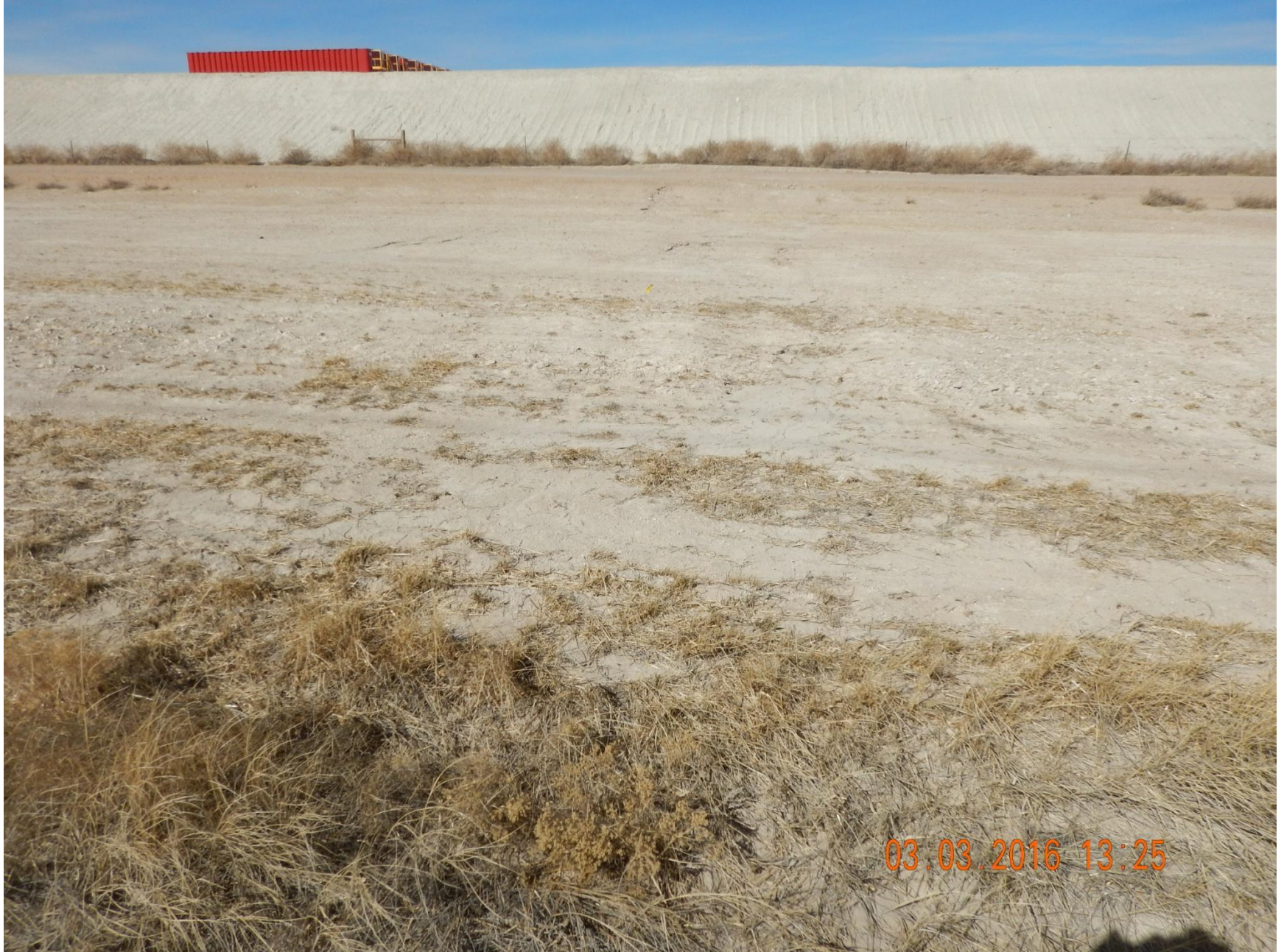
Figure 40: Photo taken from south of pipeline, facing north towards location. Photo shows stormwater erosion runoff from road, over a pipeline reclamation project, and onto adjacent lands.
