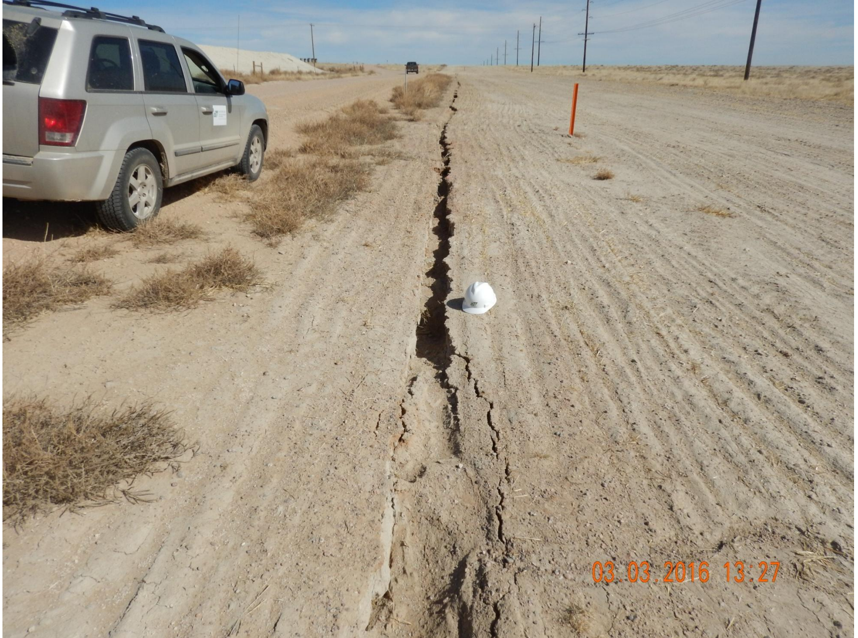
Figure 45: Photo taken from pipeline reclamation project, south of location facing east. Photo shows either subsidence or stormwater erosion occurring on pipeline.
