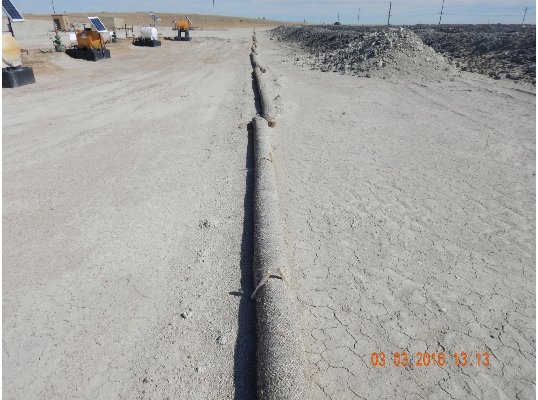
Figure 27: Photo taken from southern end of the location, facing east. Photo shows straw wattles used as a stormwater and sediment control BMP around drill cuttings.
