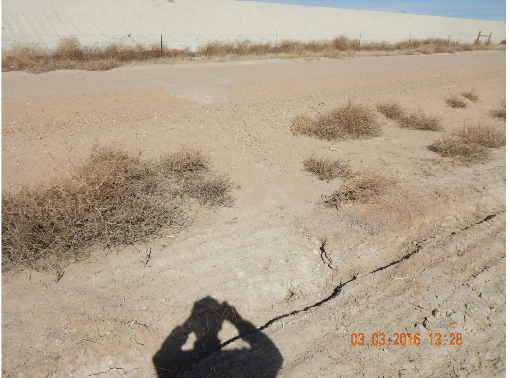
Figure 46: Photo taken from pipeline reclamation project, south of location facing east. Photo shows stormwater runoff from access road causing erosion on pipeline reclamation project.
