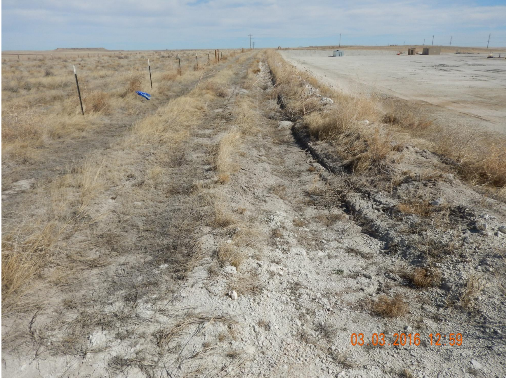
Figure 16: Photo taken from the northwest end of location, facing east. Phot shows stormwater and sediment control BMP ditch used on the north end of the location.
