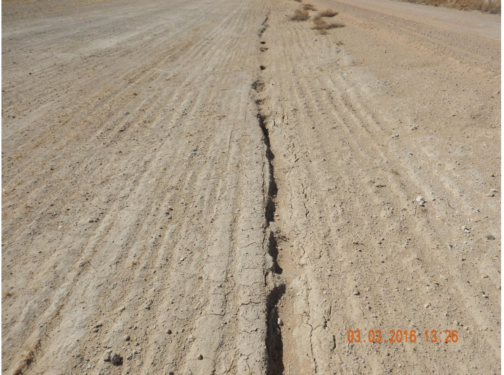
Figure 41: Photo taken from pipeline reclamation project, south of location facing west. Photo shows either subsidence or stormwater erosion occurring on pipeline.
