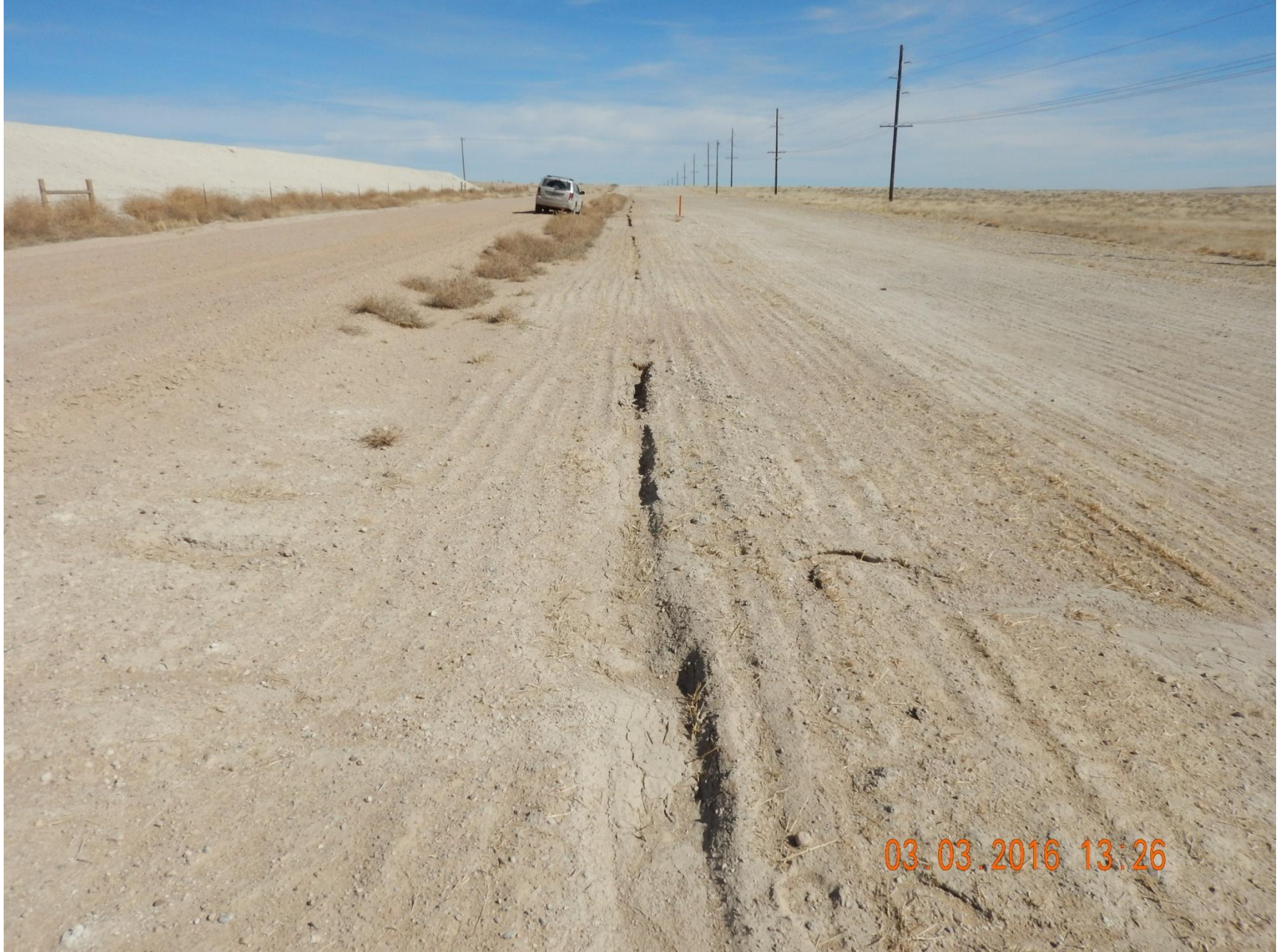
Figure 42: Photo taken from pipeline reclamation project, south of location facing east. Photo shows either subsidence or stormwater erosion occurring on pipeline. Photo also shows stormwater erosion runoff from access road.
