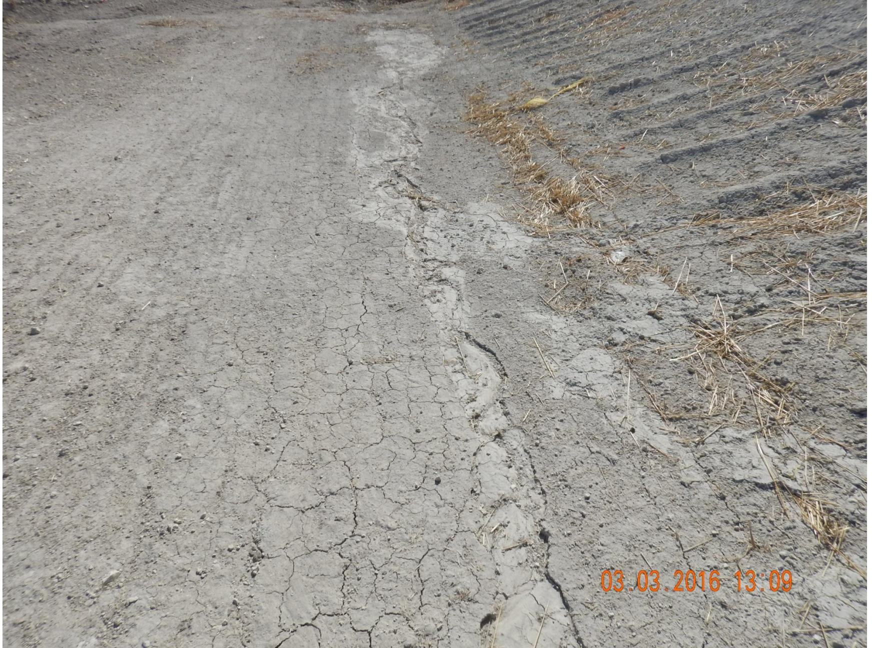
Figure 26: Photo taken at the toe of the slope on the east end of the project area, facing south. Photo shows erosion and water movement patterns.
