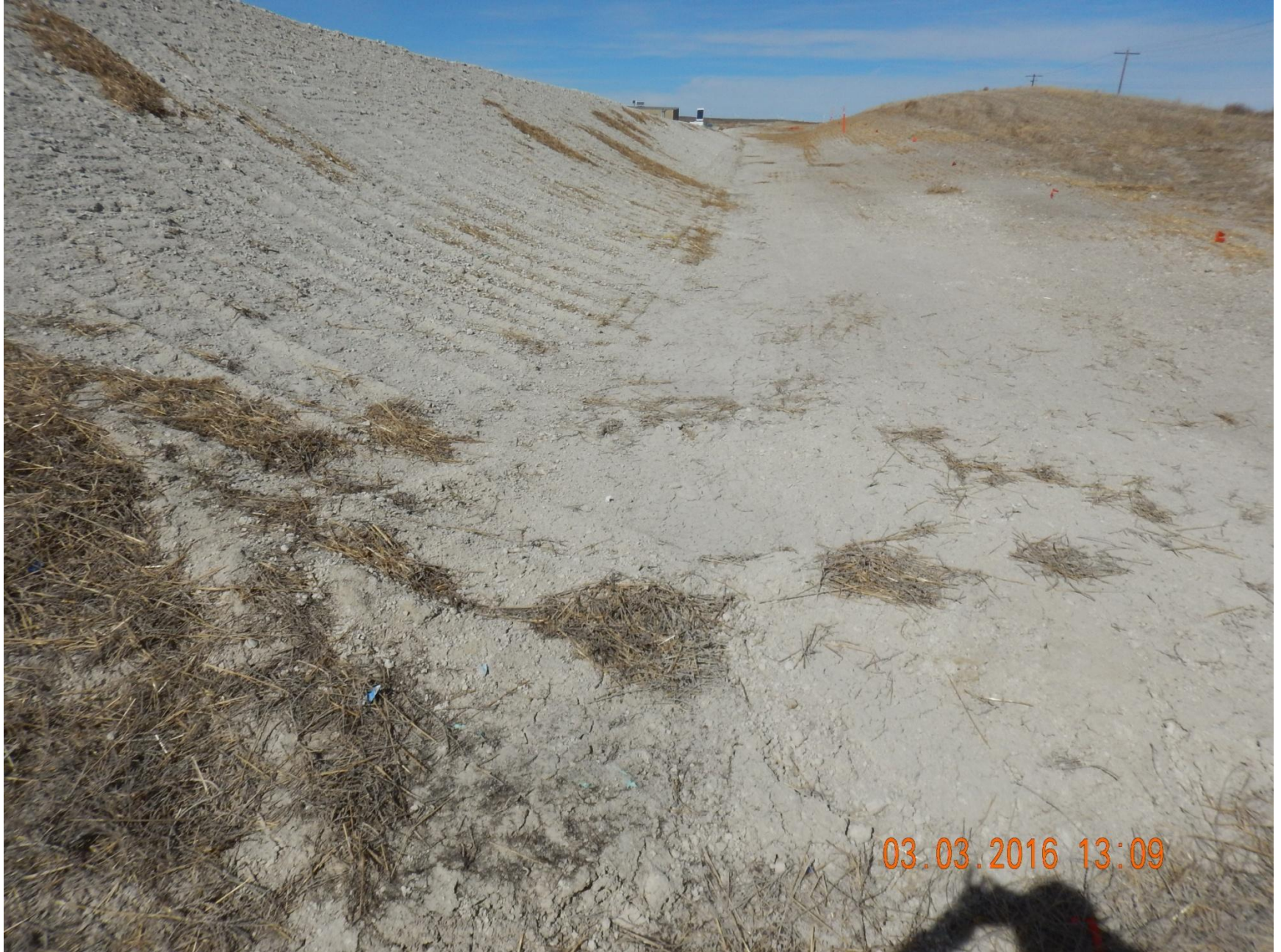
Figure 25: Photo taken from the southeast end of the project area, facing north. Photo shows slope, and vehicle tracking used as a stormwater and sediment control BMP.
