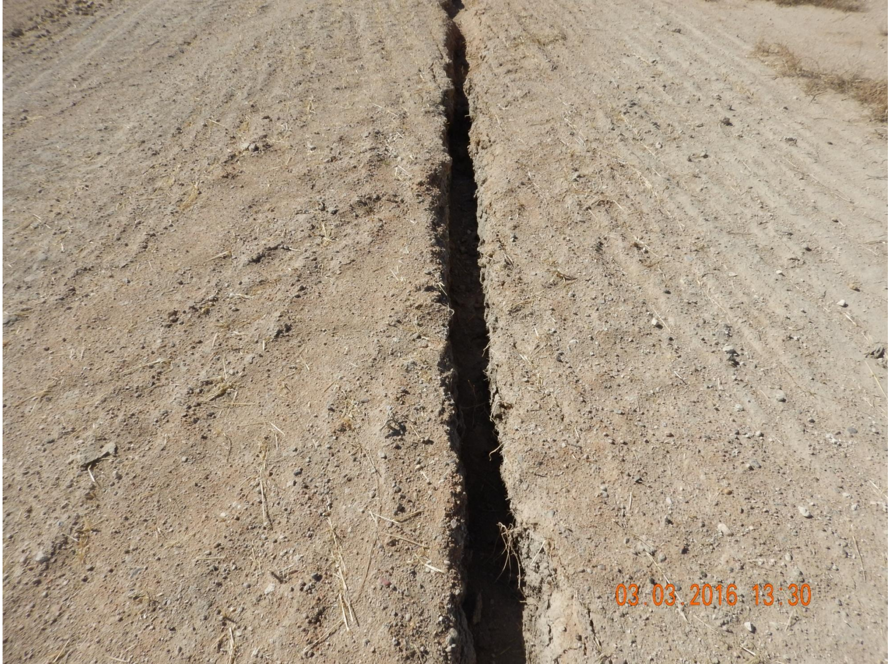
Figure 51: Photo taken from pipeline reclamation project, southeast of location facing west. Photo shows either subsidence or stormwater erosion occurring on pipeline.
