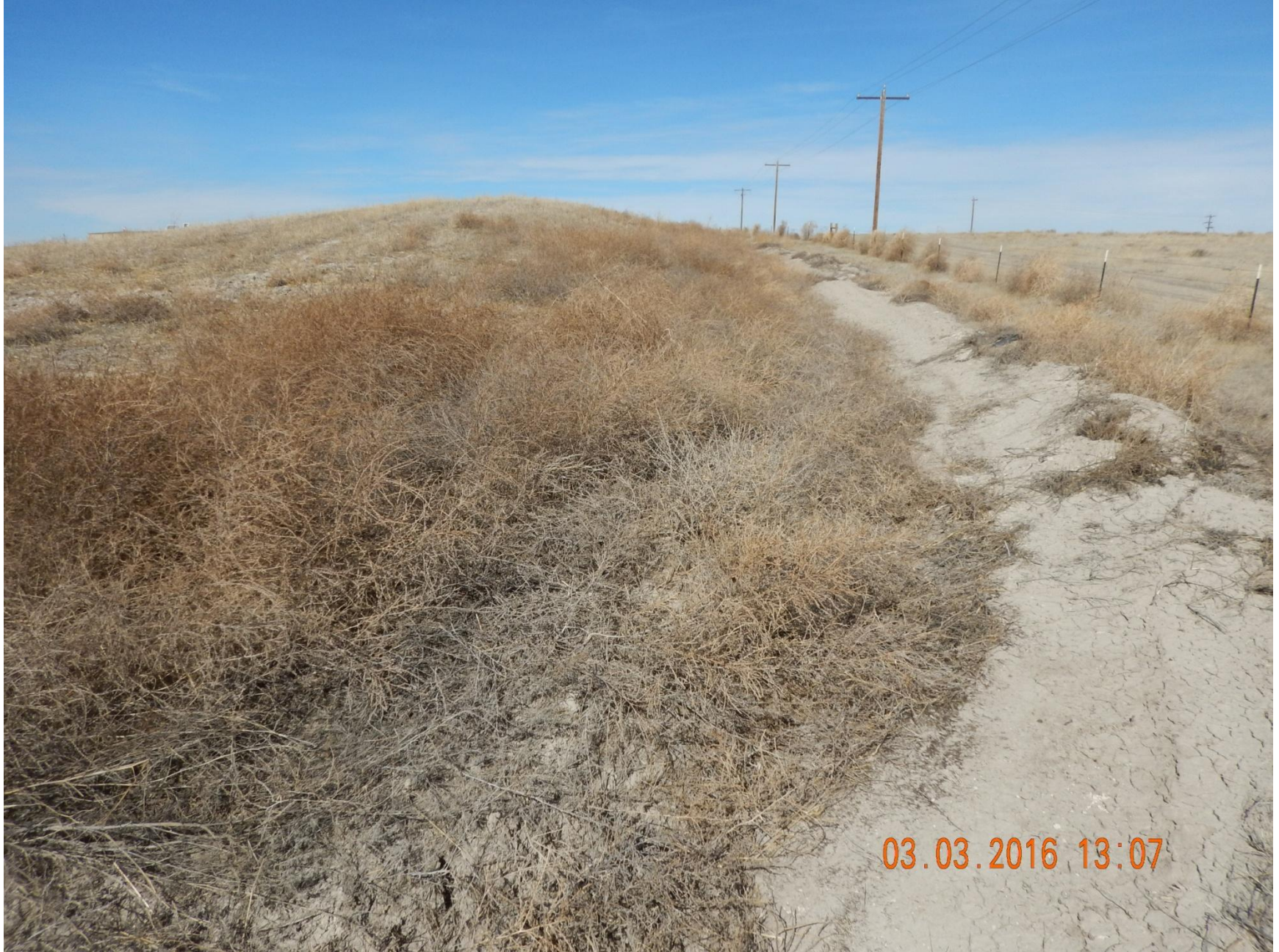
Figure 23: Photo taken from the southeast corner of the interim area, facing north. Photo shows stormwater and sediment control ditch. Note vegetation on interim area predominantly undesirable weedy vegetation.
