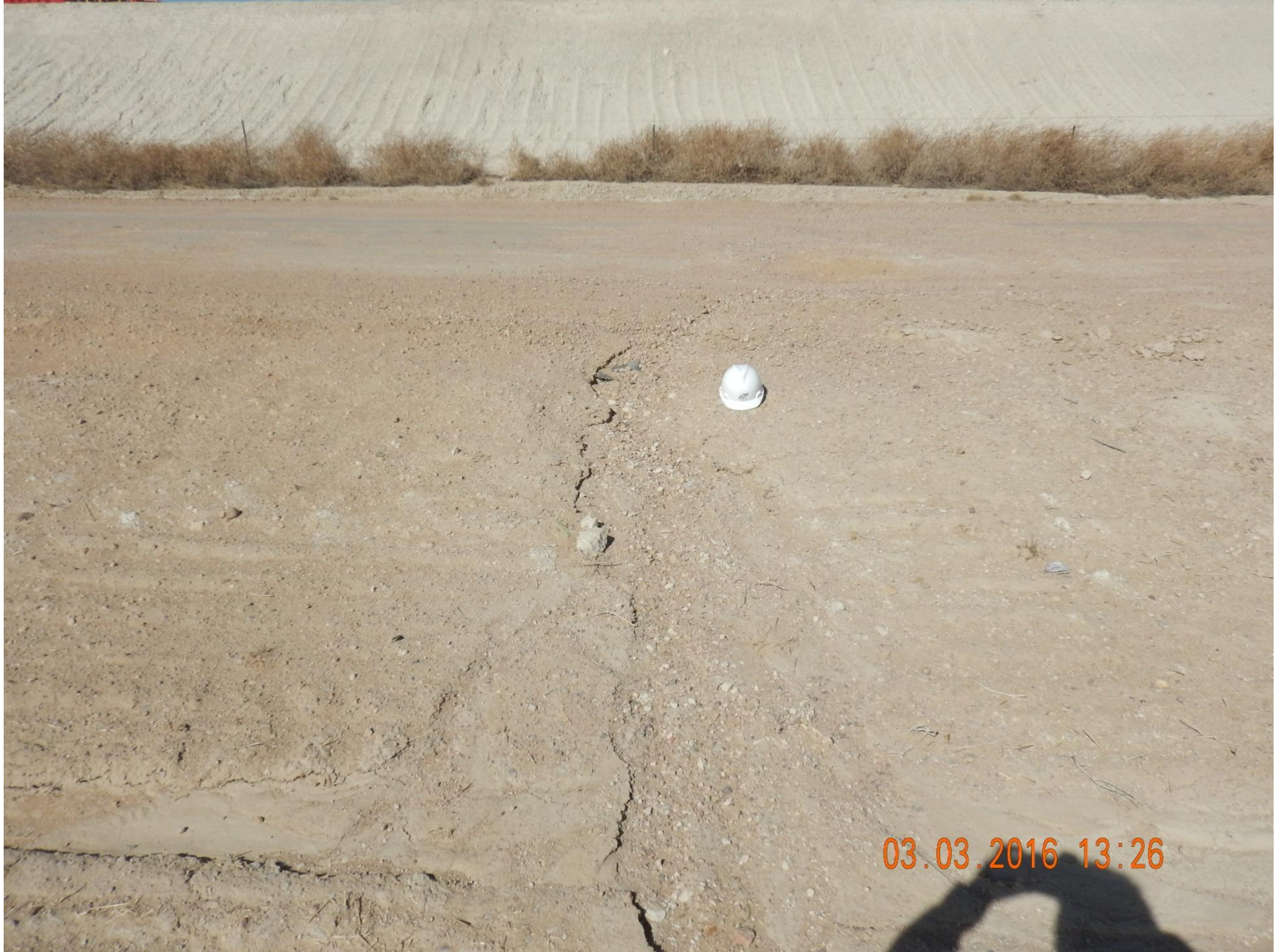
Figure 43: Photo taken from pipeline reclamation project, south of location. Photo shows stormwater erosion runoff from the access road.
