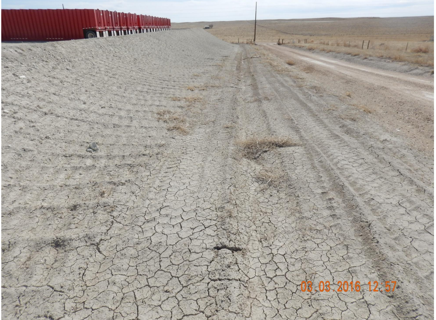
Figure 11: Photo taken from the west end of the location, facing south. Photo shows vehicle tracking on the slope of the pad, and a stormwater and sediment control BMP ditch.
