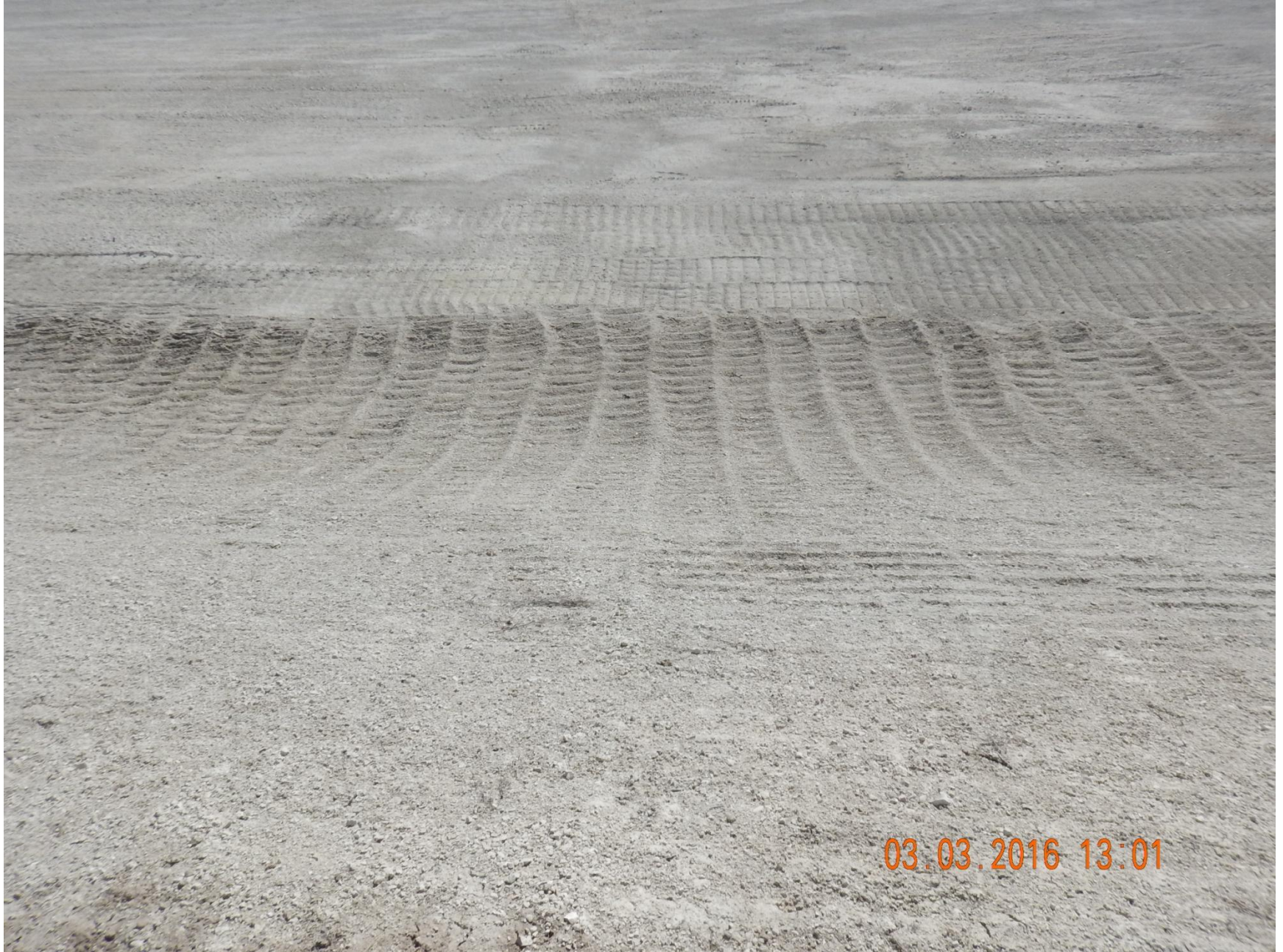
Figure 17: Photo taken from the north end of the location, facing south. Photo shows vehicle tracking used as a stormwater and sediment control BMP on the slope.
