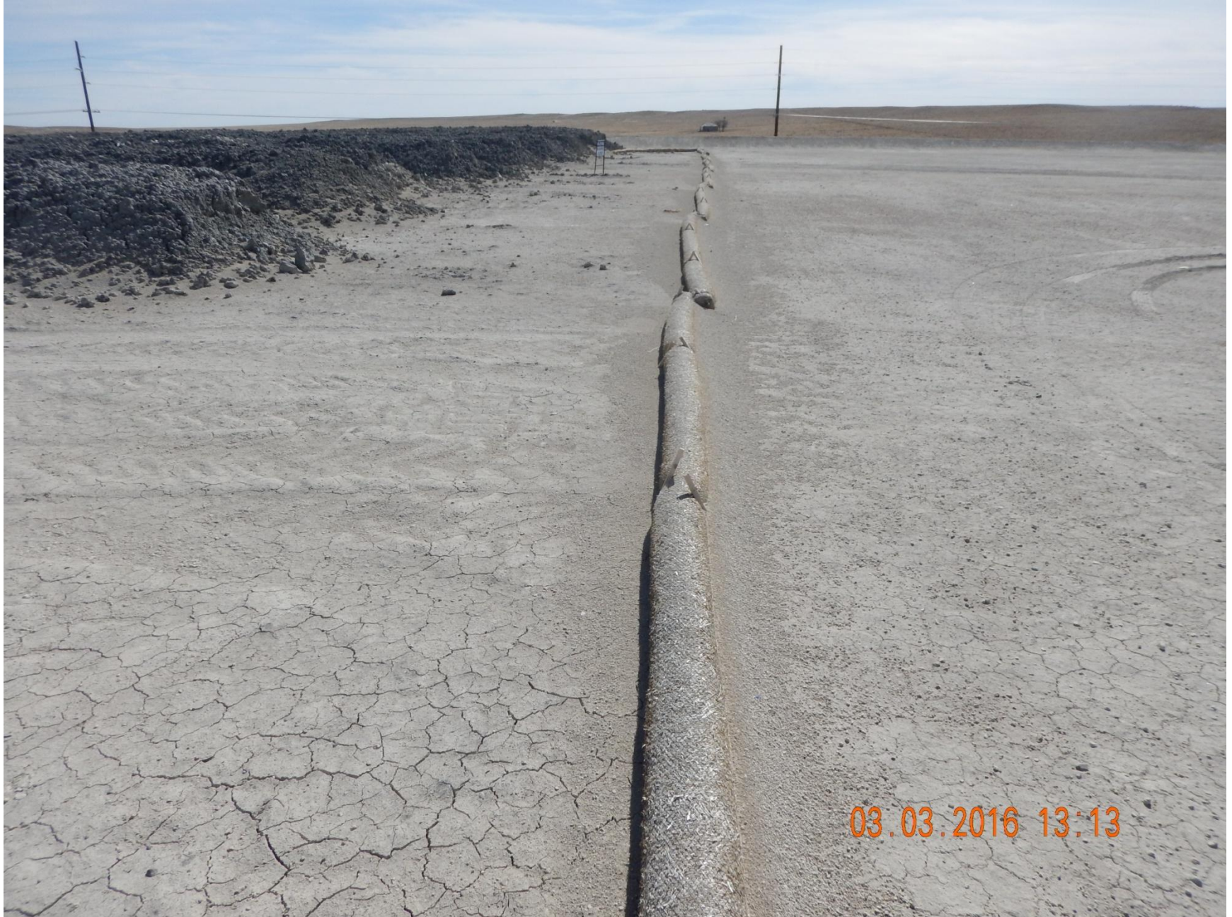
Figure 28: Photo taken from southern end of the location, facing south. Photo shows straw wattles used as a stormwater and sediment control BMP around drill cuttings.
