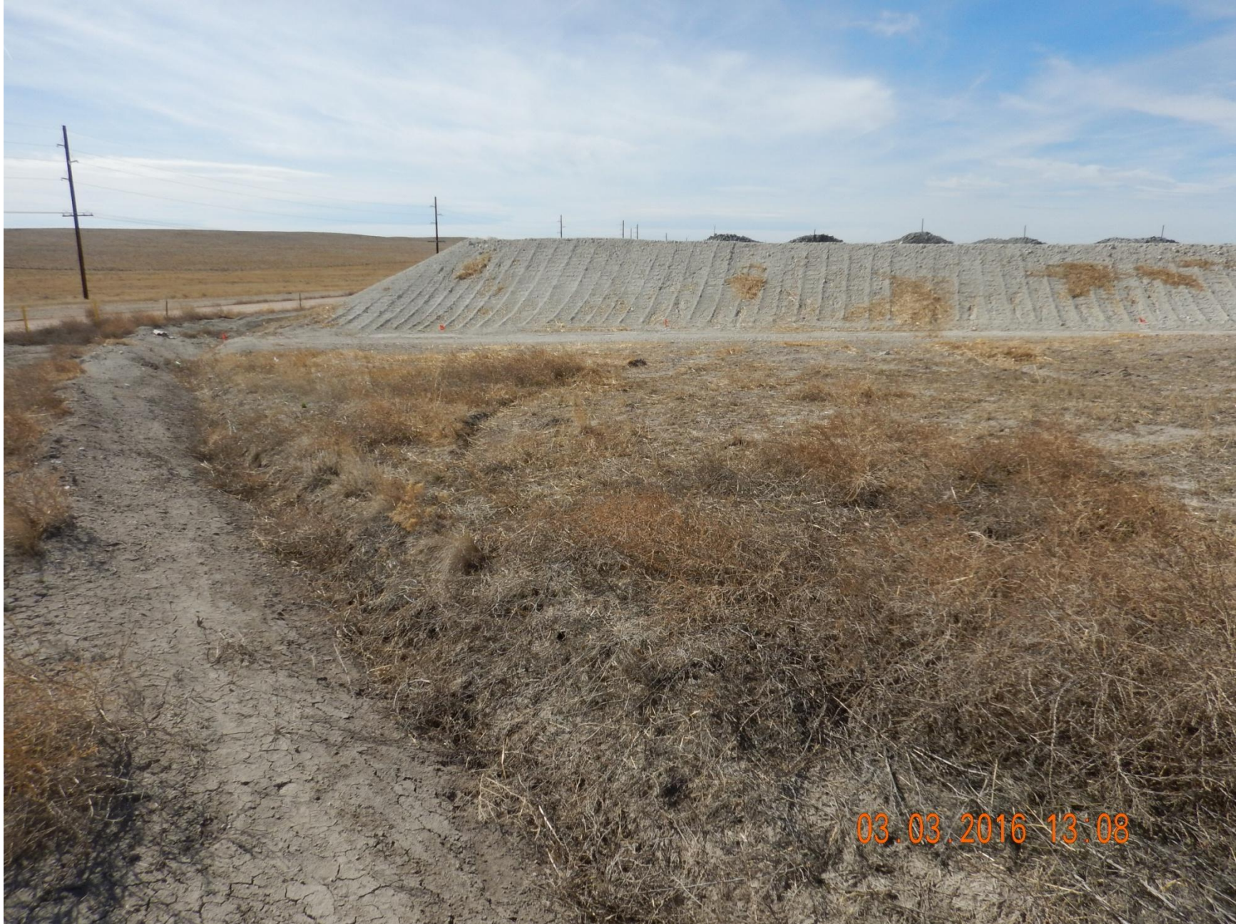
Figure 24: Photo taken from the southeast corner of the interim area, facing west. Photo shows stormwater and sediment control ditch, and slope at the project area. Note vegetation on interim area predominantly undesirable weedy vegetation.
