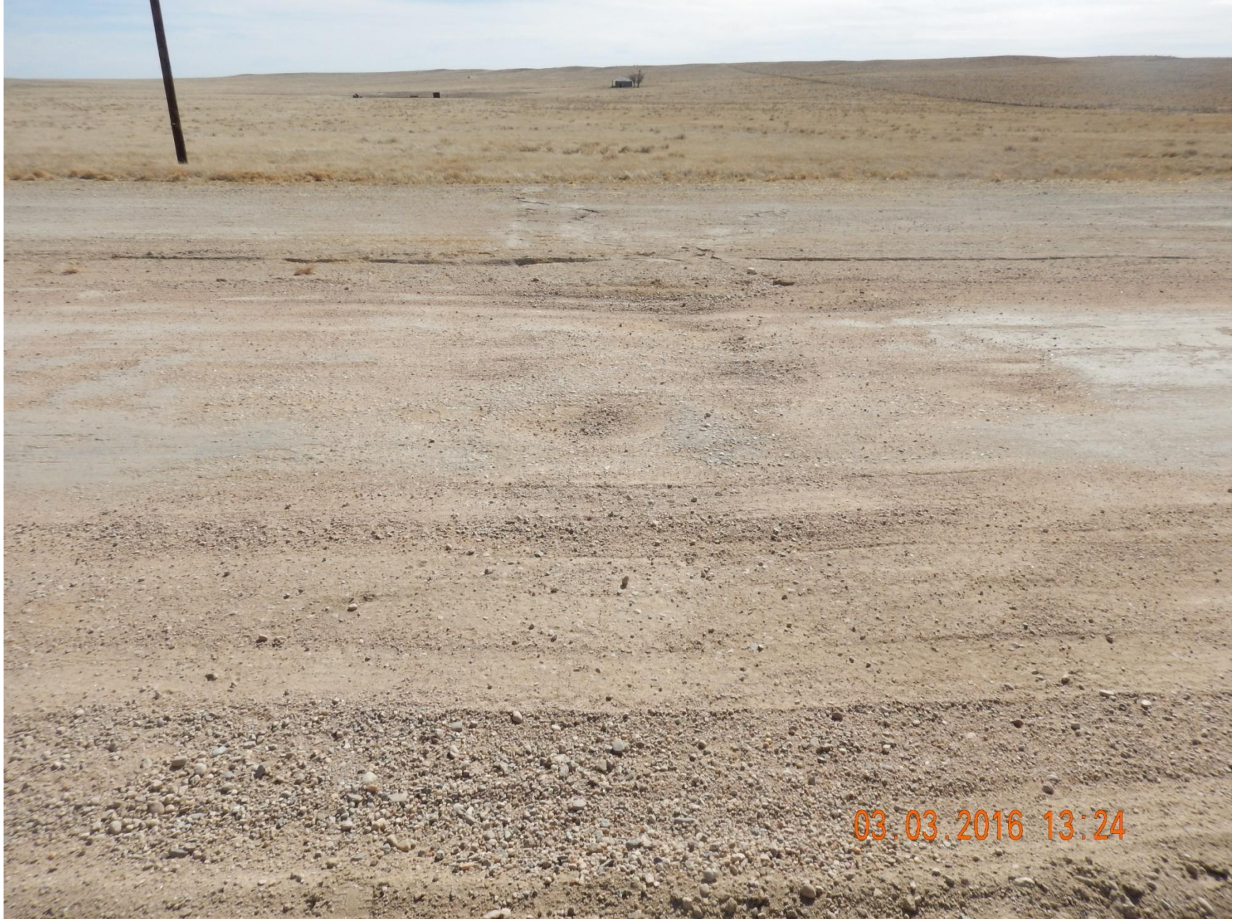
Figure 37: Photo taken from the access road that runs east/west, south of the location, facing south. Photo shows stormwater erosion running off road, over a pipeline reclamation project, and onto adjacent lands.
