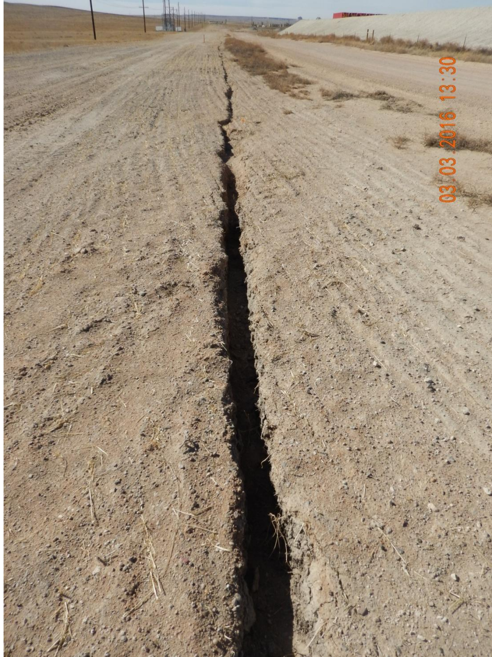
Figure 52: Photo taken from pipeline reclamation project, southeast of location facing west. Photo shows either subsidence or stormwater erosion occurring on pipeline.
