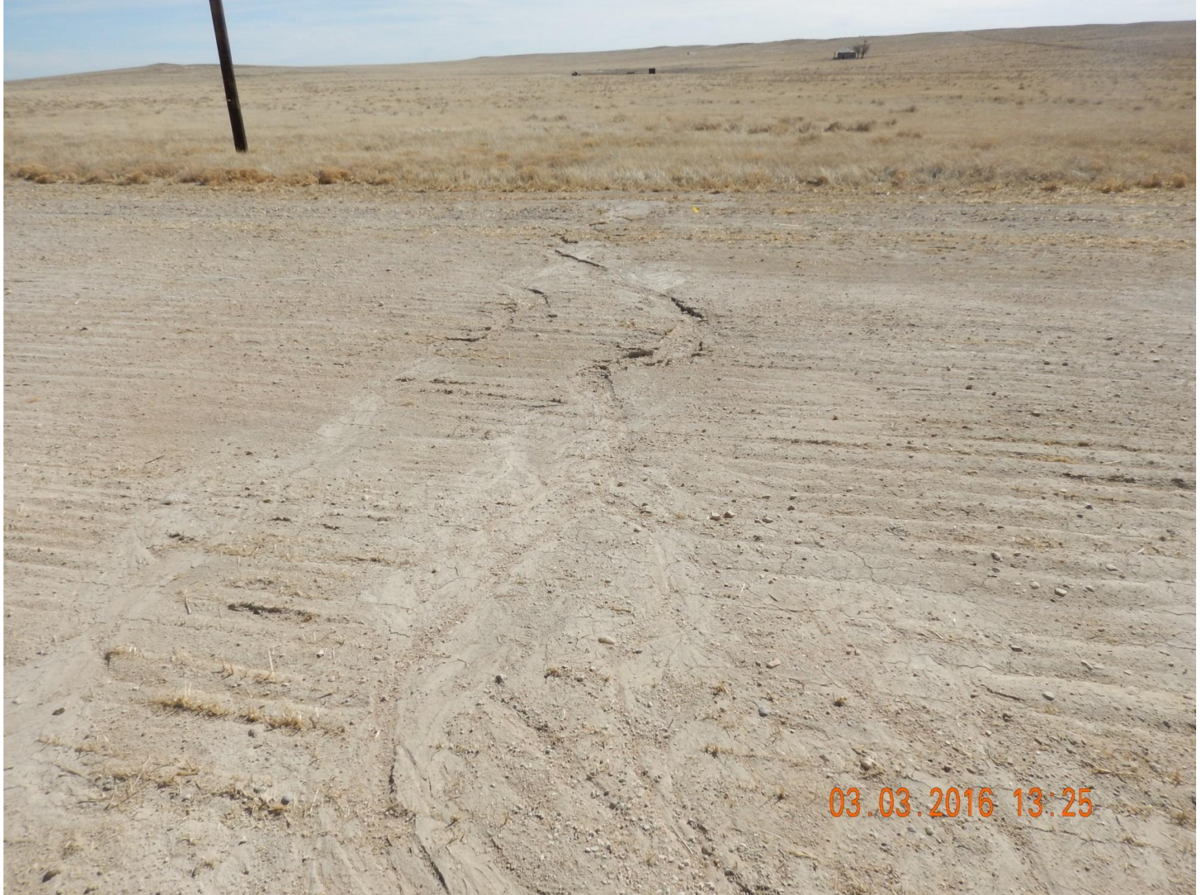
Figure 39: Photo taken from pipeline, south of the location, facing south. Photo shows stormwater erosion runoff from road, over a pipeline reclamation project, and onto adjacent lands.
