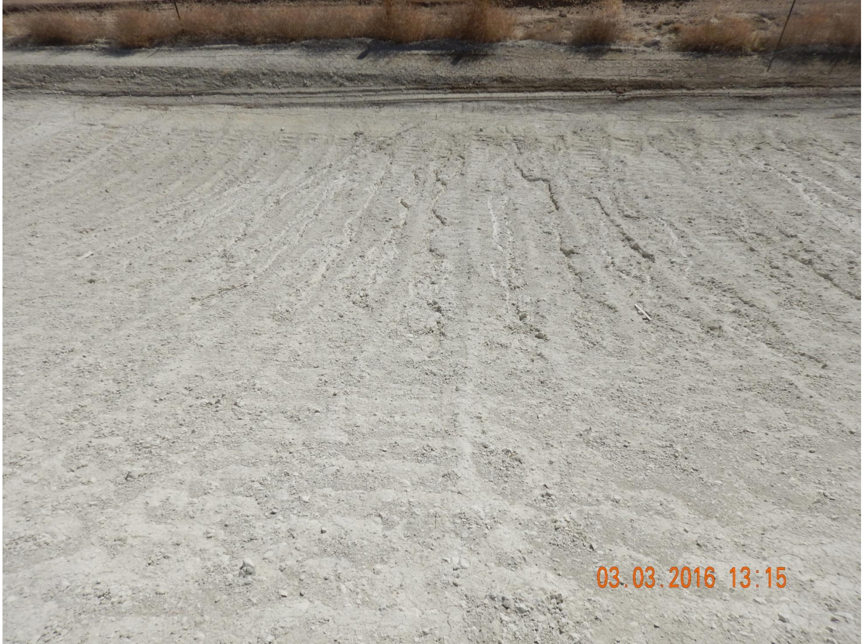
Figure 31: Photo taken from the south end of the location, facing south. Photo shows rill erosion beginning to form on the slope.
