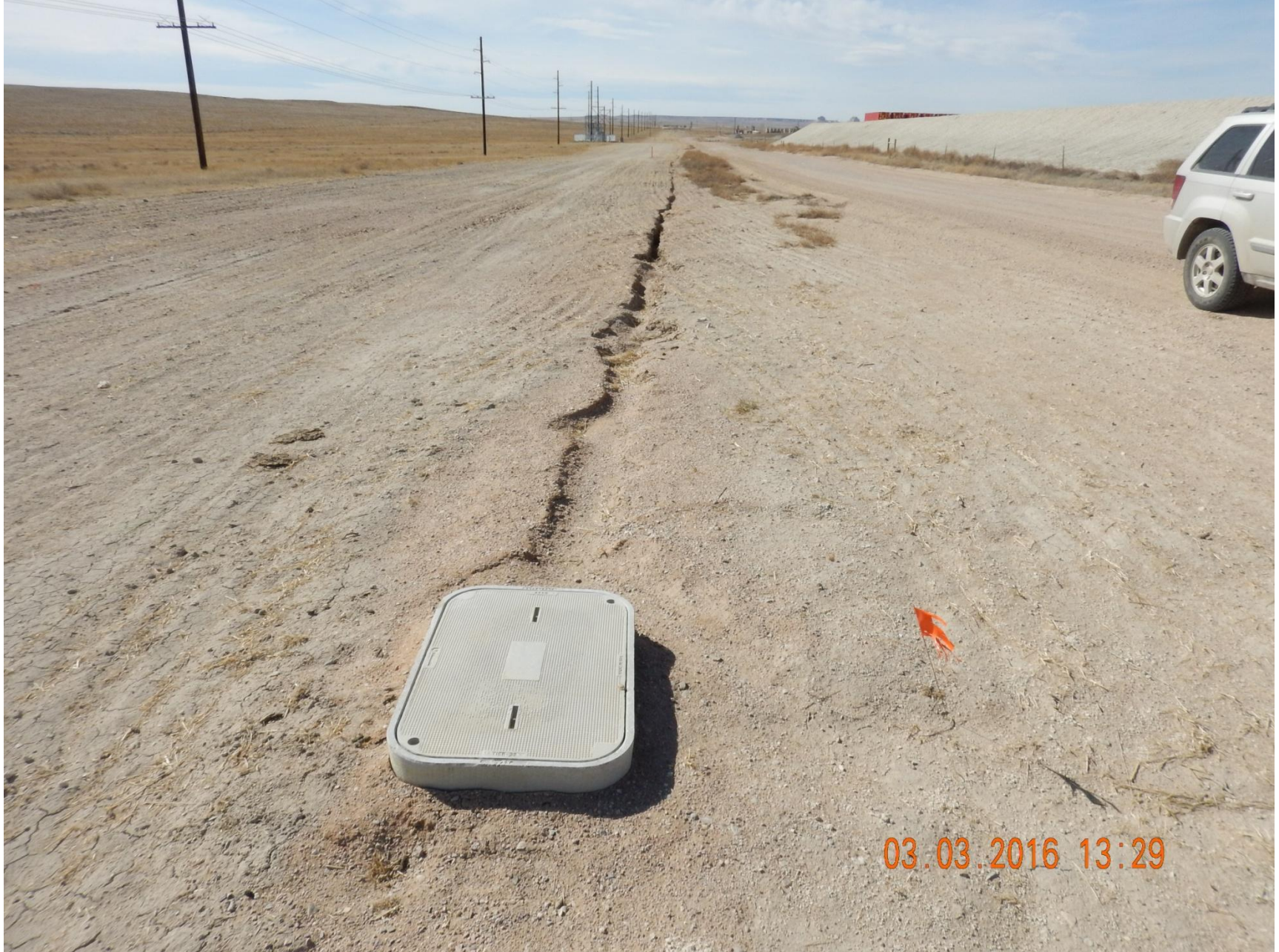
Figure 49: Photo taken from pipeline reclamation project, southeast of location facing west. Photo shows either subsidence or stormwater erosion occurring on pipeline.
