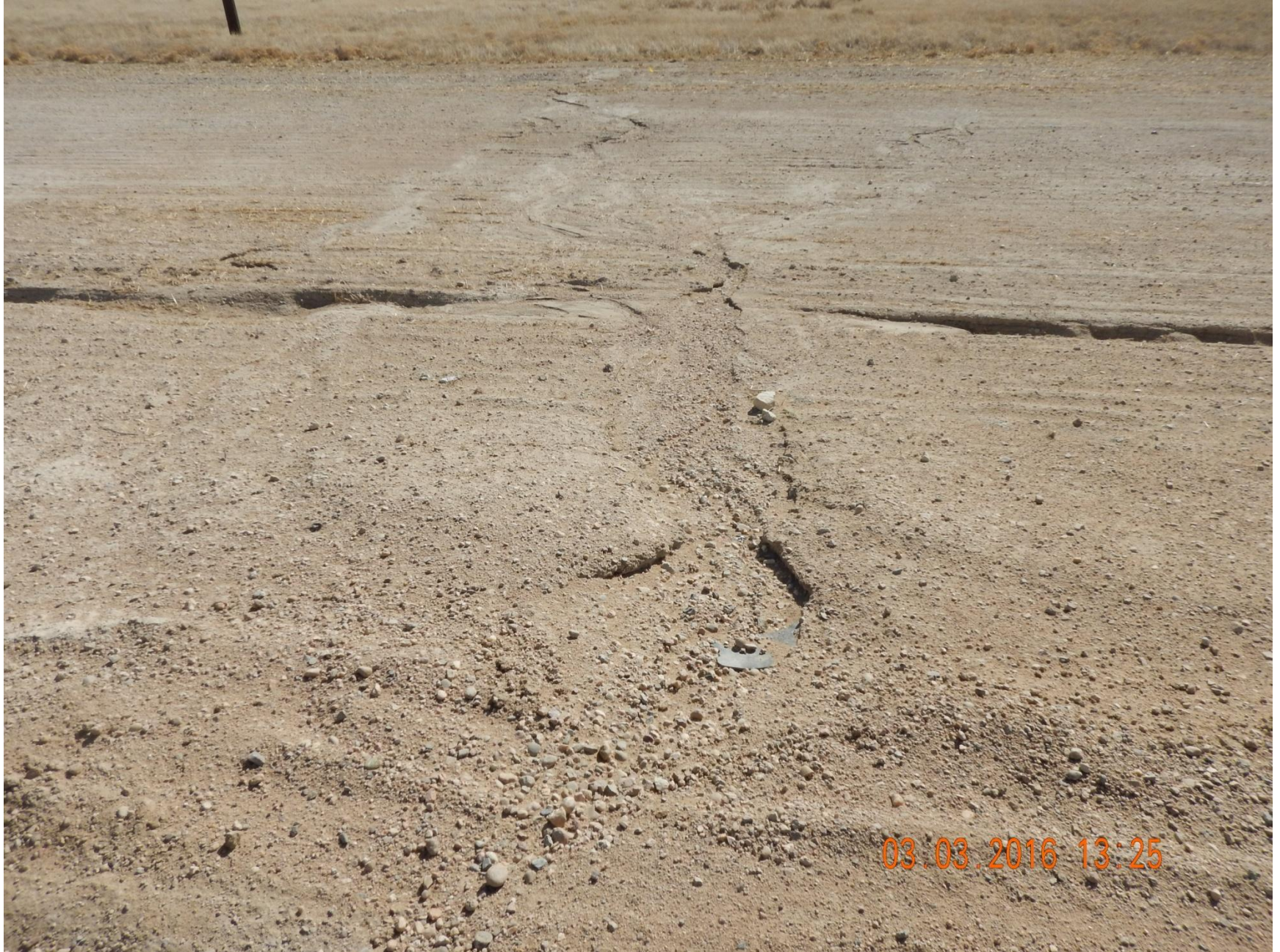
Figure 38: Photo taken from the access road that runs east/west, south of the location, facing south. Photo shows stormwater erosion running off road, over a pipeline reclamation project, and onto adjacent lands.
