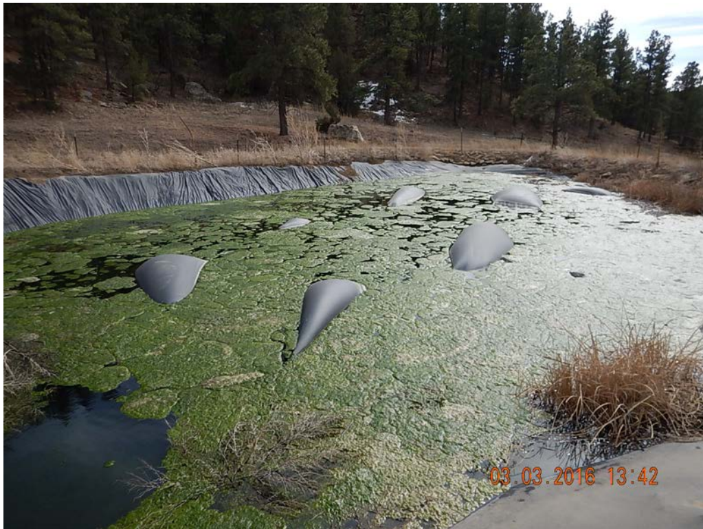
Figure 5 – Bubbles in pit liner and vegetation growing in pit.
