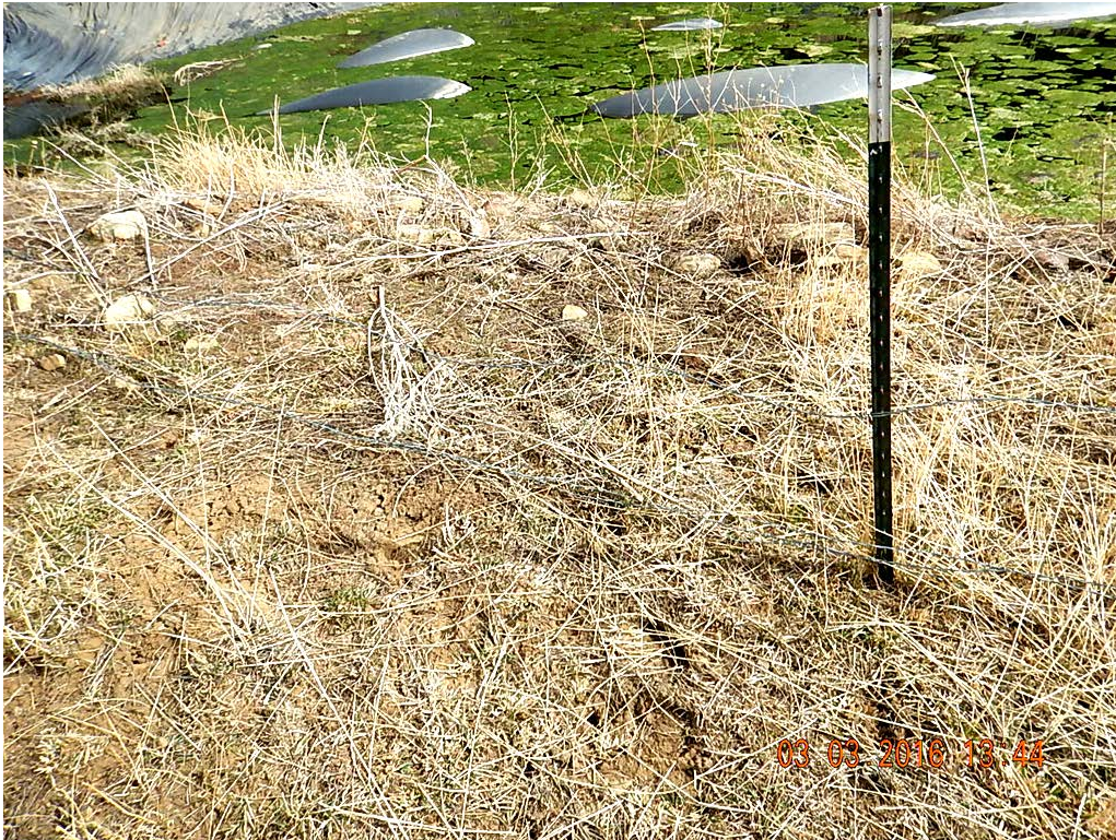
Figure 7 – Fencing is in disrepair.
