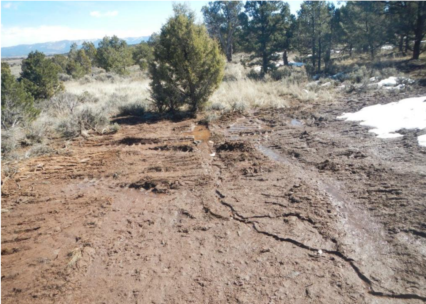
Photo 2. Another view of stormwater erosion occurring where sediment is being carried offsite into the grassy swale shown in Photo 1.
