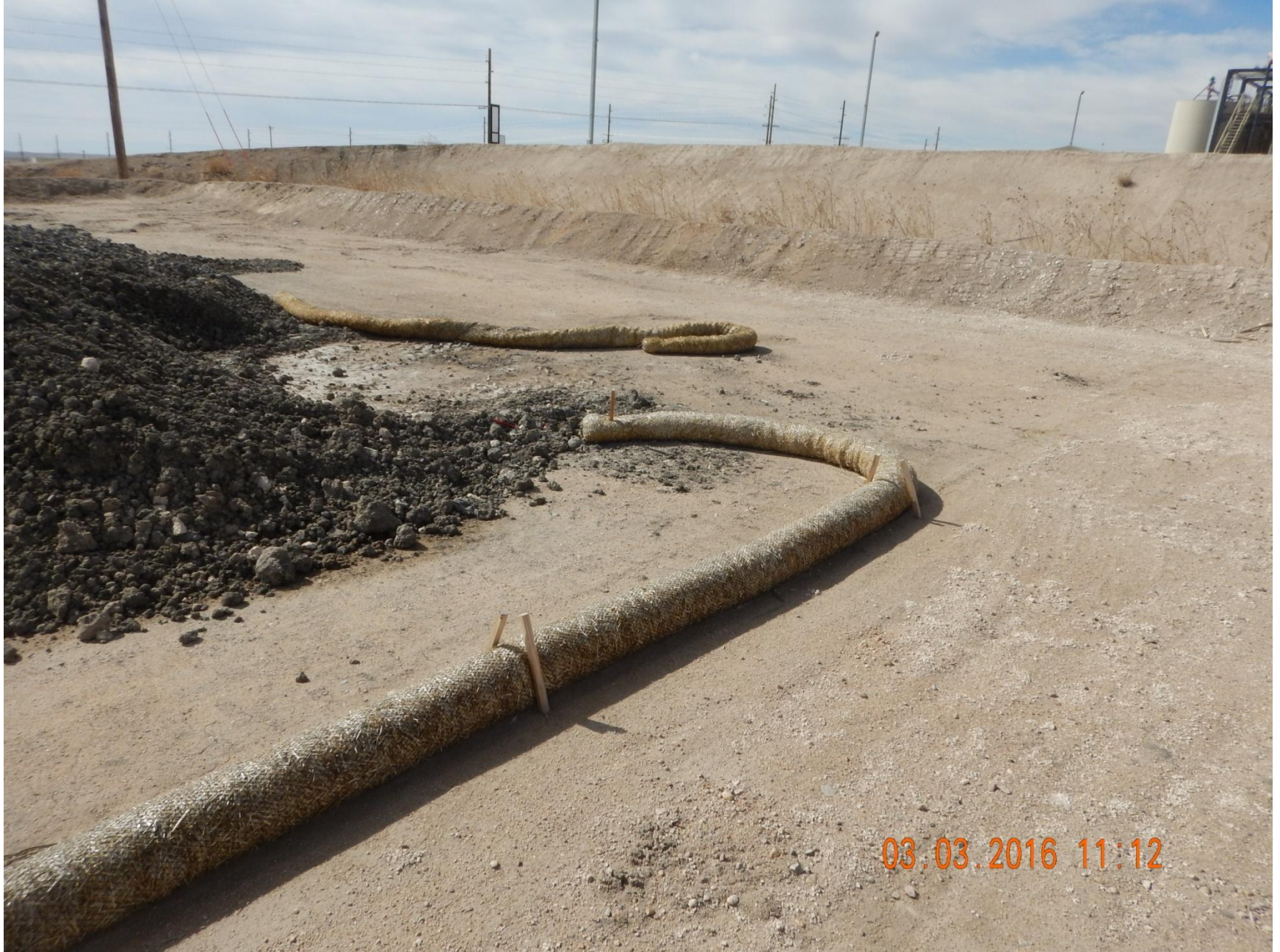
Figure 4: Photo taken from the west end of the location, facing southwest. Photo shows wattles in disrepair.
