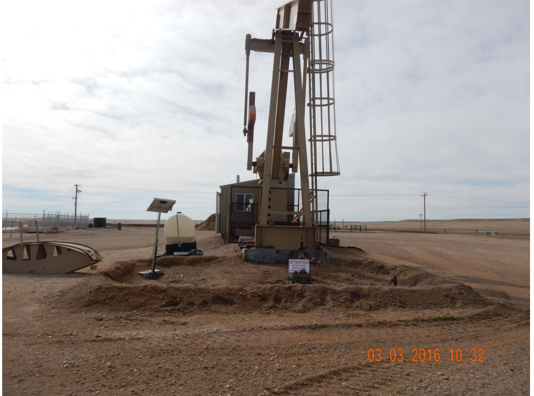
Figure 1: Photo taken from pump, facing south. Photo shows sign missing at wellhead.
