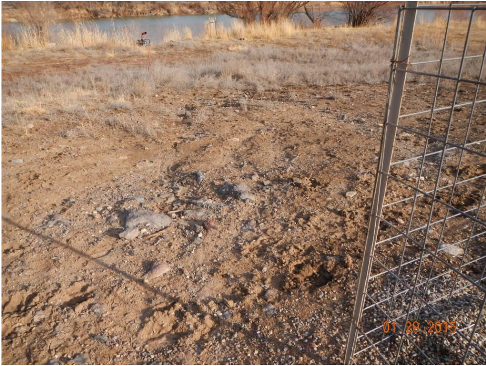
Second area of run-off and erosion 1/29/15
