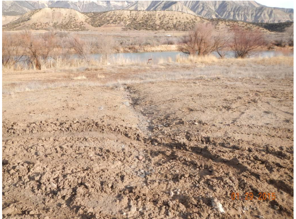
First area of stormwater run-off and erosion 1/29/15
