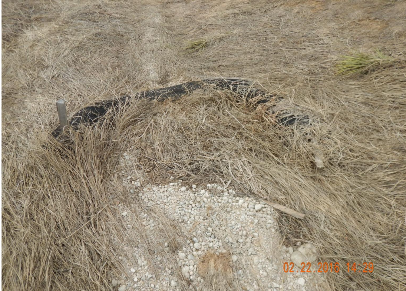
Photo 9. Photo taken from the western location, facing South. Stormwater and sediment BMPs need to be maintained to ensure controls are functioning properly. Wattle is full of sediment and debris.
