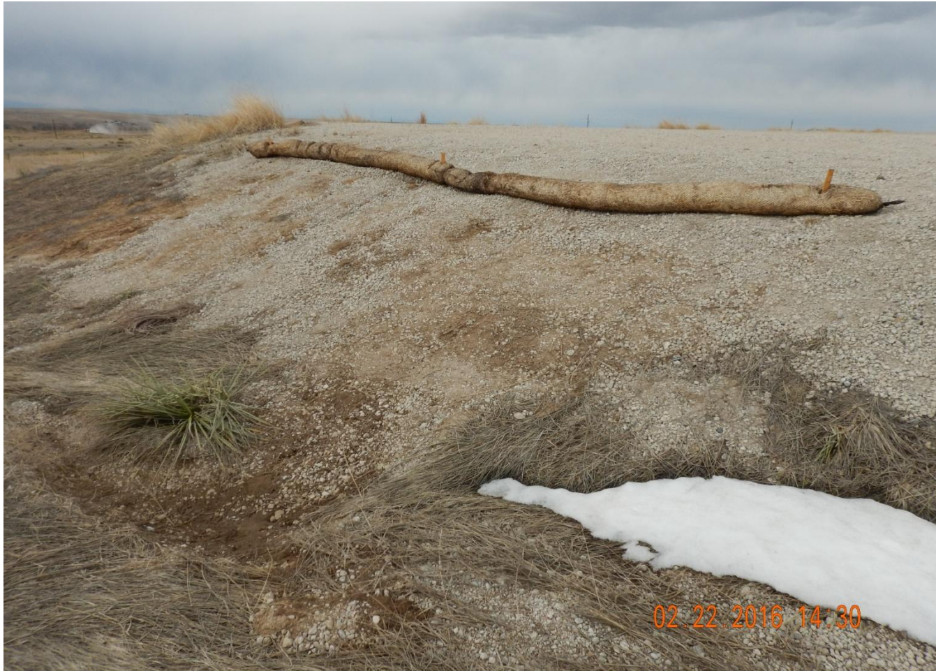
Photo 13. Photo taken from the southwest location, facing North. Wattle not properly installed. Gravel and sediment washing underneath wattle. Interim reclamation area needs to be reseeded and stabilized to minimize erosion while vegetative growth establishes.
