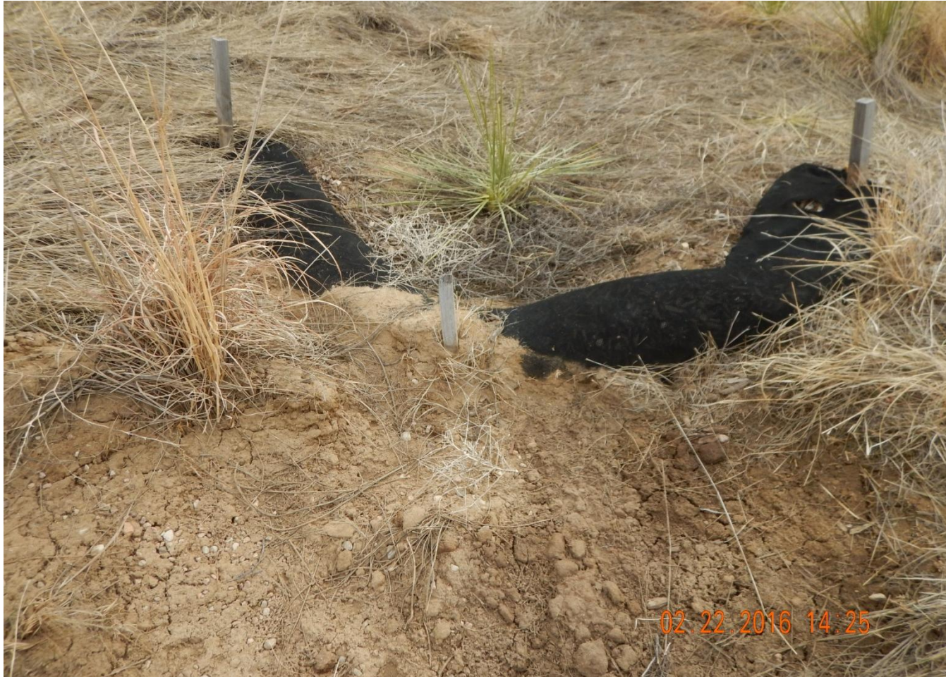
Photo 8. Photo taken from the western location, facing South. Stormwater and sediment BMPs need to be maintained to ensure controls are functioning properly.
