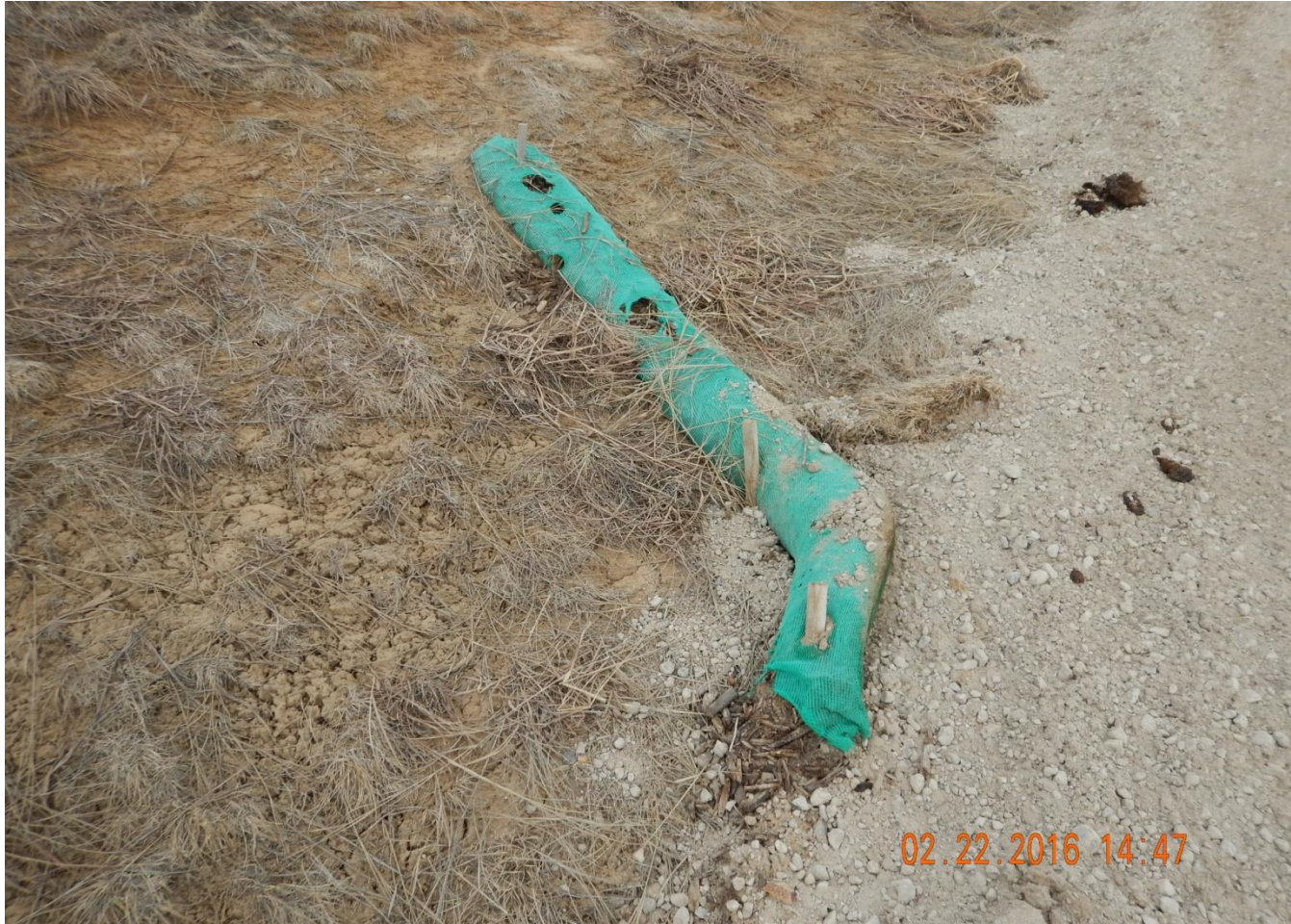
Photo 17. Photo taken from the entrance of the location, facing towards north wattle. Stormwater and sediment BMPs need to be maintained to controls are functioning properly. Wattle needs to be replaced.
