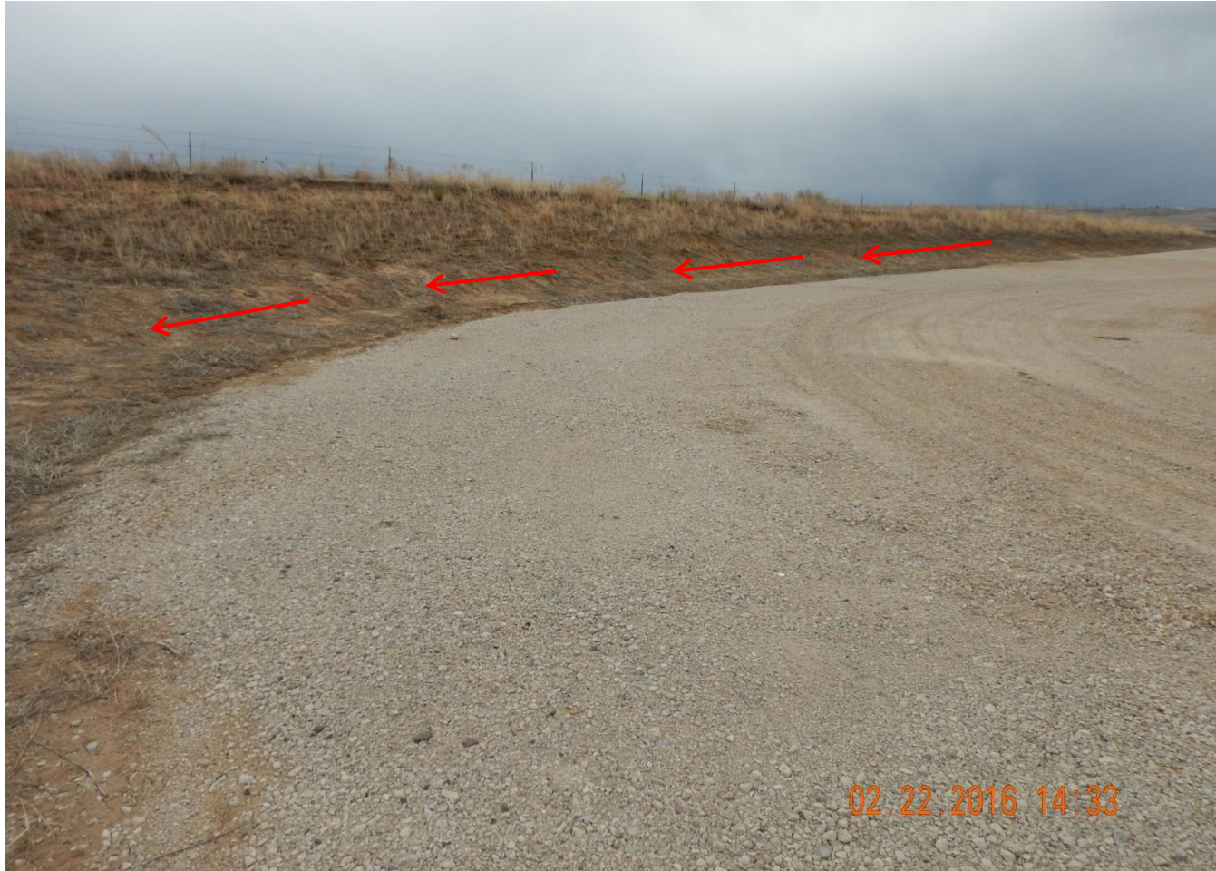
Photo 14. Photo taken from the southeast location, facing South. Cut slope needs to be stabilized with vegetation.
