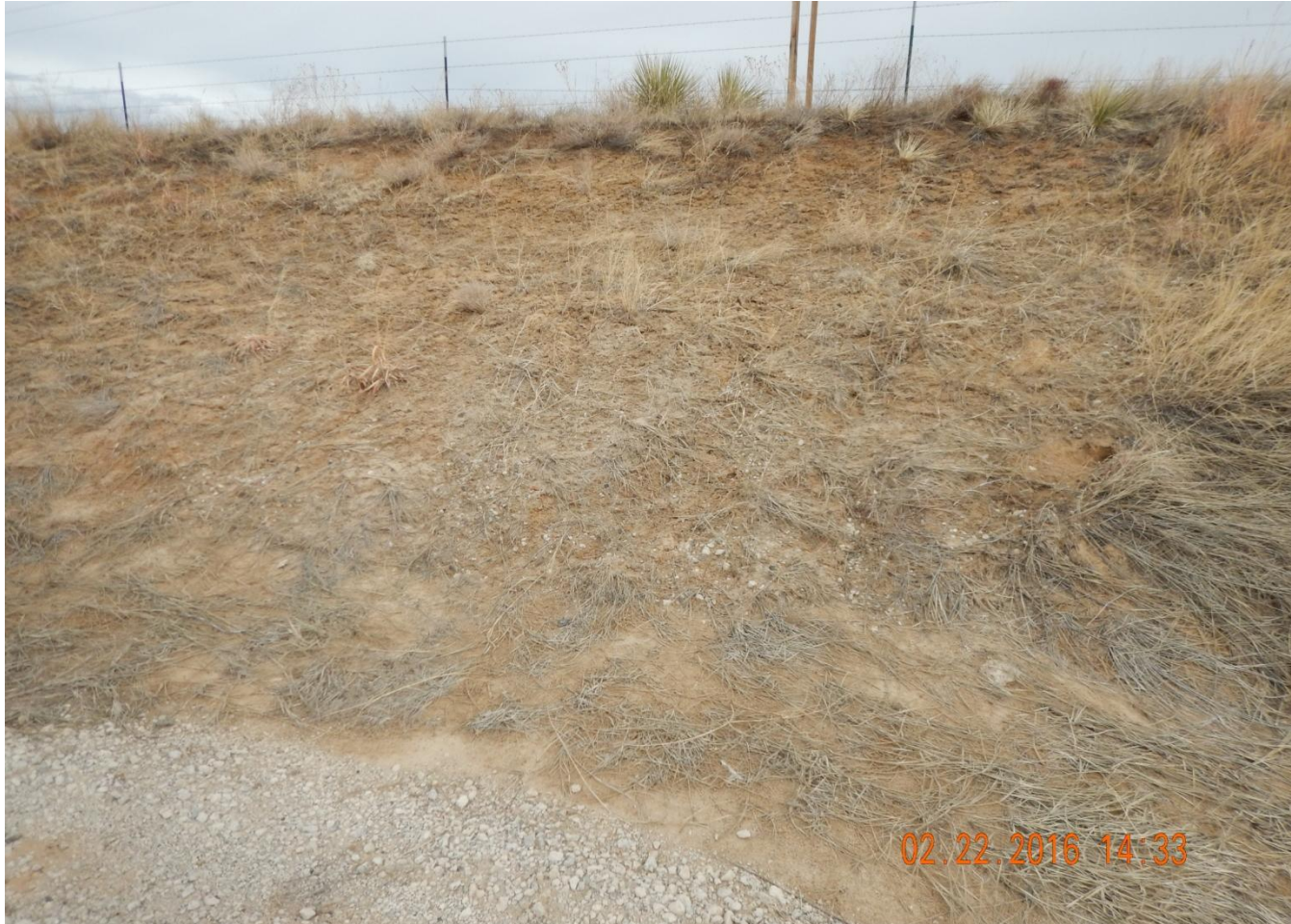
Photo 15. Photo taken from the southeast location, facing East. Cut slope needs to be stabilized with vegetation.
