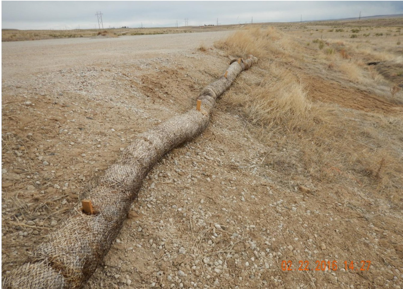
Photo 11. Photo taken from the western location, facing North. Wattle not properly installed. Gravel and sediment washing underneath wattle. Interim reclamation area needs to be reseeded and stabilized to minimize erosion while vegetative growth establishes.
