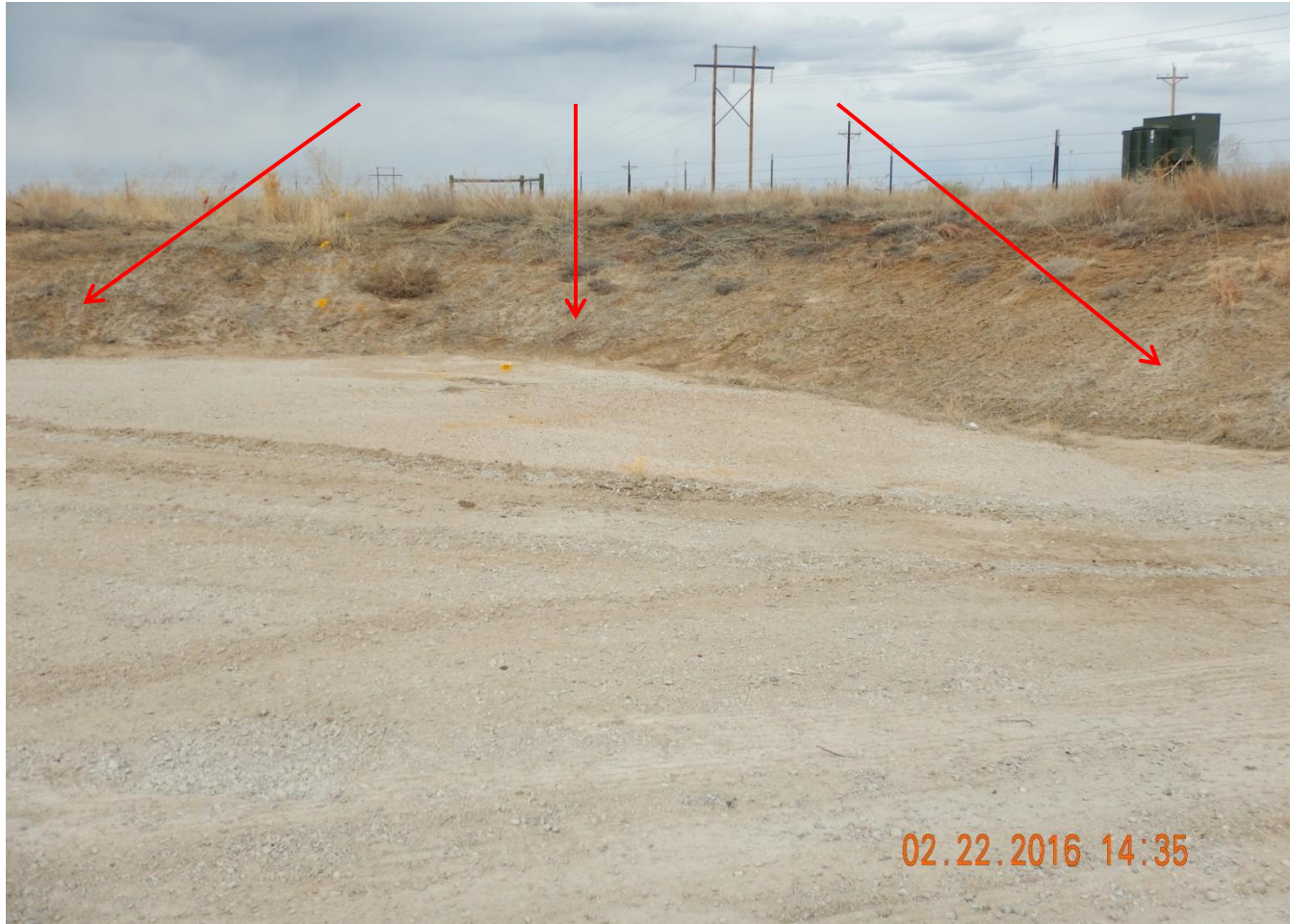
Photo 16. Photo taken from the southeast location, facing Northeast. Cut slope needs to be stabilized with vegetation.
