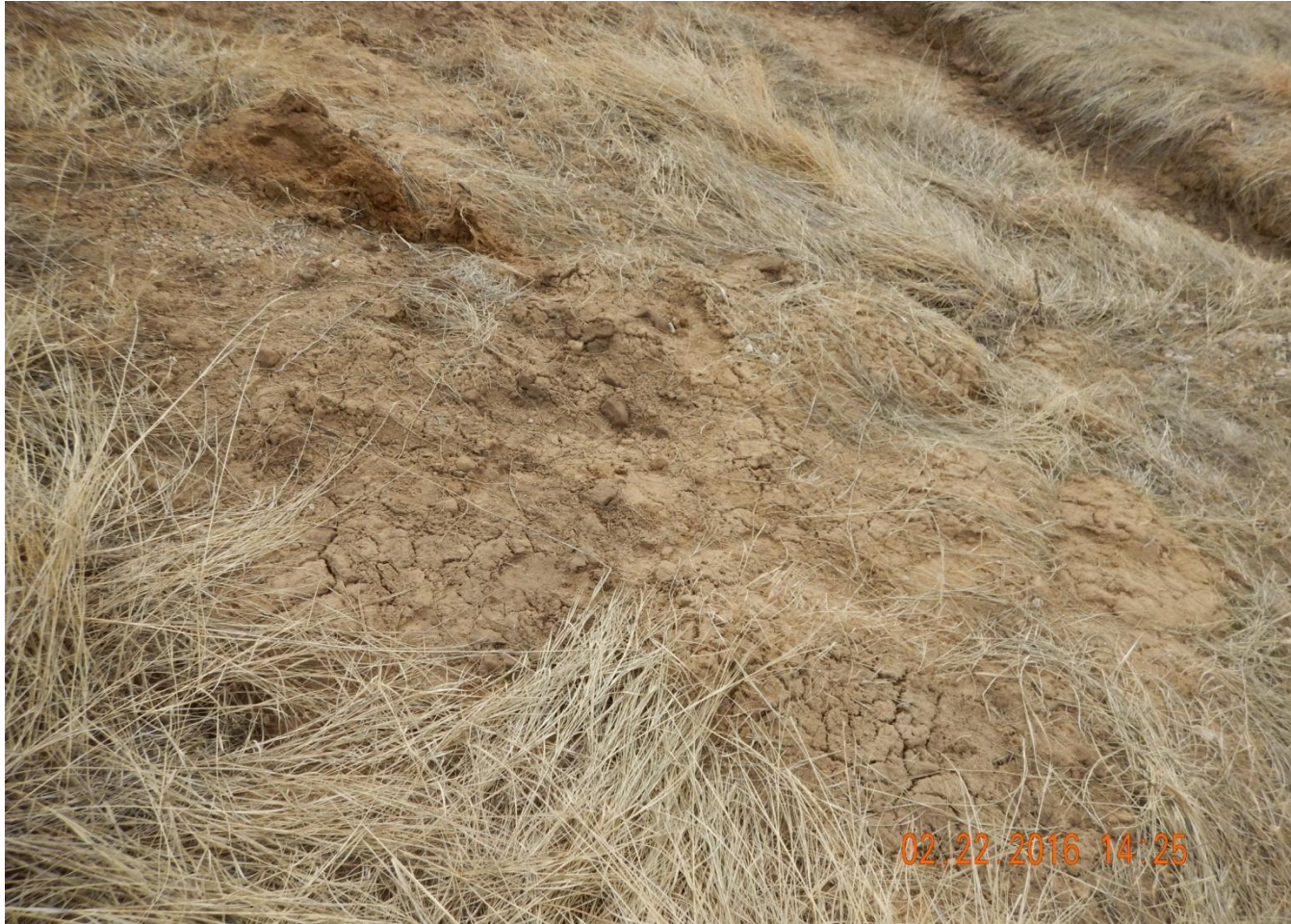
Photo 6. Photo taken from the western location, facing South. Interim reclamation area needs to be stabilized to minimize erosion while vegetative growth establishes. Erosion is occurring along portions of the western interim reclamation area.
