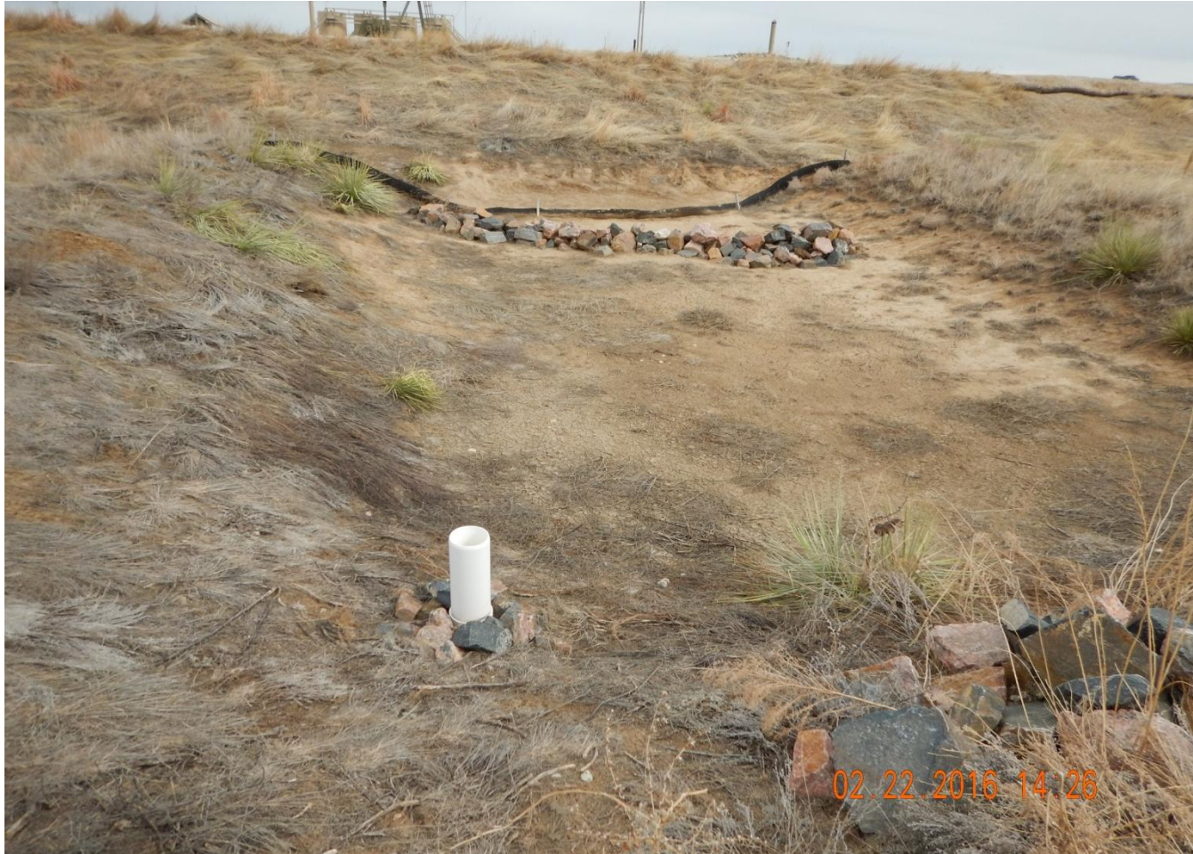
Photo 10. Photo taken from the western sediment trap location, facing East. Sediment trap was designed and installed correctly.
