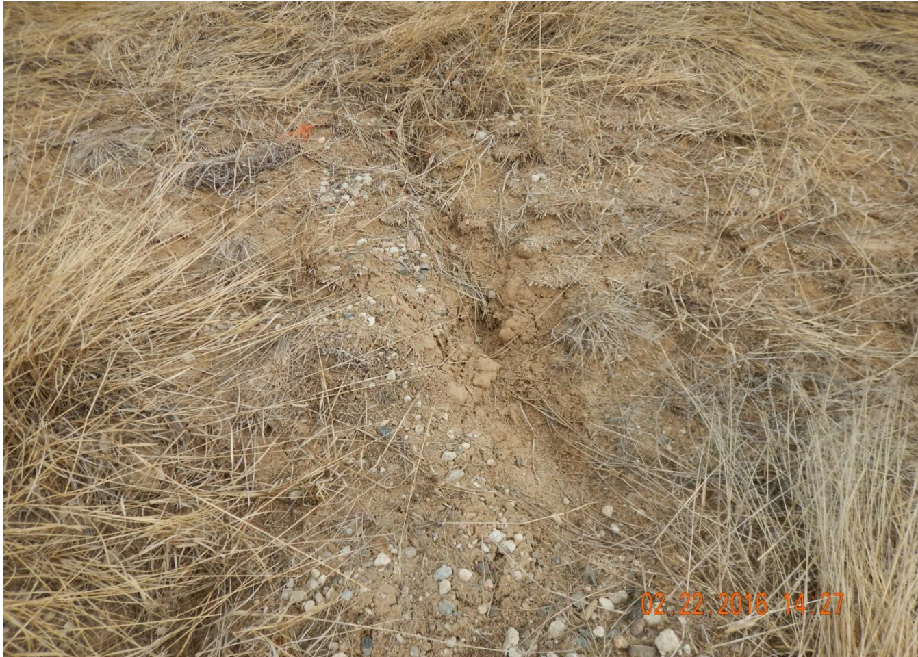
Photo 7. Photo taken from the western location, facing South. Interim reclamation area needs to be stabilized to minimize erosion while vegetative growth establishes. Erosion is occurring along portions of the western interim reclamation area.
