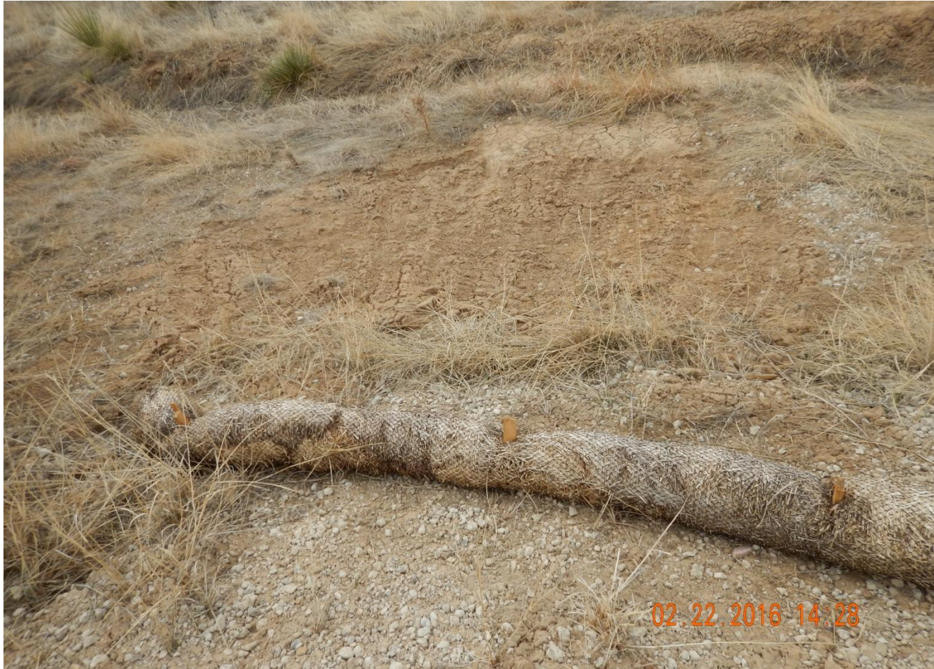
Photo 12. Photo taken from the western location, facing West. Wattle not properly installed. Gravel and sediment washing underneath wattle. Interim reclamation area needs to be stabilized to minimize erosion while vegetative growth establishes.
