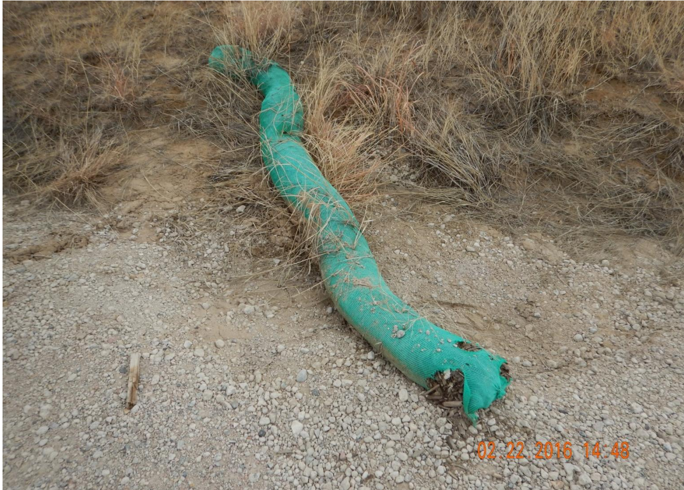
Photo 18. Photo taken from the entrance of the location, facing towards south wattle. Stormwater and sediment BMPs need to be maintained to ensure controls are functioning properly. Wattle needs to be replaced.
