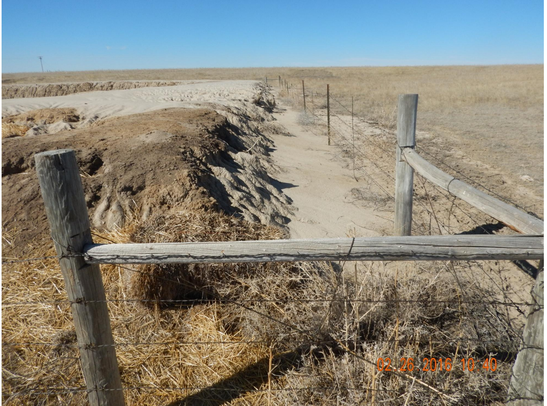
Figure 12: Photo taken from the northeast end of pit, facing west. Photo of erosion on pit, and hay bales used as a stormwater control. Note stormwater controls used are improperly installed and have not been maintained. Stormwater controls have not been installed on the northern end of the pit.
