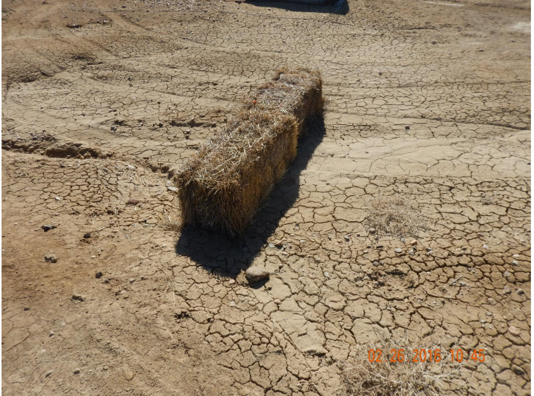
Figure 18: Photo taken from the east end of location. Photo of erosion on location, and hay bales used as a stormwater control method. Note stormwater controls used are improperly installed.
