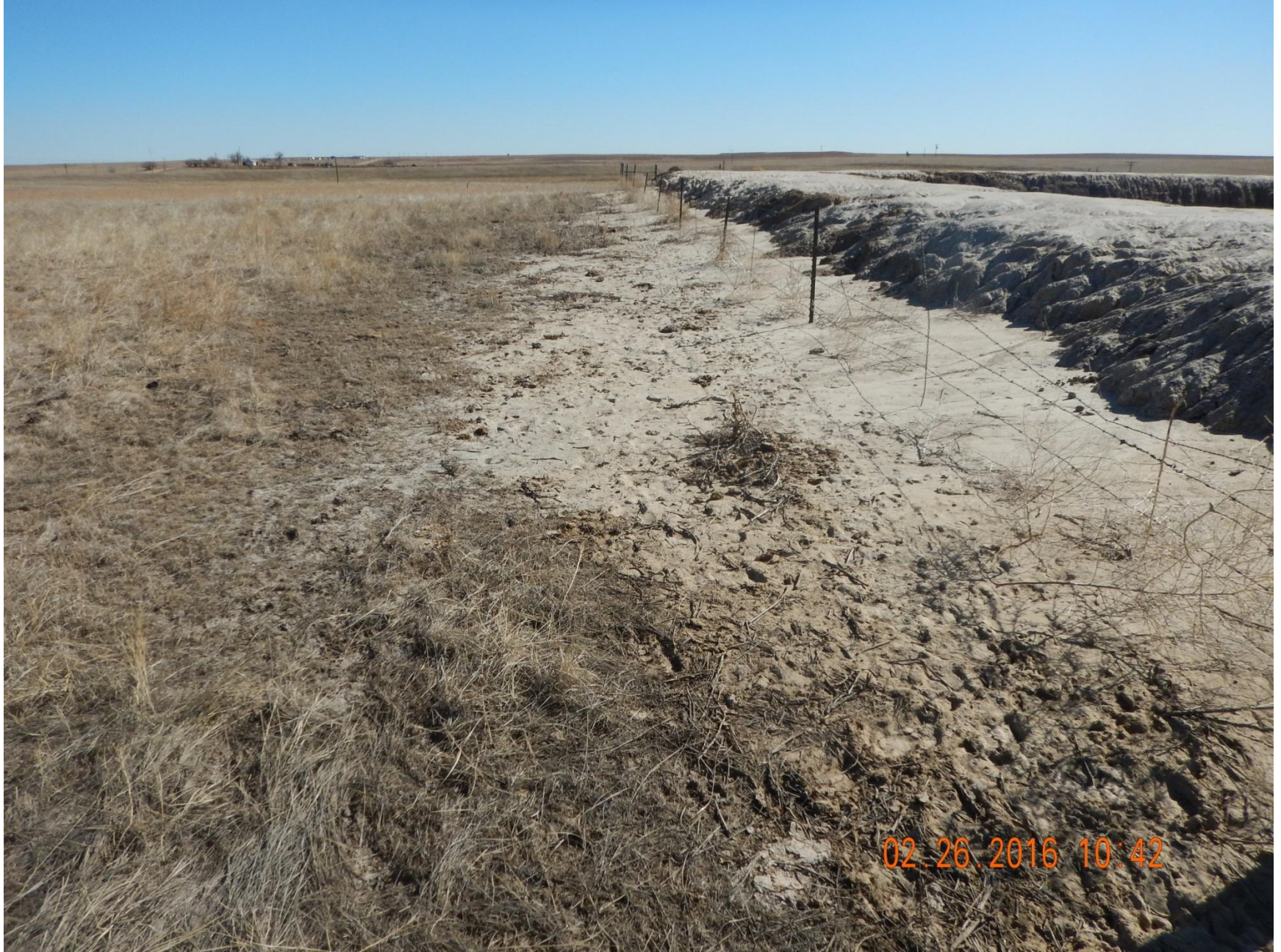
Figure 16: Photo taken from the northwest end of pit, facing west. Photo of erosion on pit. Note stormwater controls have not been installed on the northern end of the pit.
