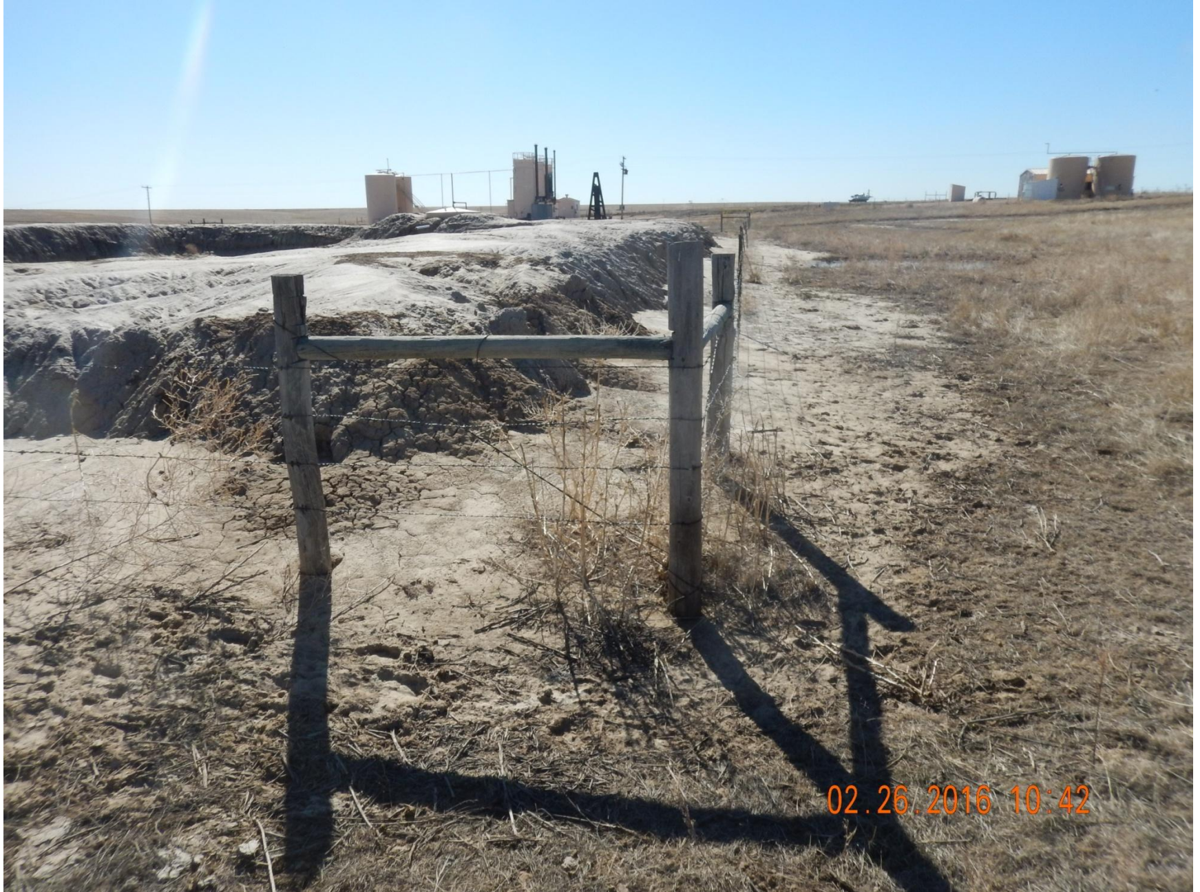
Figure 14: Photo taken from the northwest end of pit, facing south. Photo of erosion on pit. Note stormwater controls have not been installed on the northern and western end of the pit.
