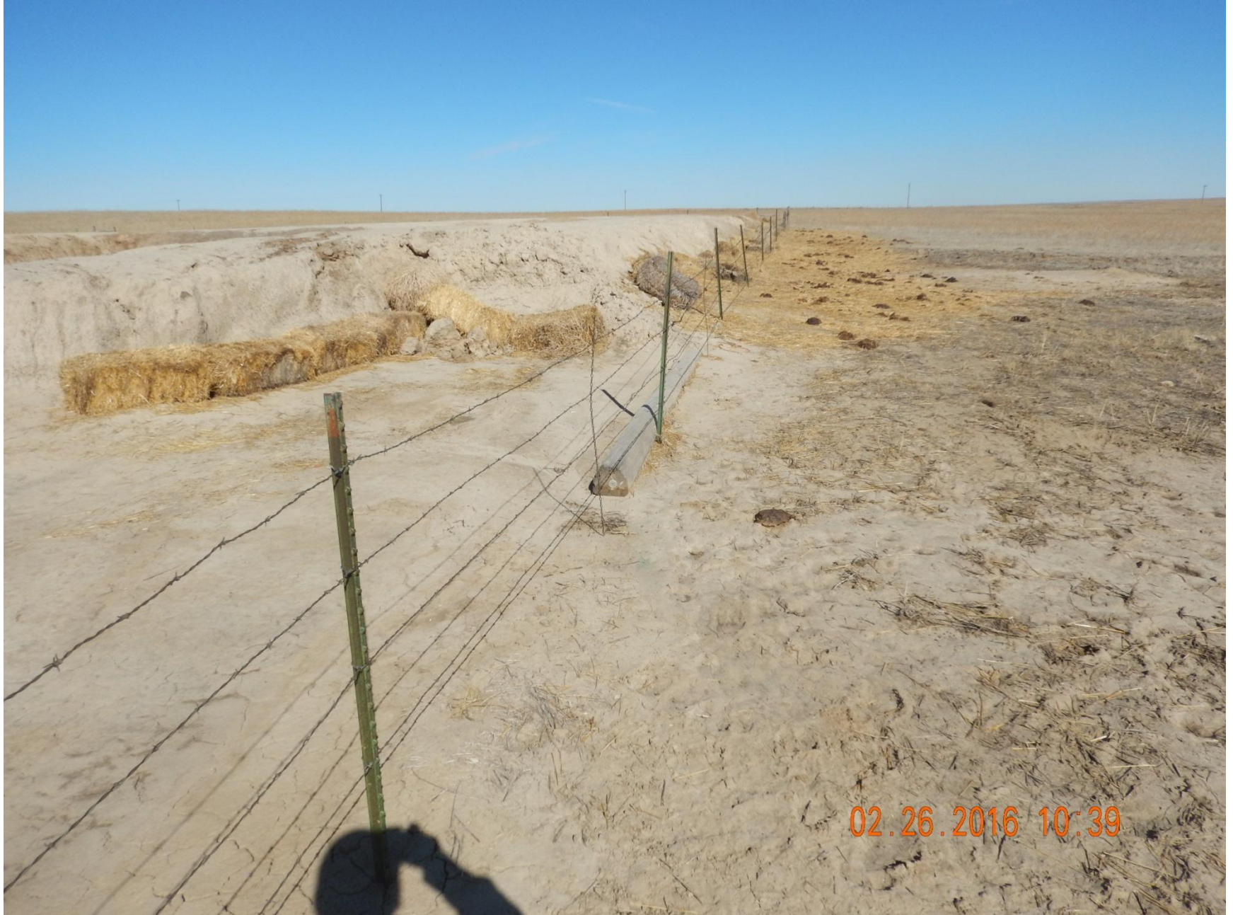
Figure 8: Photo taken from the southeast end of pit, facing northwest. Photo of erosion on pit, and hay bales used as a stormwater control. Note stormwater controls used are improperly installed and have not been maintained.
