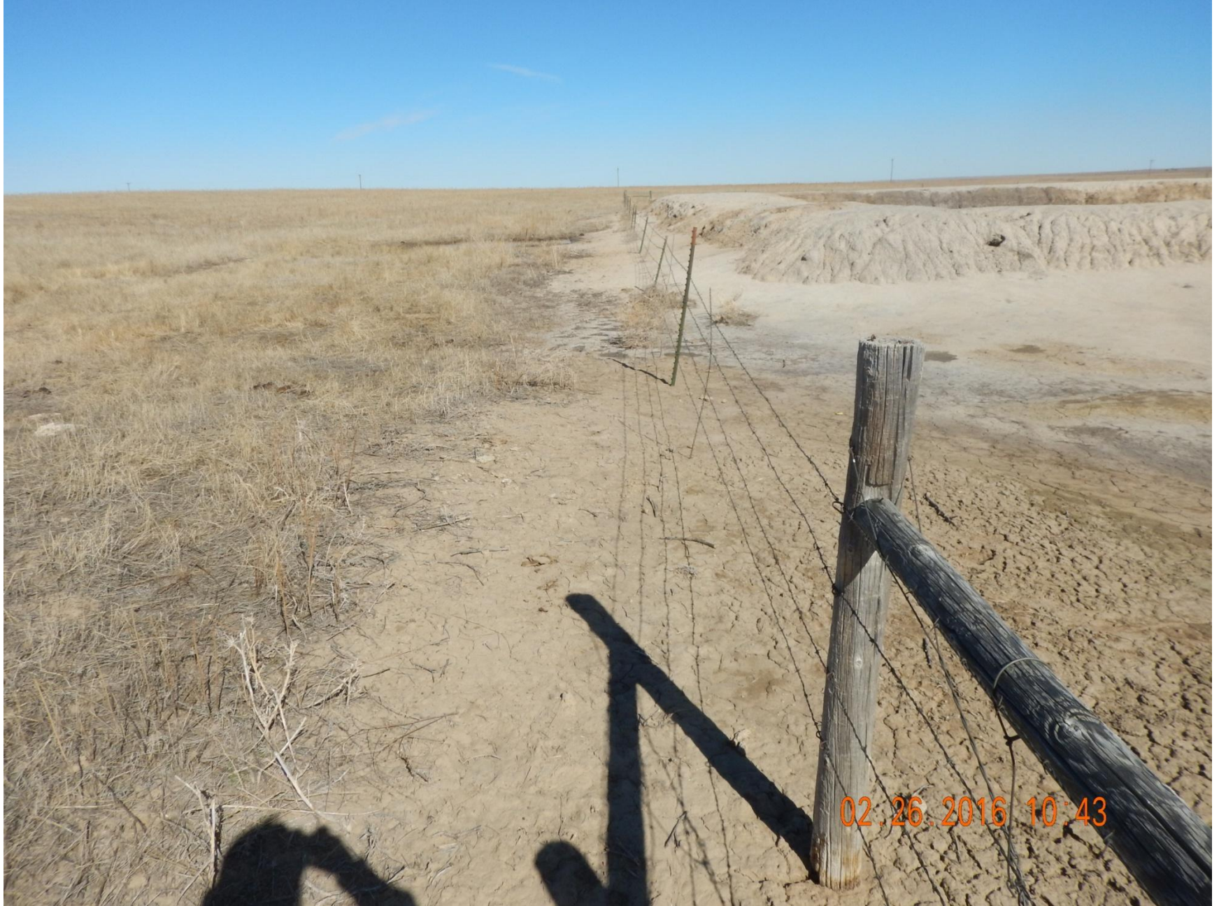
Figure 16: Photo taken from the southwest end of pit, facing north. Photo of erosion on pit. Note stormwater controls have not been installed on the western end of the pit.
