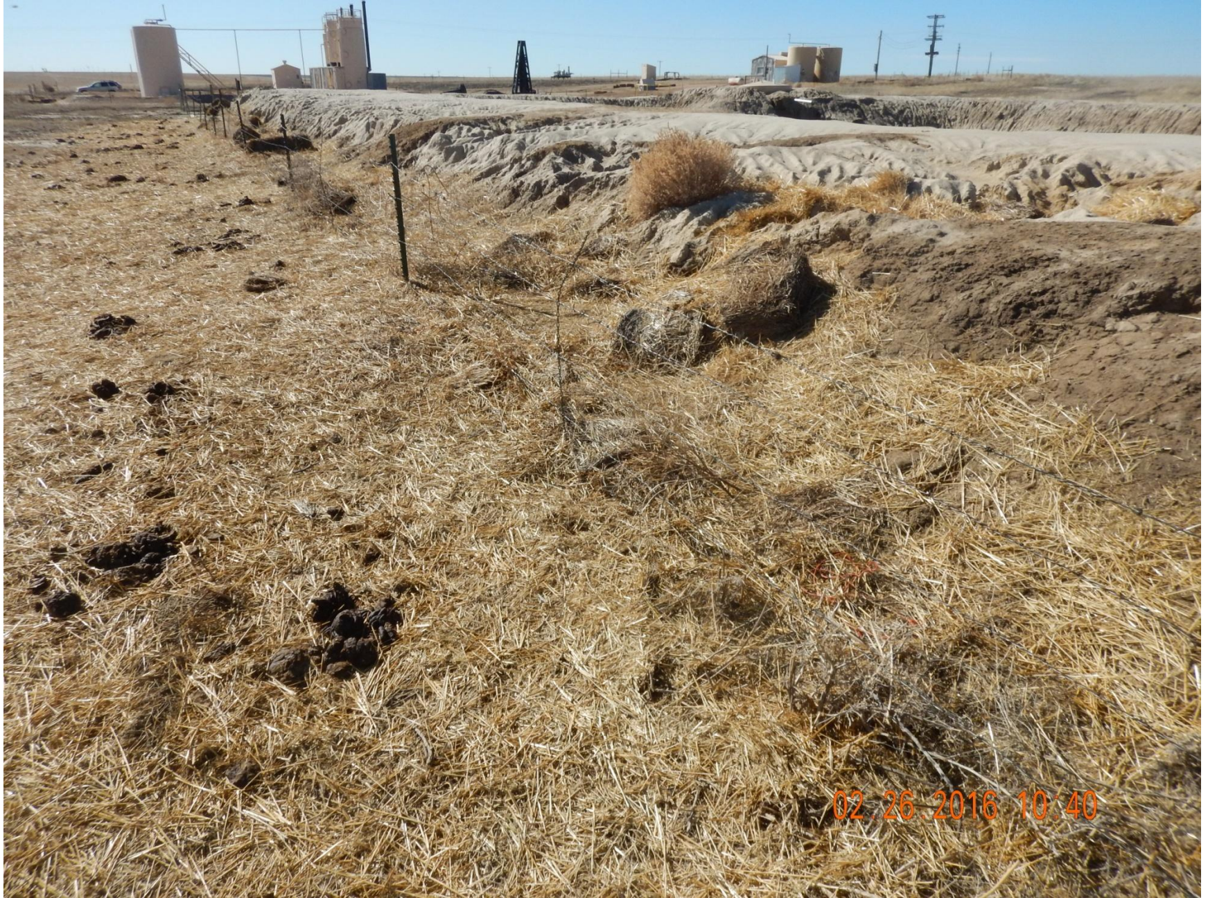
Figure 11: Photo taken from the northeast end of pit, facing south. Photo of erosion on pit, and hay bales used as a stormwater control. Note stormwater controls used are improperly installed and have not been maintained.
