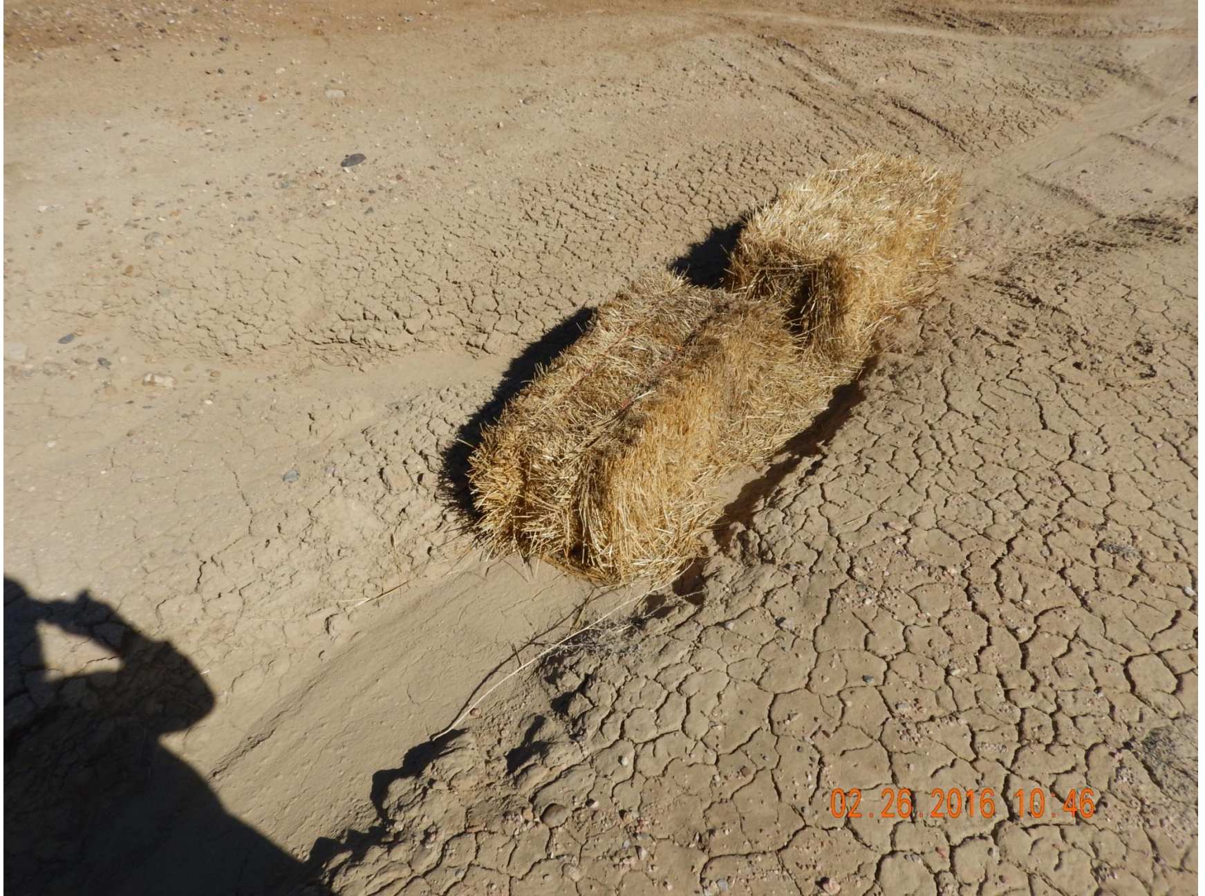
Figure 20: Photo taken from south end of location. Photo of erosion on location, and hay bales used as a stormwater control method. Note stormwater controls used are improperly installed .
