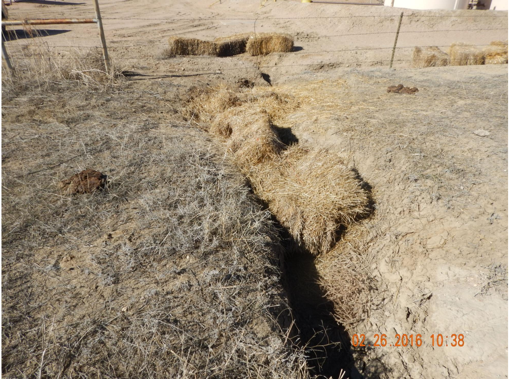
Figure 4: Photo taken east of location, facing west. Photo of gully forming off location and hay bales used as a stormwater control. Note that stormwater control method used for gully erosion is inadequate and unsatisfactory.
