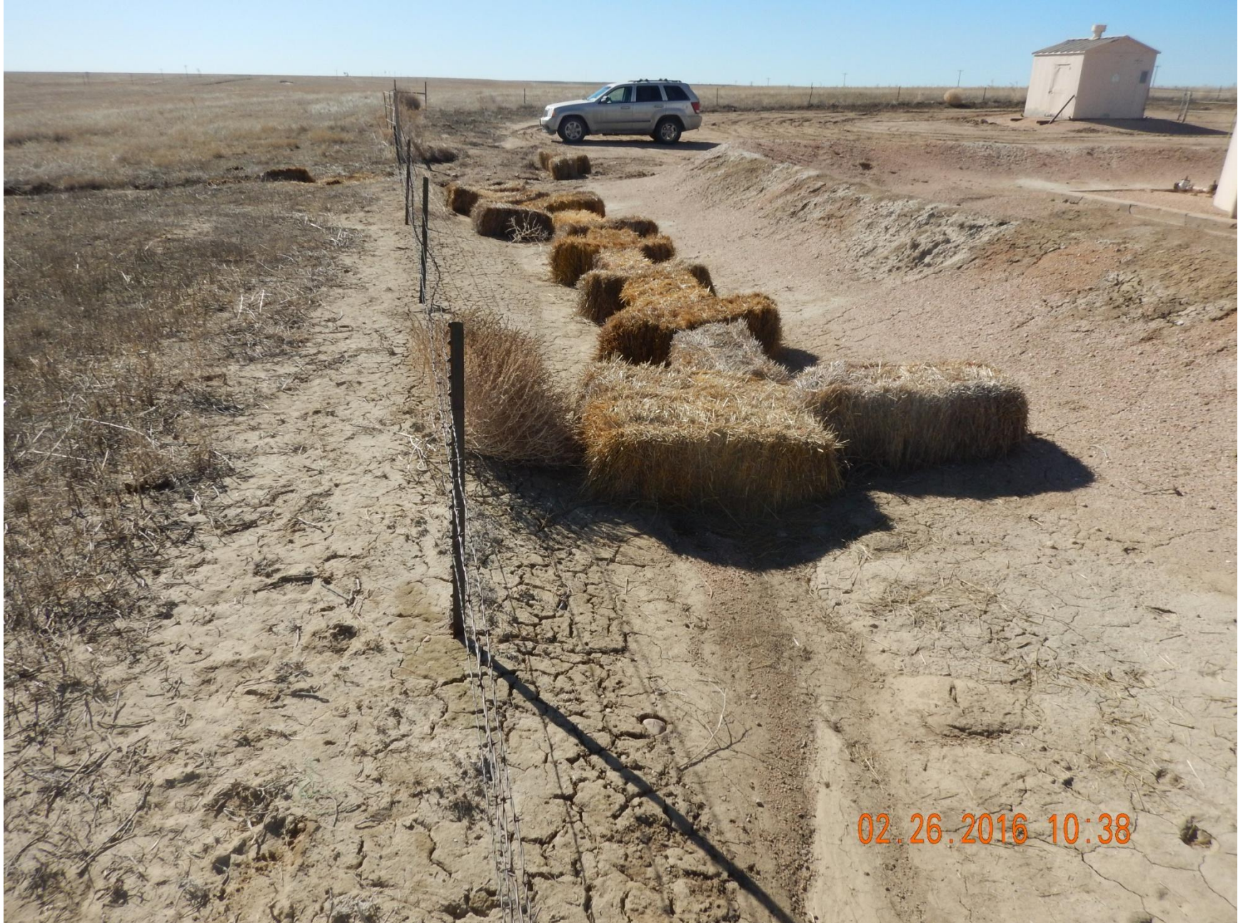
Figure 6: Photo taken from east end of location, facing south. Photo of erosion on location, and hay bales used as a stormwater control method. Note stormwater controls used are improperly installed.
