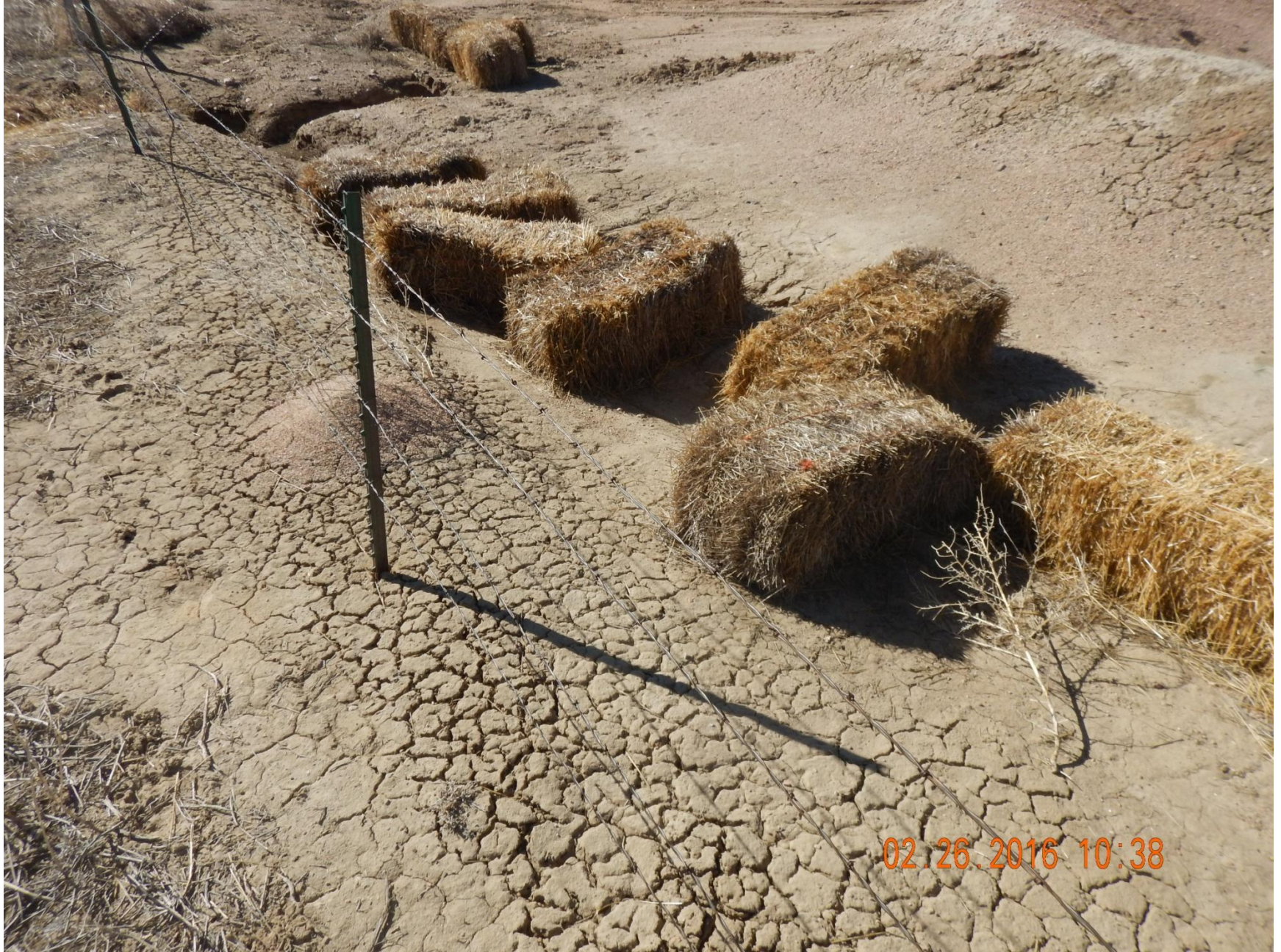
Figure 5: Photo taken from east end of location, facing southwest. Photo of erosion on location, and hay bales used as a stormwater control method. Note stormwater controls used are improperly installed.
