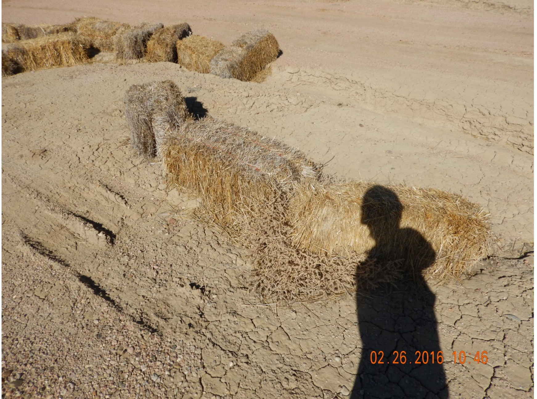
Figure 22: Photo taken from south end of location. Photo of erosion on location, and hay bales used as a stormwater control method. Note stormwater controls used are improperly installed.
