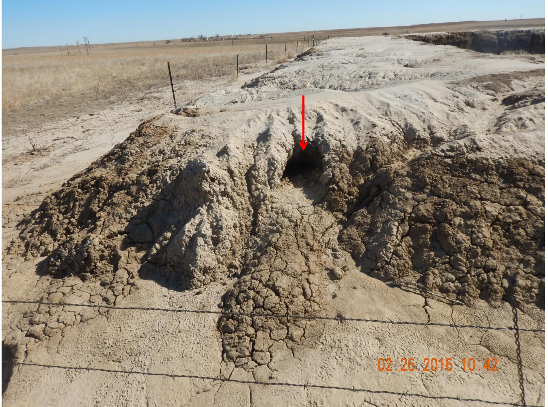
Figure 15: Photo taken from the northwest end of pit, facing east. Photo shows burrowing activities by wildlife taking place in pit wall.
