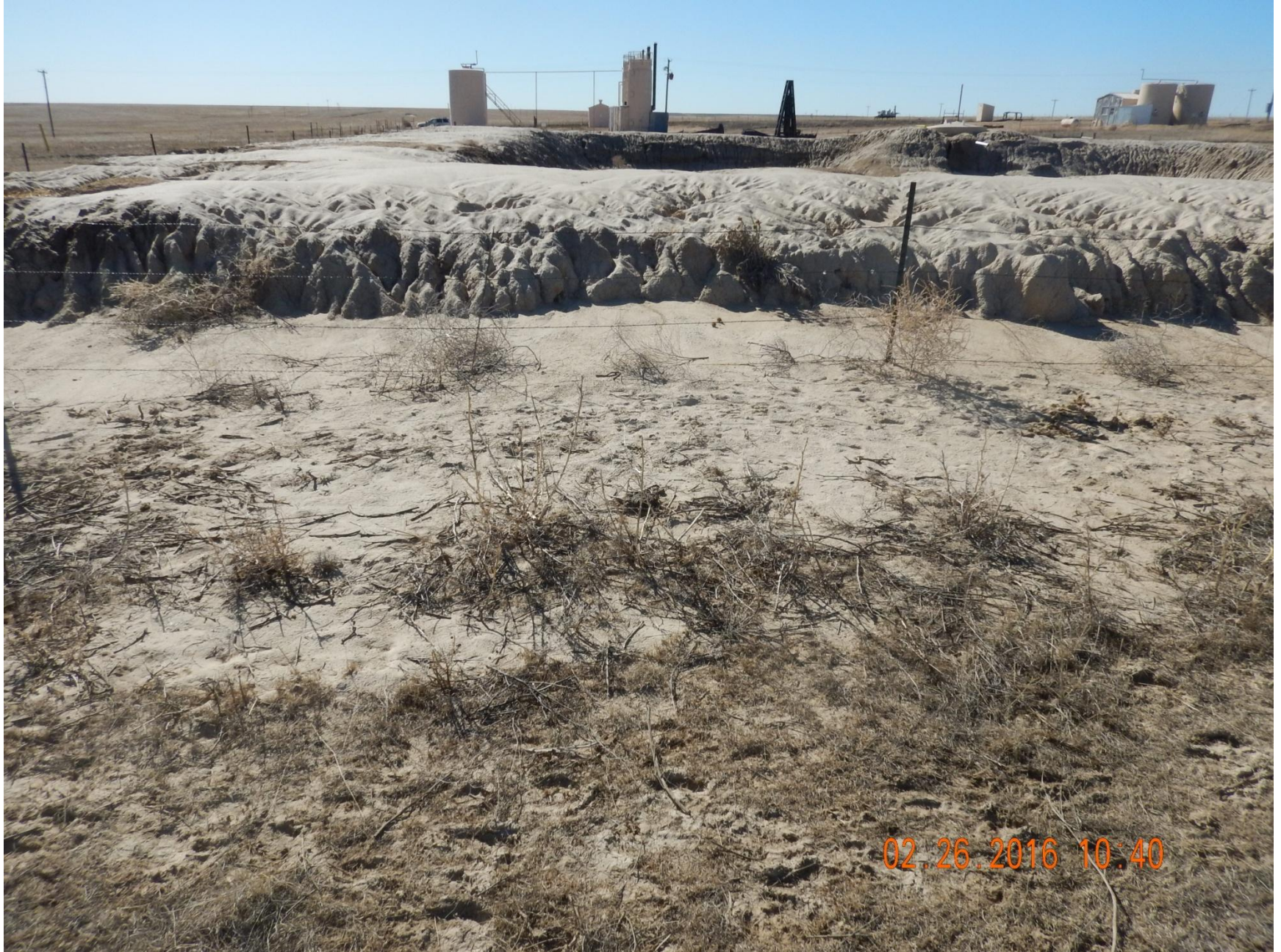
Figure 13: Photo taken from the north end of pit, facing south. Photo of erosion on pit. Note stormwater controls have not been installed on the northern end of the pit.
