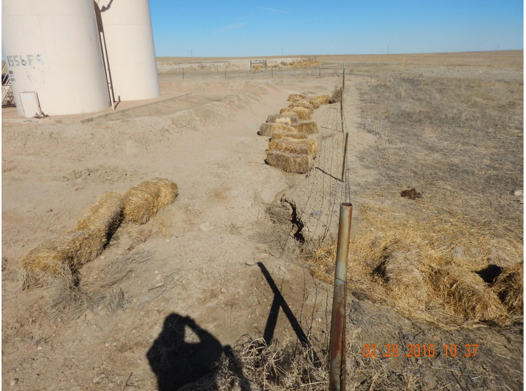
Figure 3: Photo taken from east end of location, facing north. Photo of gulley formation on and off location, and hay bales used as a stormwater control. Note stormwater controls used are inadequate and improperly installed.
