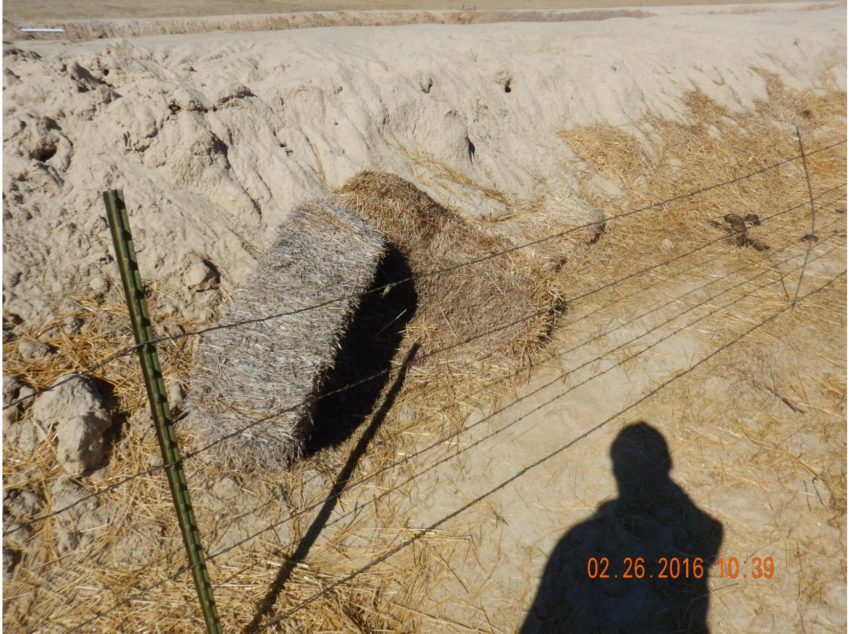
Figure 9: Photo taken from the southeast end of pit, facing northwest. Photo of erosion on pit, and hay bales used as a stormwater control. Note stormwater controls used are improperly installed and have not been maintained.
