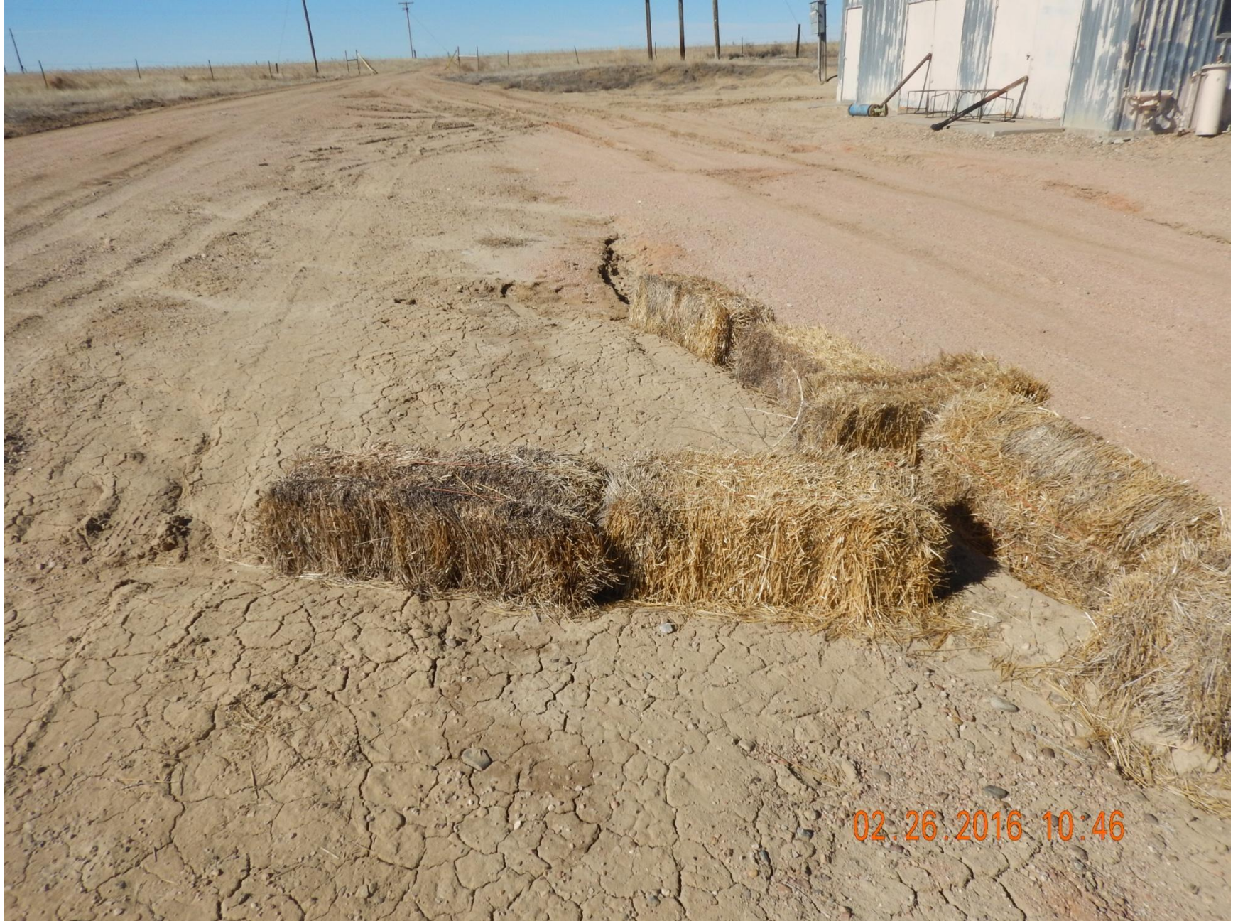
Figure 24: Photo taken from south end of location, facing west. Photo of erosion on location, and hay bales used as a stormwater control method. Note stormwater controls used are improperly installed.
