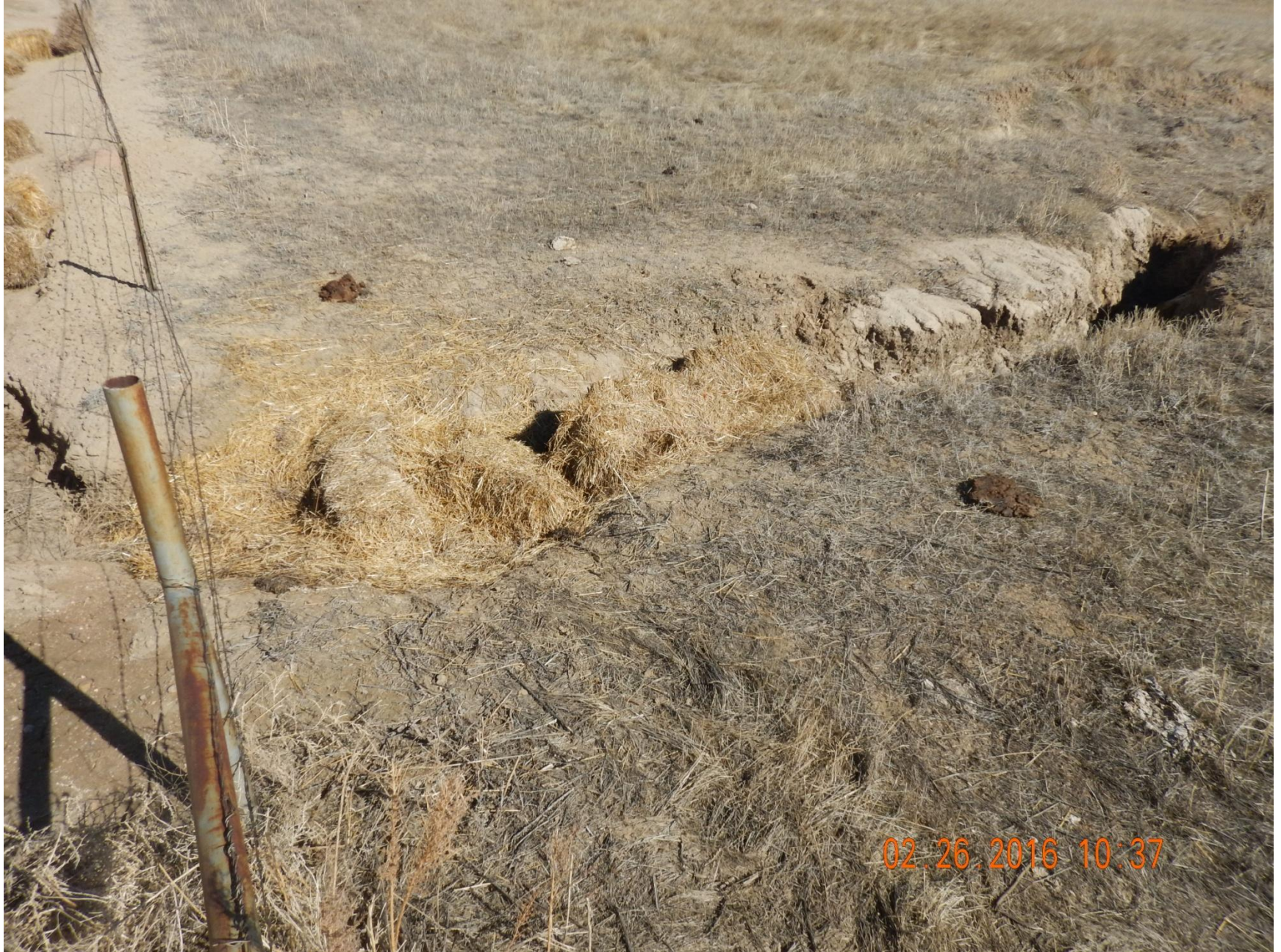
Figure 1: Photo taken from east end of location. Photo of gulley forming off location and hay bales used as a stormwater control method. Note that stormwater control method used for gulley erosion is inadequate and unsatisfactory.
