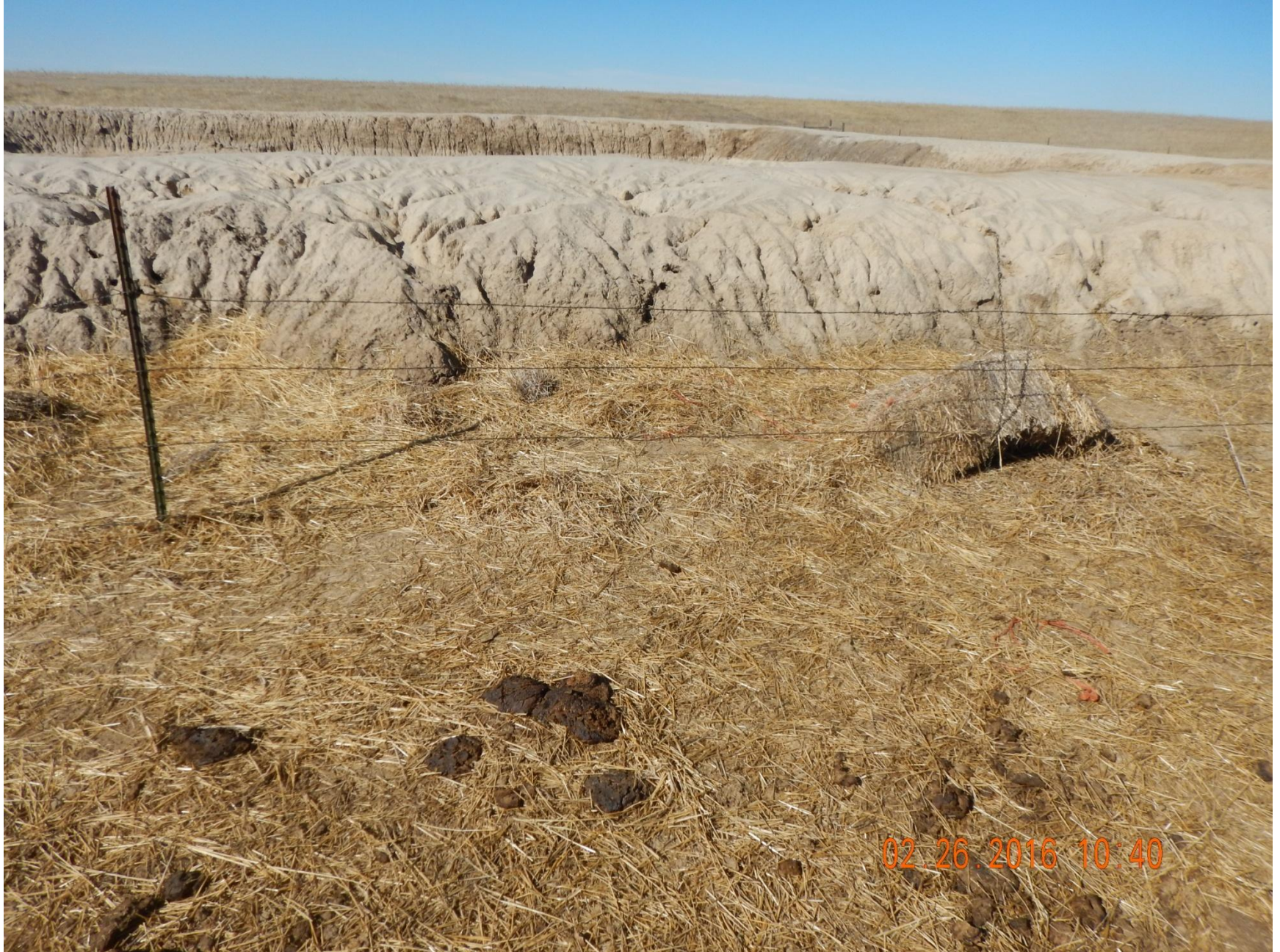
Figure 10: Photo taken from the east end of pit, facing west. Photo of erosion on pit, and hay bales used as a stormwater control. Note stormwater controls used are improperly installed and have not been maintained.
