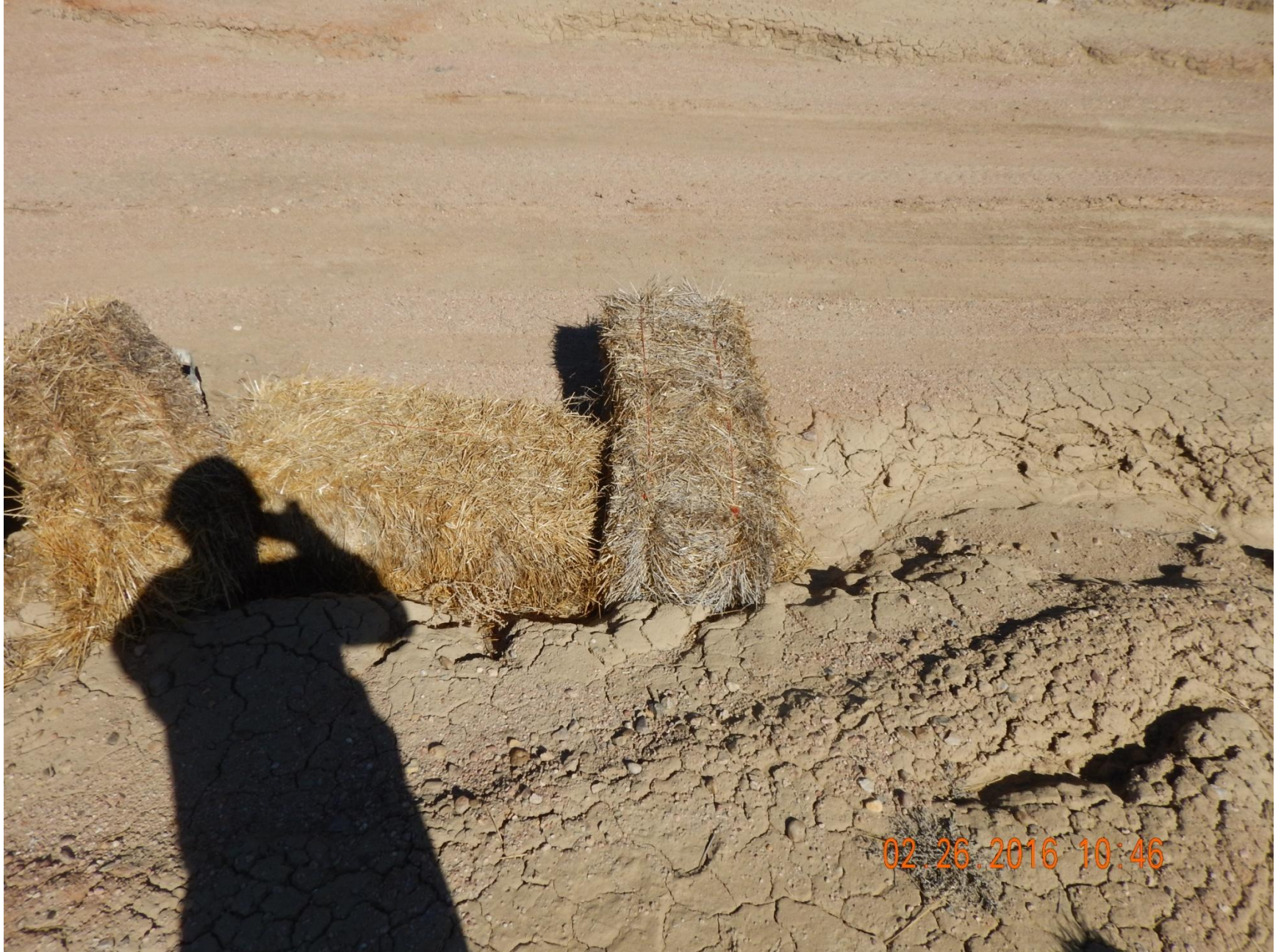
Figure 23: Photo taken from south end of location. Photo of erosion on location, and hay bales used as a stormwater control method. Note stormwater controls used are improperly installed.
