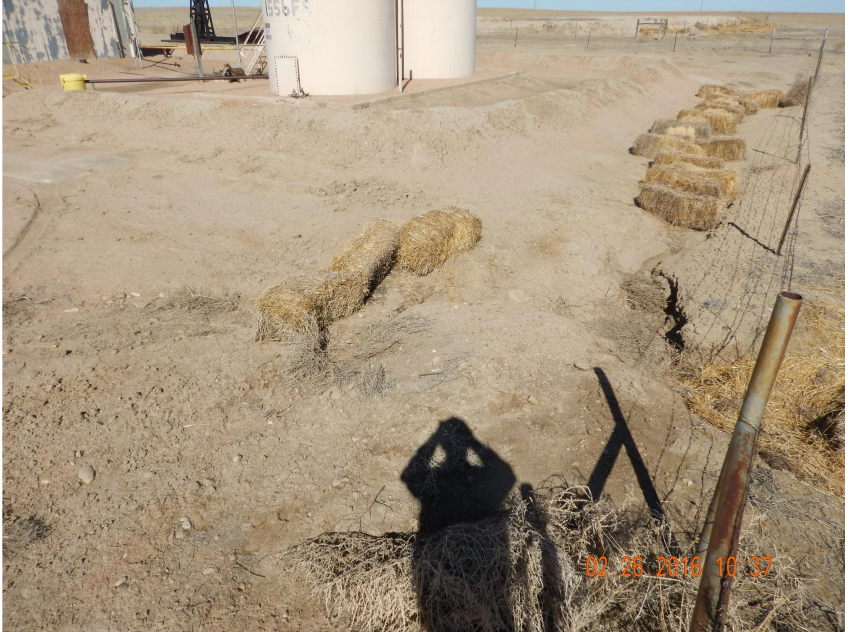
Figure 2: Photo taken from east end of location facing northwest. Photo of gully formation on location and hay bales used as a stormwater control. Note that stormwater control method used is inadequate and improperly installed.
