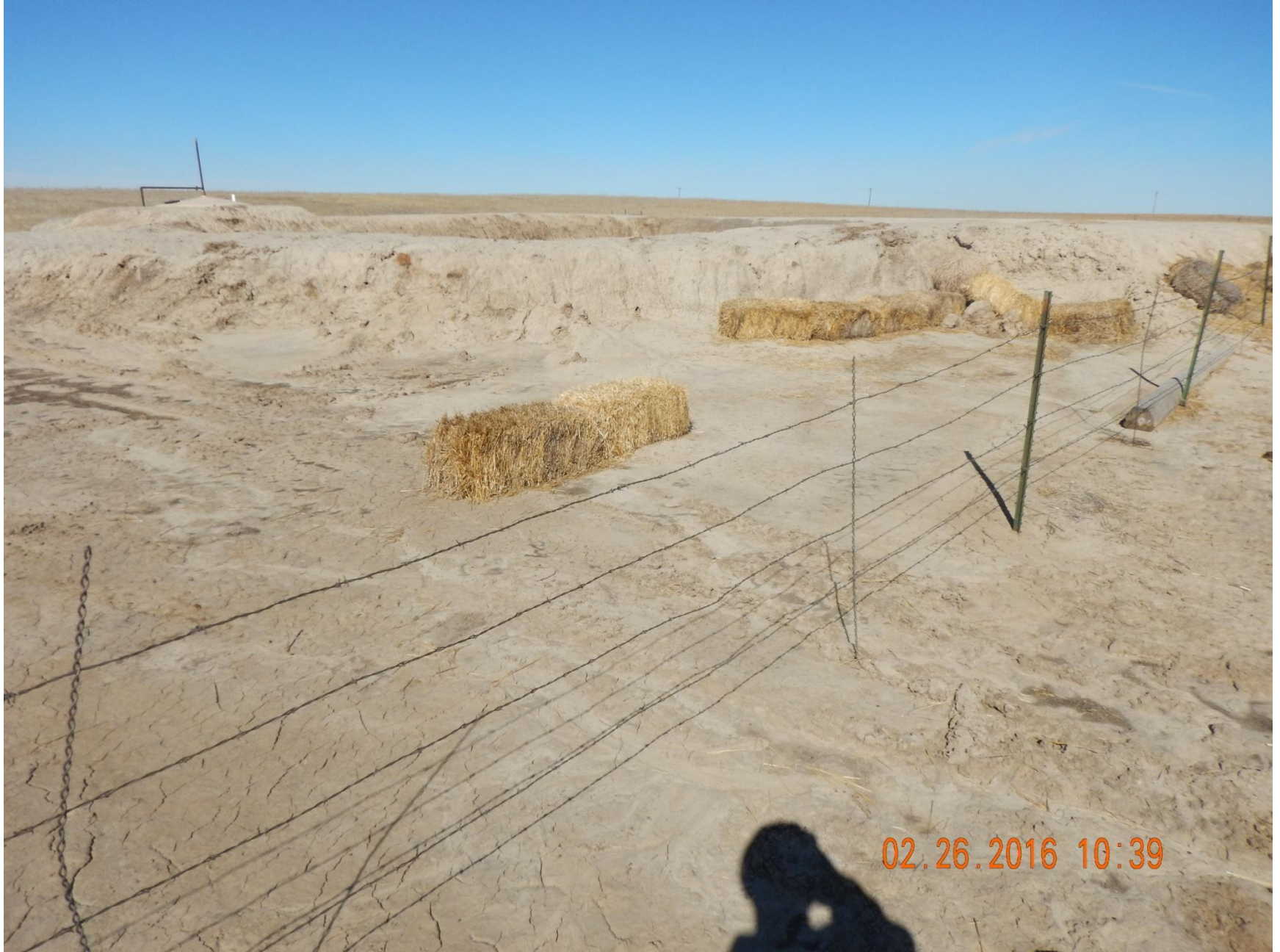
Figure 7: Photo taken from the southeast end of pit, facing northwest. Photo of erosion on pit, and hay bales used as a stormwater control. Note stormwater controls used are improperly installed.
