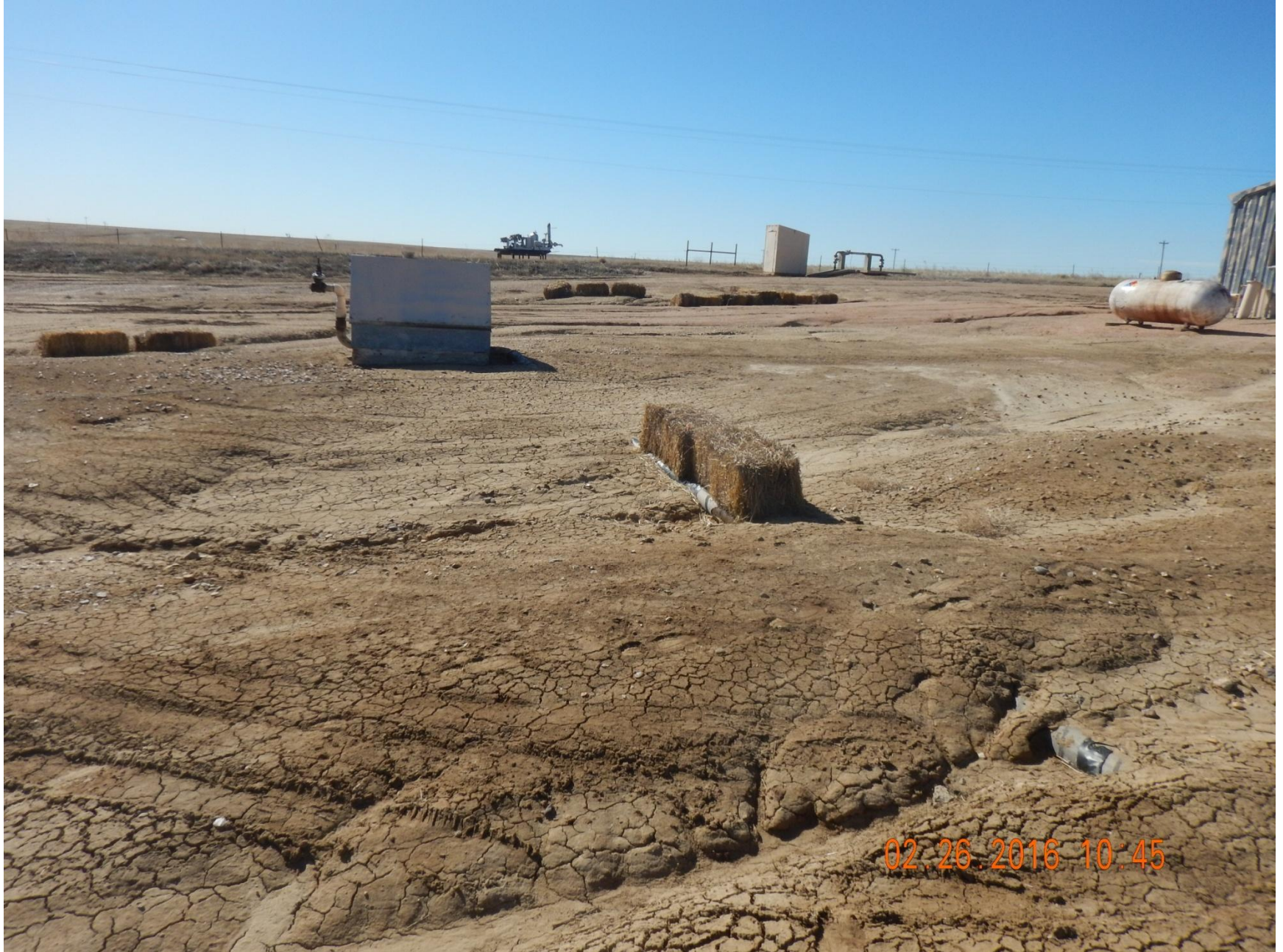
Figure 19: Photo taken from north end of location facing south. Photo of erosion on location, and hay bales used as a stormwater control method. Note stormwater controls used are improperly installed.
