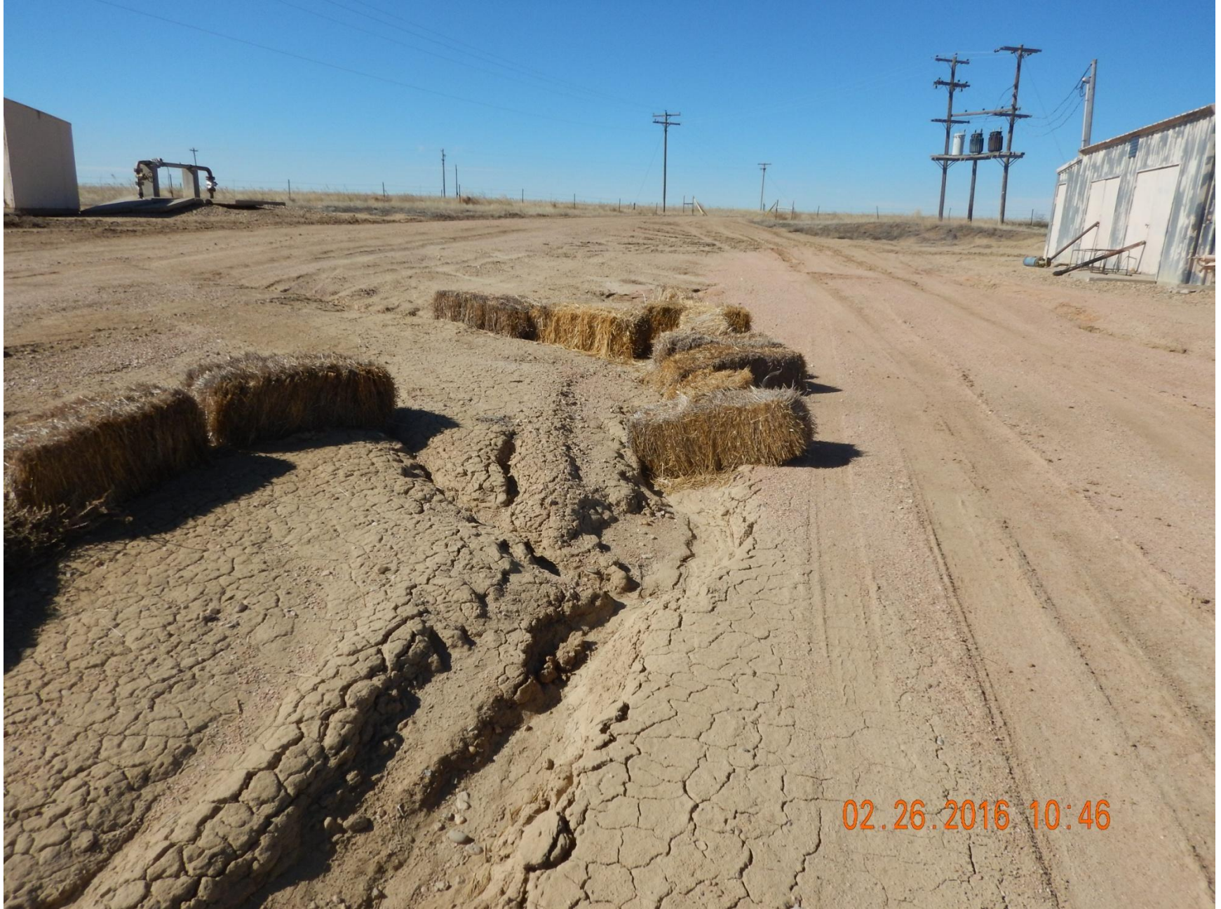
Figure 21: Photo taken from south end of location, facing west. Photo of erosion on location, and hay bales used as a stormwater control method. Note stormwater controls used are improperly installed.
