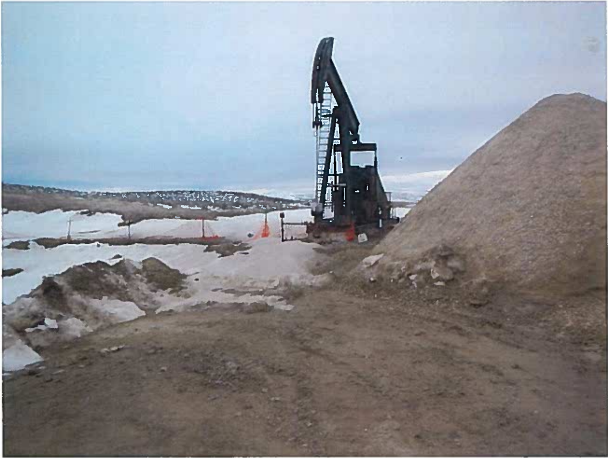
Picture taken looking South: pit is snow covered. Pad slopes into pit. Fencing around pit is not continuous, Storage of E&P waste is not per rule 907.
