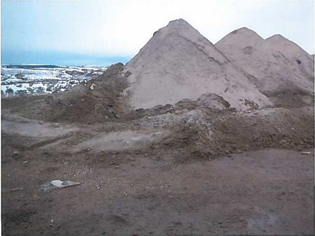
Picture taken looking West: E&P waste containment observed to be inadequate, E&P waste should be maintained per Rule 907.
