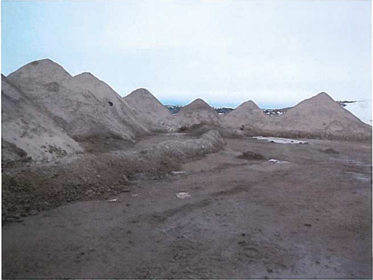
Picture taken looking North: E&P waste containment observed to be inadequate, E&P waste should be maintained per Rule 907.
