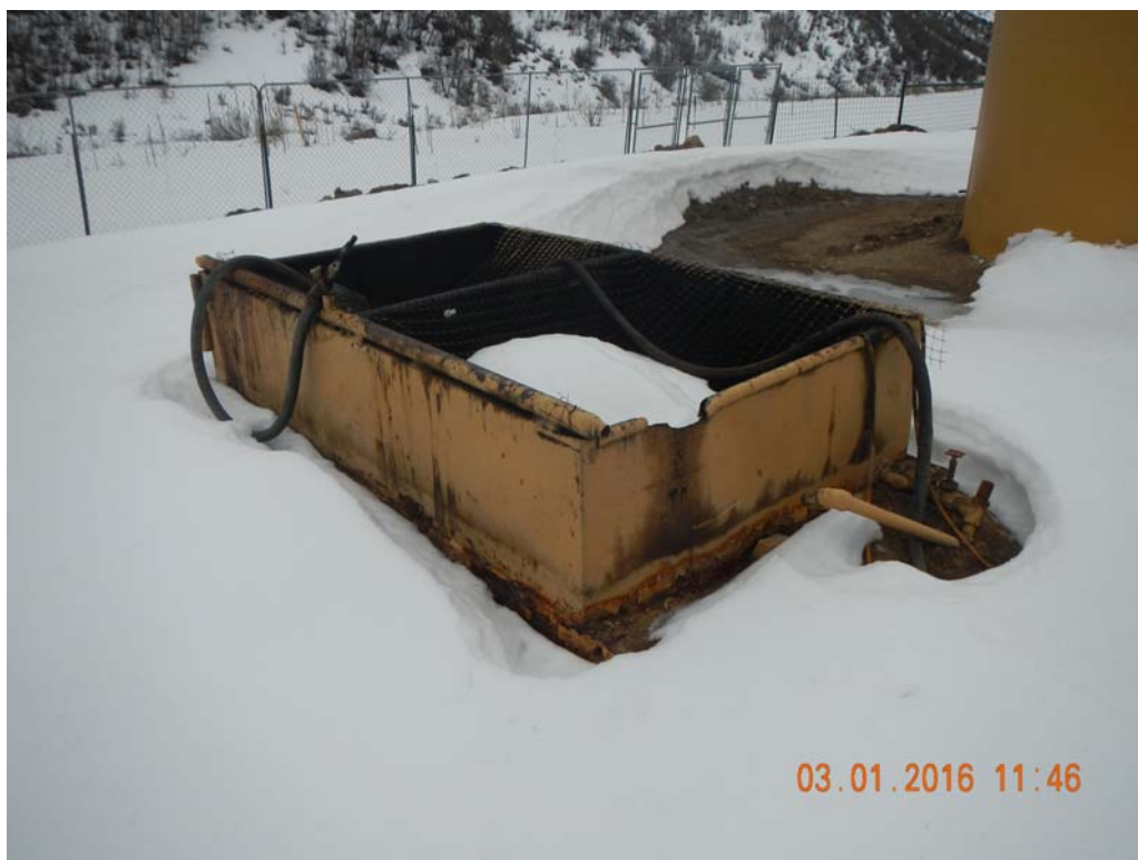
Open top tank with sagging netting and oily contents.
