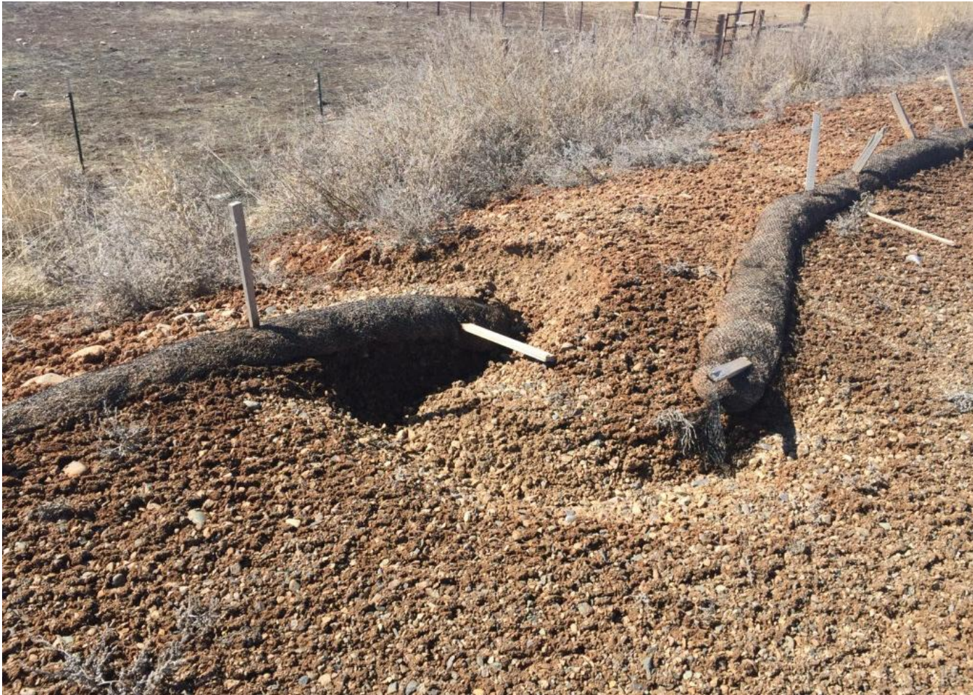
Photo 7. View of stormwater erosion that is occurring in the southern portion of the project area. Wattles need to be repaired and new BMPs may need to be installed.
