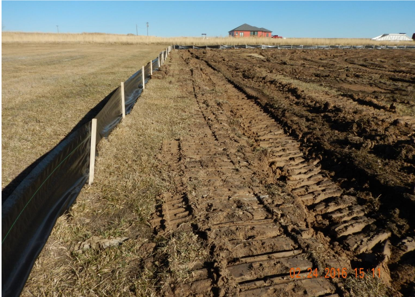
Photo 4. Photo taken from north-central location, facing East. Stormwater and sediment control BMPs installed in center of photo.
