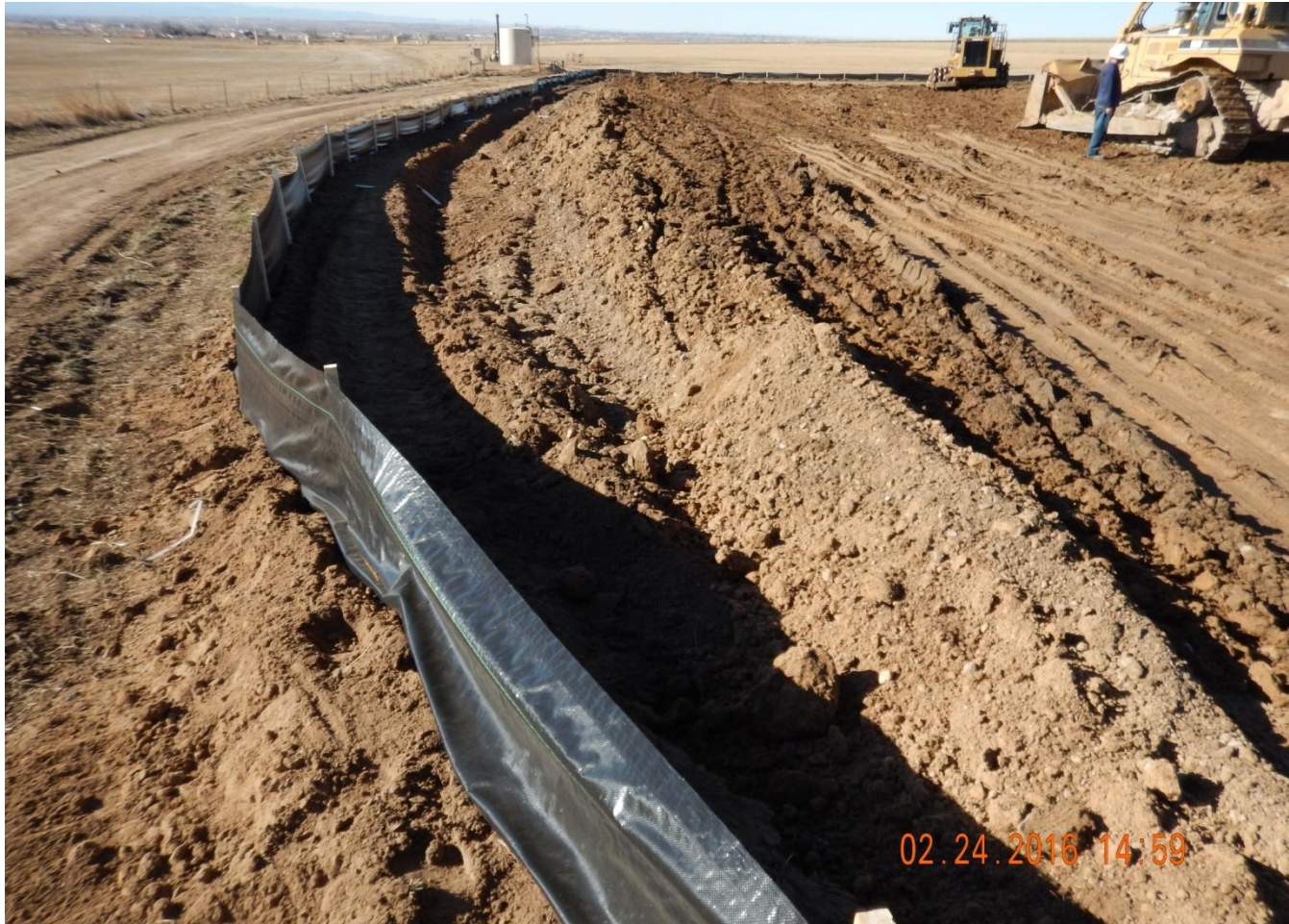
Photo 1. Photo taken from southwest location, facing North. Stormwater and sediment control BMPs installed in center of photo.
