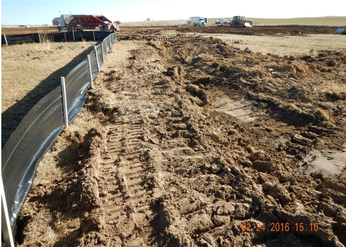
Photo 3. Photo taken from north-central location, facing South. Stormwater and sediment control BMPs installed in center of photo.
