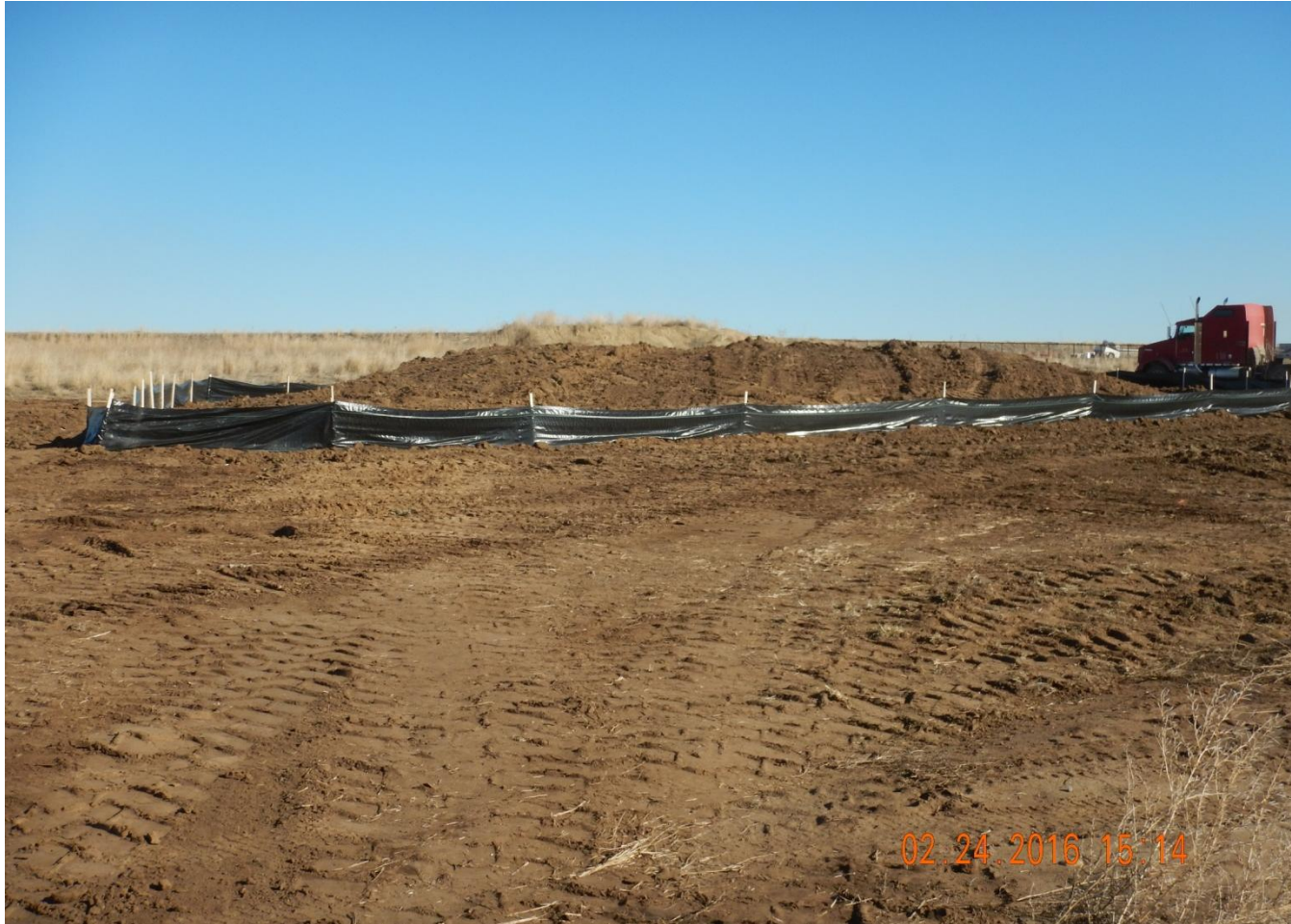
Photo 7. Photo taken from south of well location, facing East. Topsoil stockpile moved south of well location about 30 meters. Sediment control BMPs installed around topsoil stockpile.
