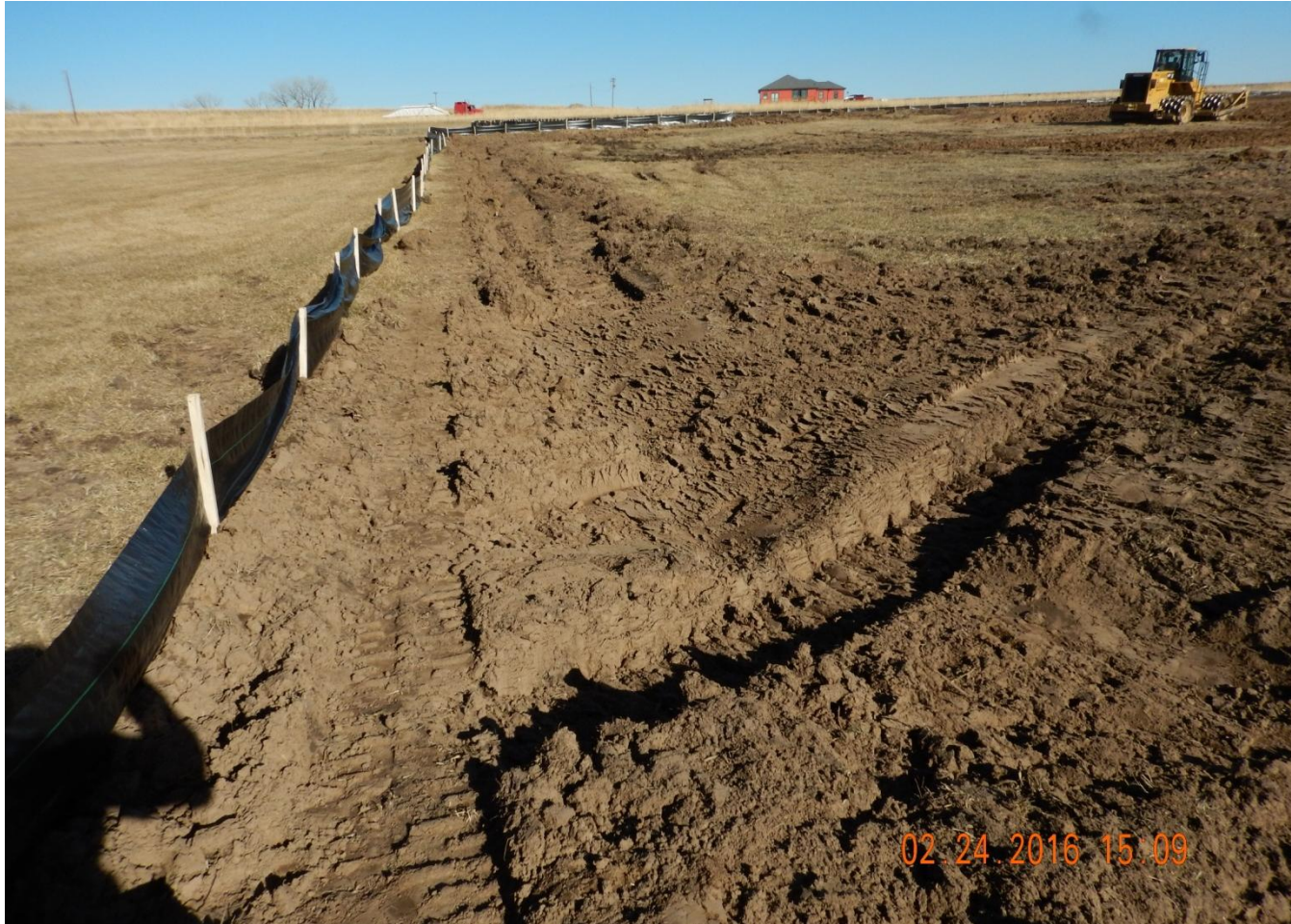
Photo 2. Photo taken from northwest location, facing East. Stormwater and sediment control BMPs installed in center of photo.
