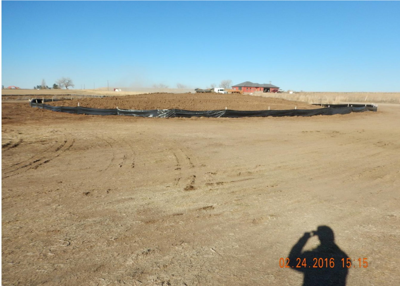
Photo 8. Photo taken from south of well location, facing North. Topsoil stockpile moved south of well location about 30 meters. Sediment control BMPs installed around topsoil stockpile.
