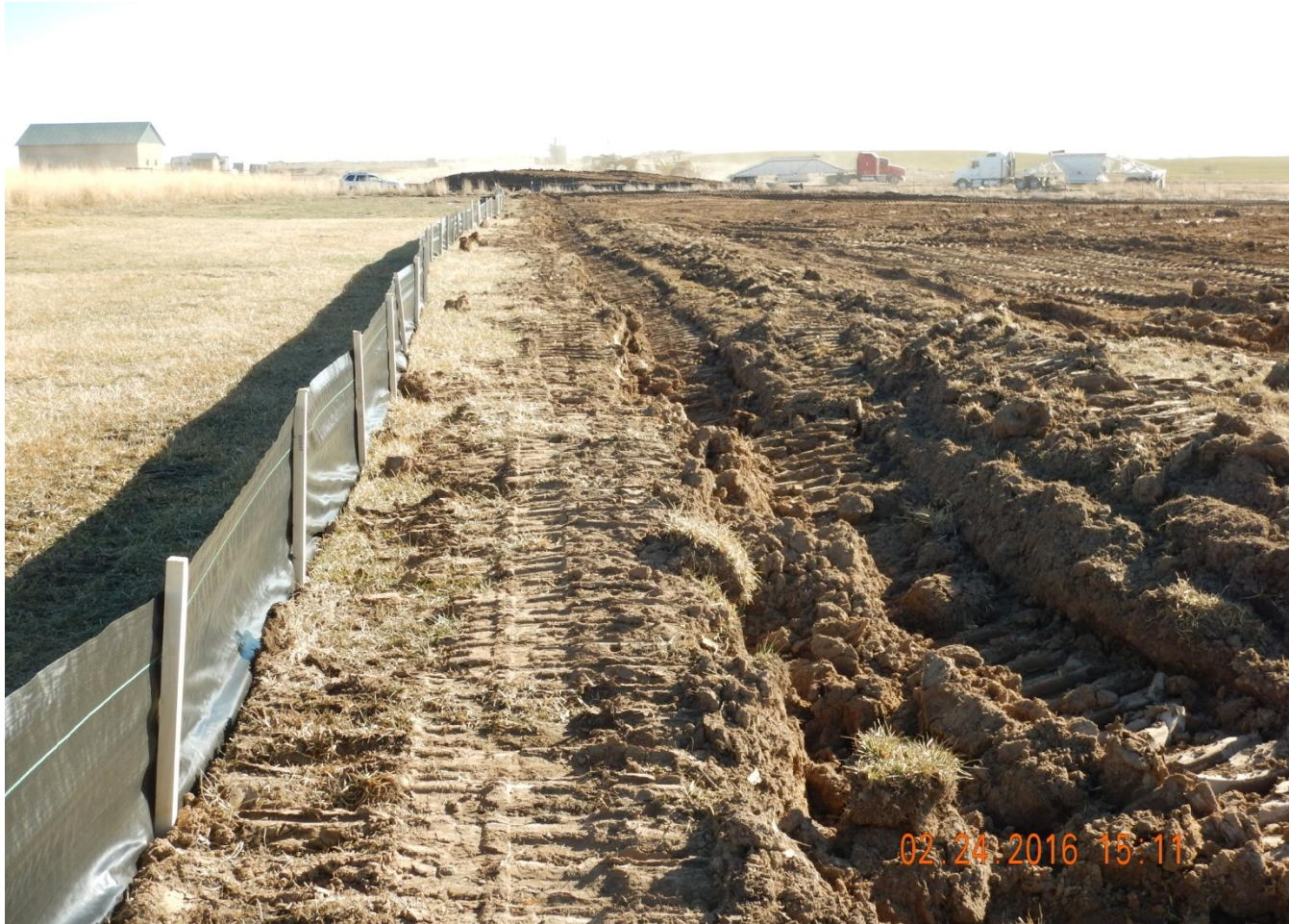
Photo 5. Photo taken from northeast location, facing South. Stormwater and sediment control BMPs installed in center of photo.
