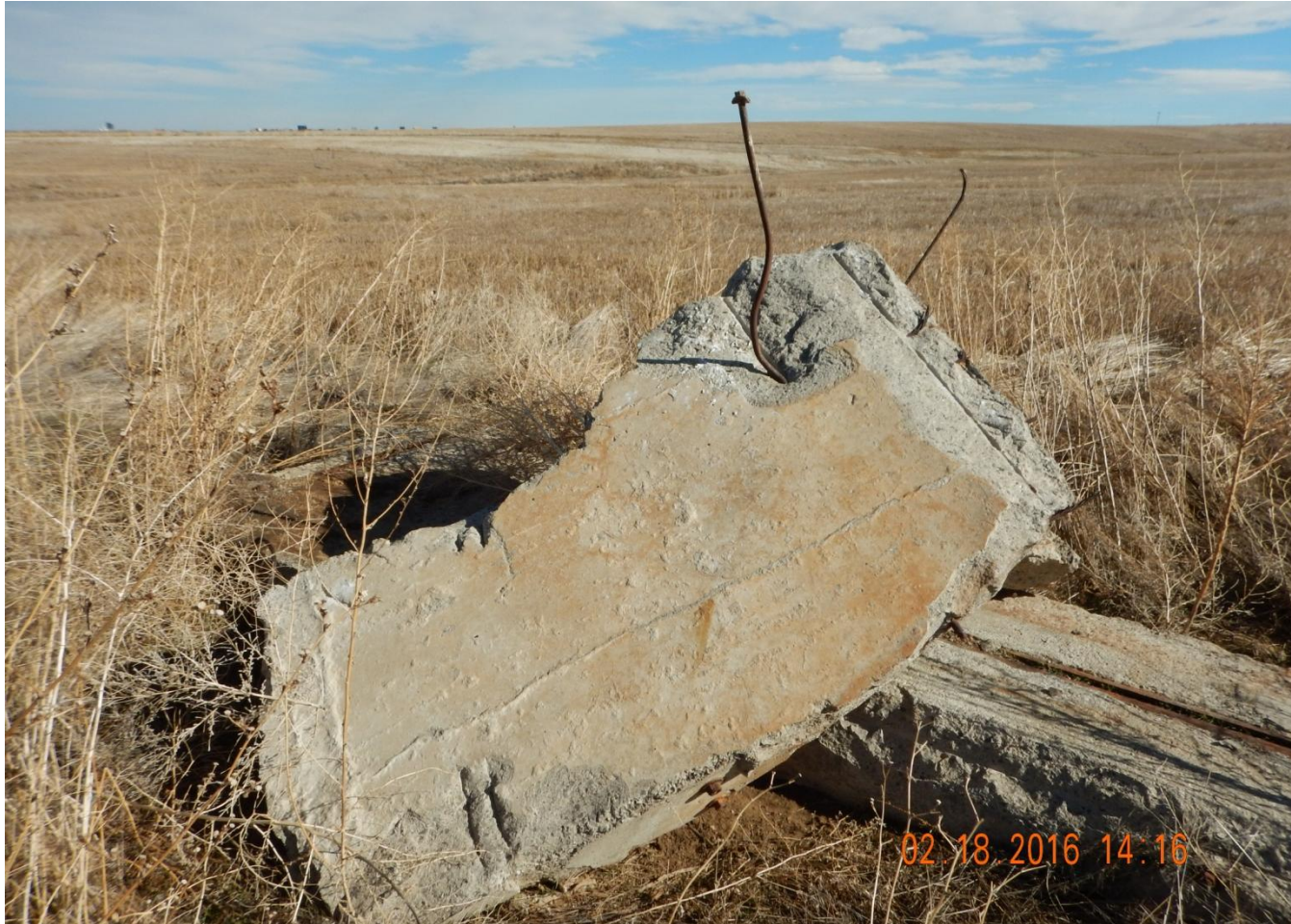
Photo 6. Photo taken from center of location. Waste material left behind.
