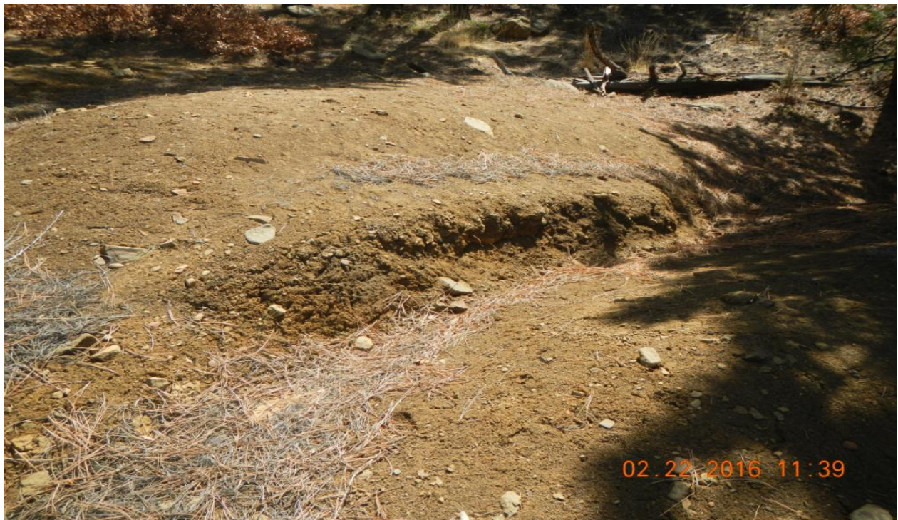
photo 8: Signs of erosion off the southeast corner of the location.
