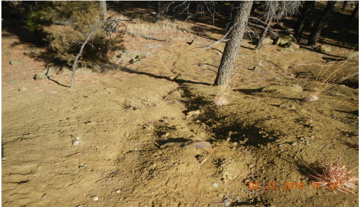
photo 5: Signs of erosion off the north side of the location.
