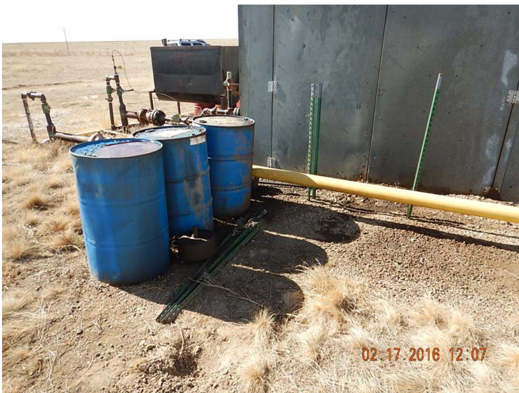
Figure 4 – Barrels leaking and stained soil on east side of compressor.
