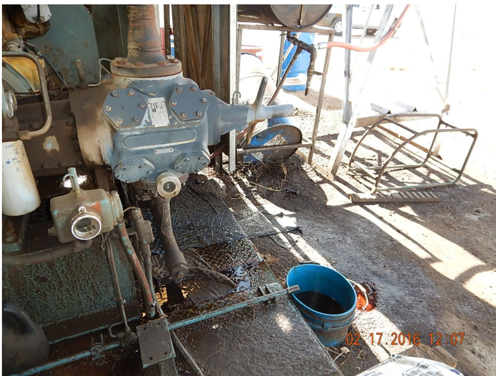
Figure 6 – Compressor leaking oil on west side of facility.
