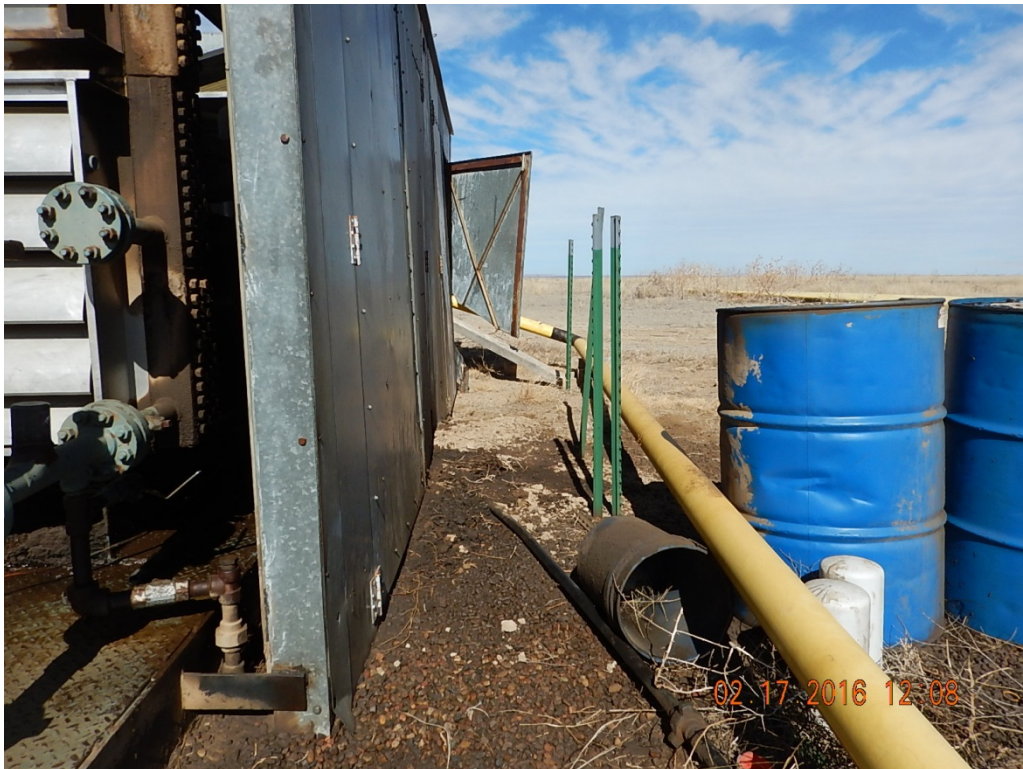
Figure 5 – Stained soil on east side of compressor.
