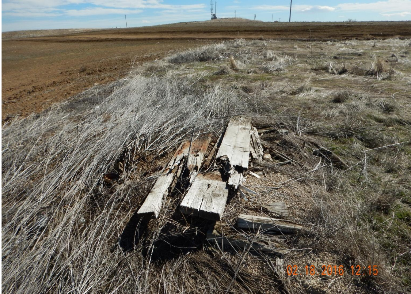
Photo 4. Photo taken from north well location, facing East. Well location not properly reclaimed-not recontoured and waste material left behind.
