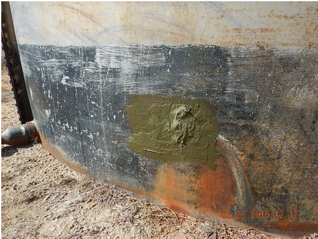
Figure 3 – Leak in produced water tank has been repaired and stained soil removed.
