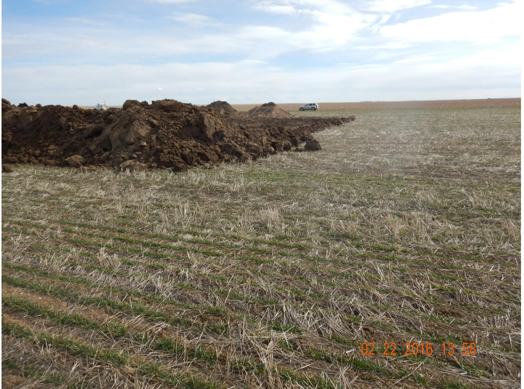
Figure 15: Photo taken from the northwest corner of location, facing south. Photo shows perimeter stormwater and sediment controls have not been installed.
