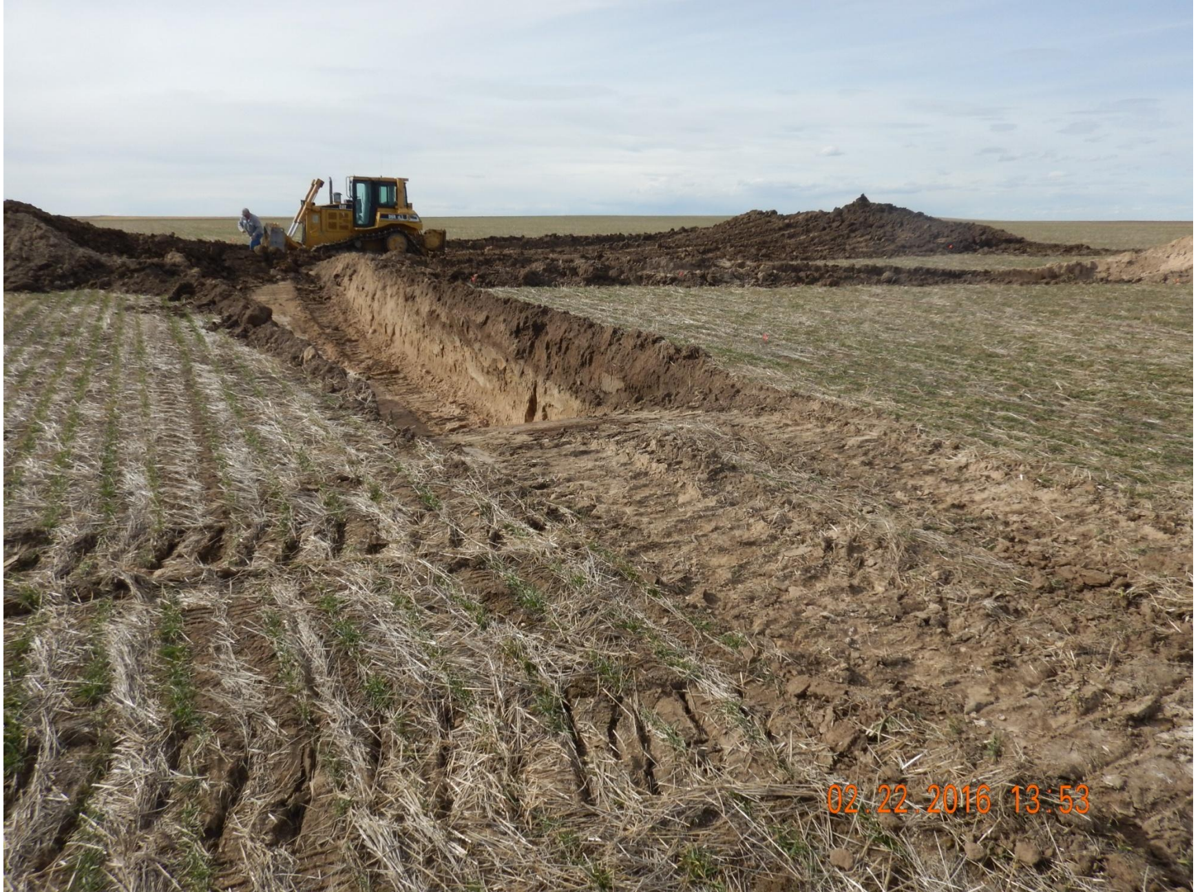
Figure 10: Photo taken from the southeast corner of location, facing west. Photo shows perimeter stormwater and sediment controls have not been installed.
