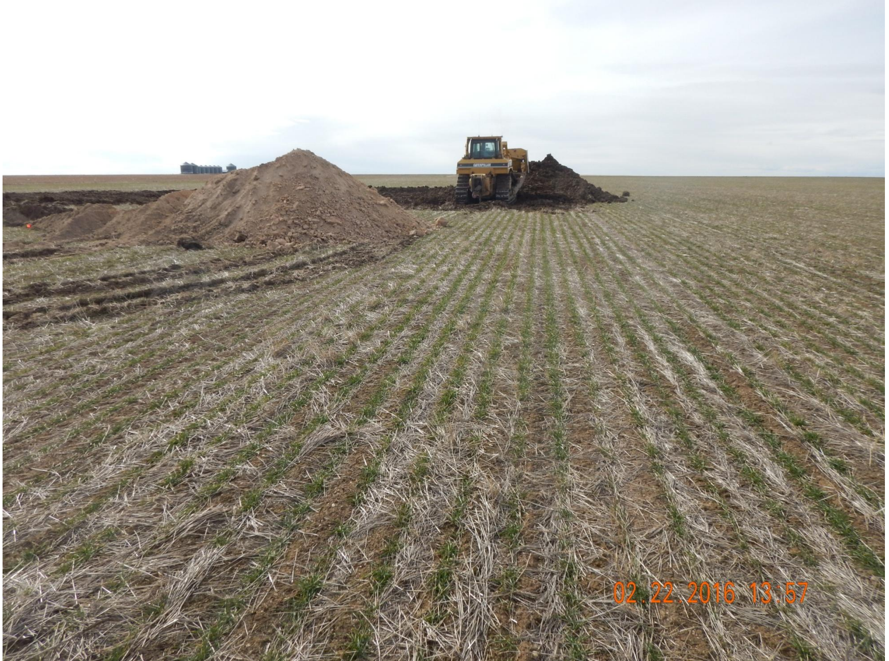
Figure 13: Photo taken from the northeast corner of location, facing west. Photo shows perimeter stormwater and sediment controls have not been installed.
