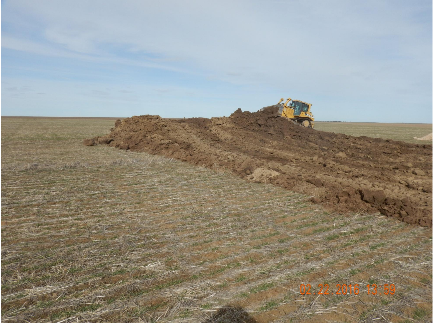
Figure 7: Photo taken from the west end of the location, facing northeast. Photo shows perimeter stormwater and sediment controls have not been installed.
