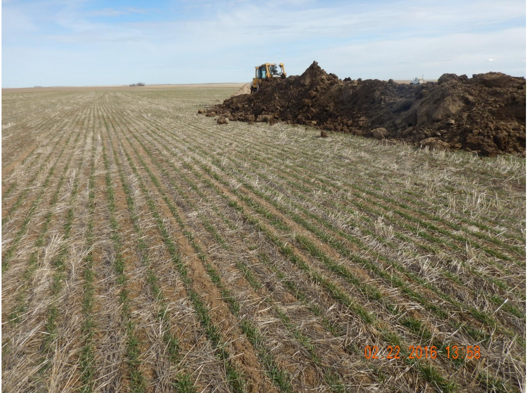
Figure 14: Photo taken from the northwest corner of location, facing east. Photo shows perimeter stormwater and sediment controls have not been installed.
