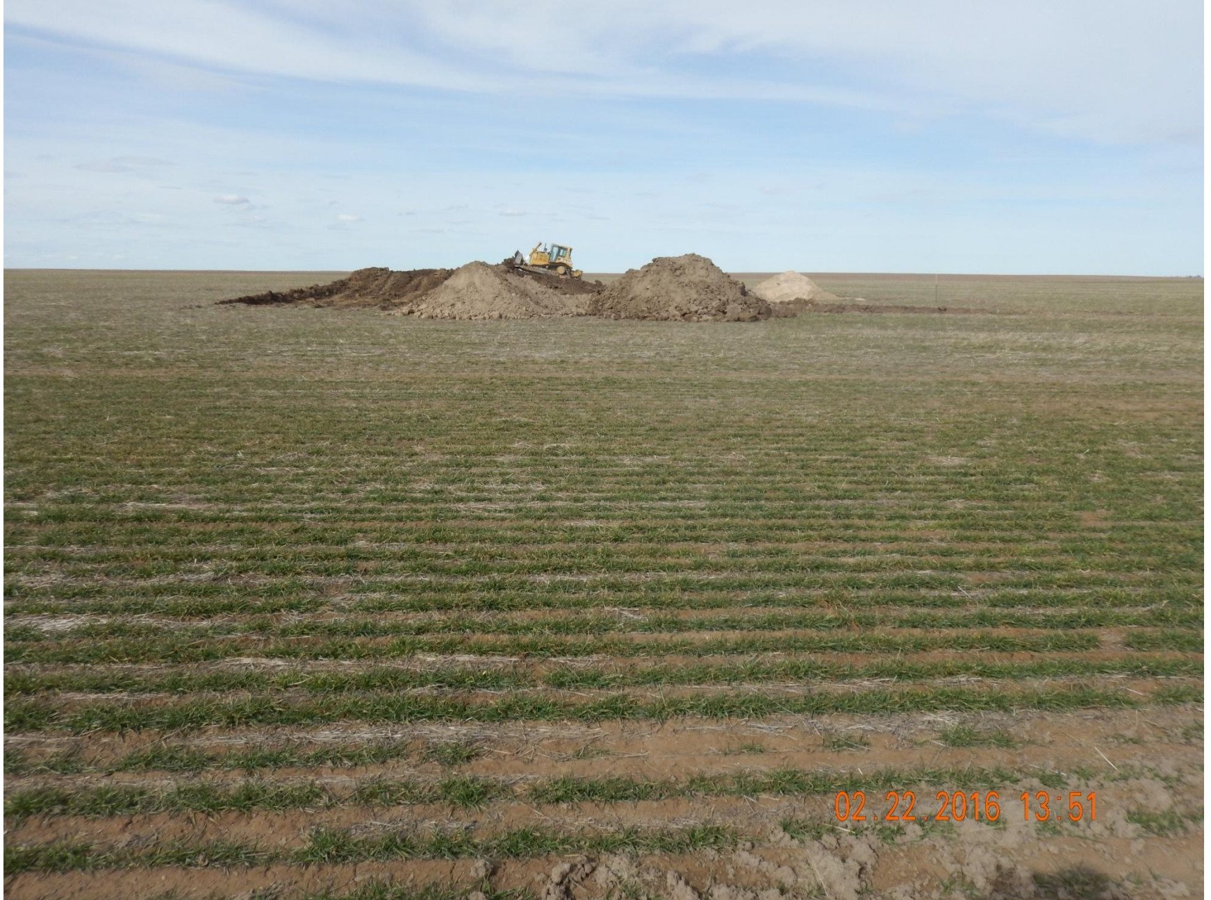
Figure 1: Photo taken from access road, south of location facing north. Photo of construction in process. Note stormwater and sediment control BMPs not in place.
