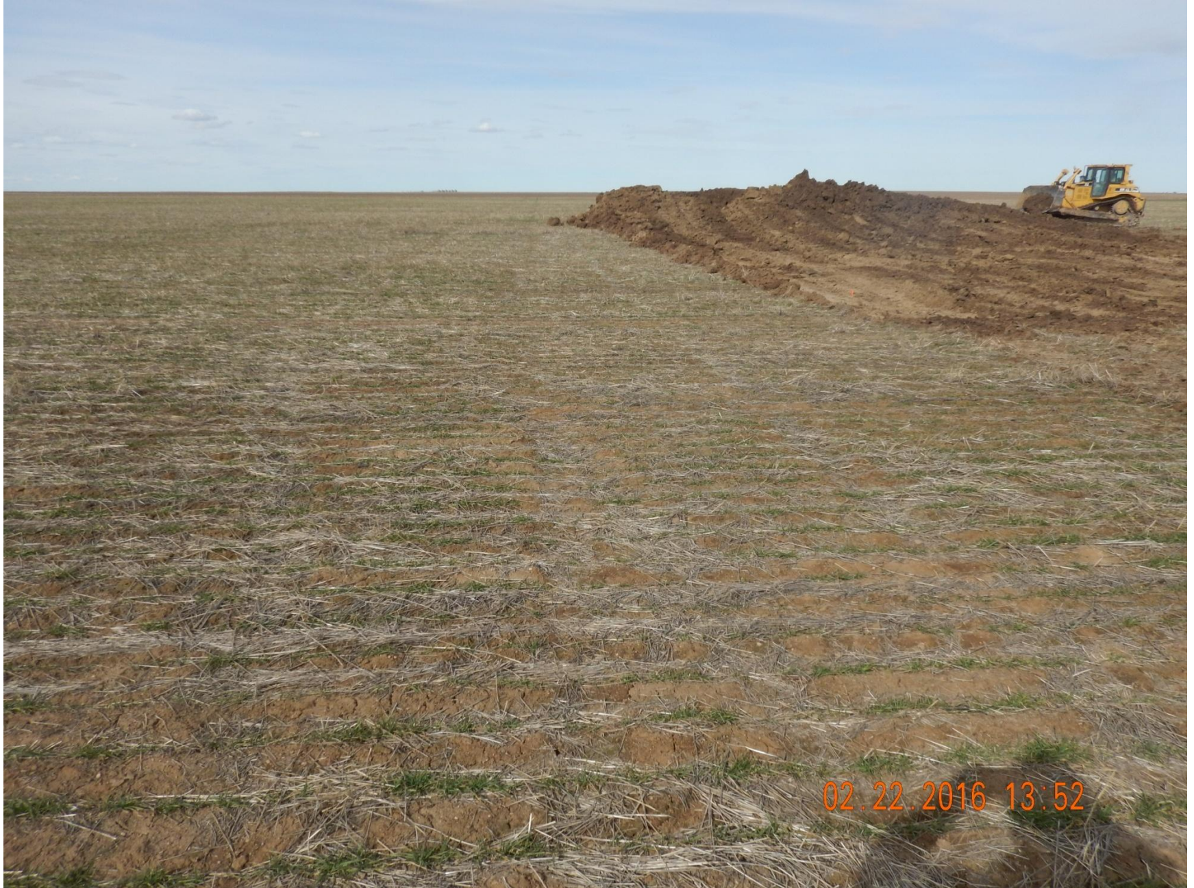
Figure 8: Photo taken from the southwest corner of location, facing north. Photo shows perimeter stormwater and sediment controls have not been installed.
