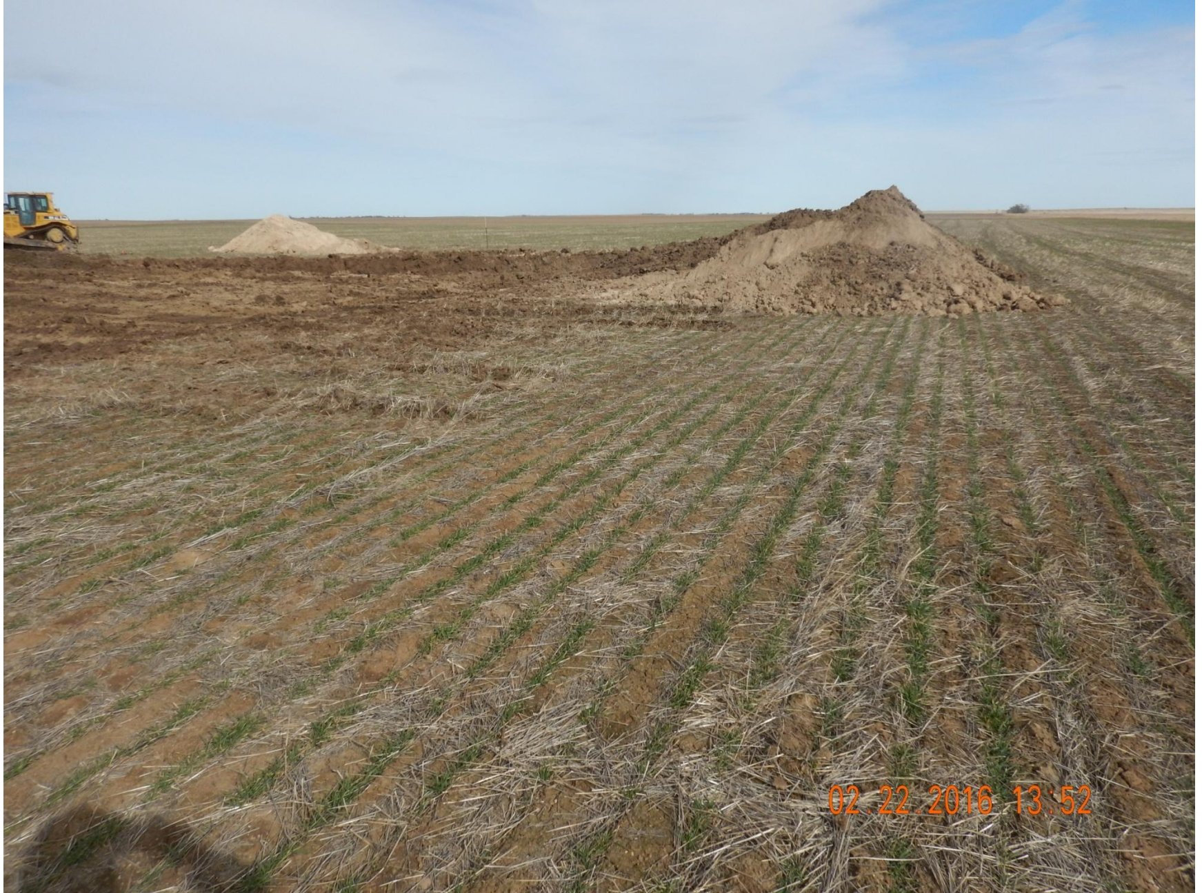
Figure 7: Photo taken from the southwest corner of location, facing east. Photo shows perimeter stormwater and sediment controls have not been installed.
