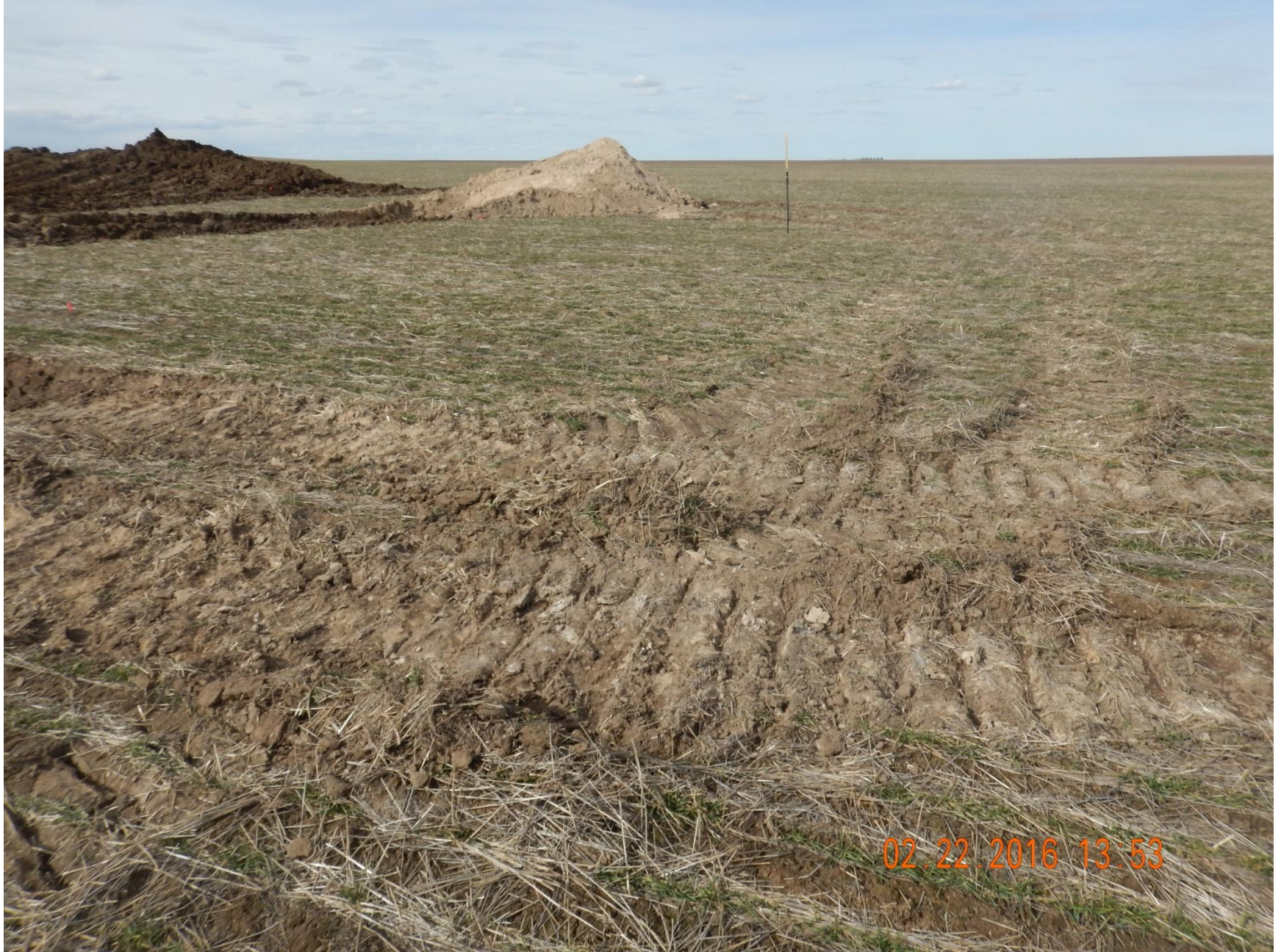
Figure 9: Photo taken from the southeast corner of location, facing north. Photo shows perimeter stormwater and sediment controls have not been installed.
