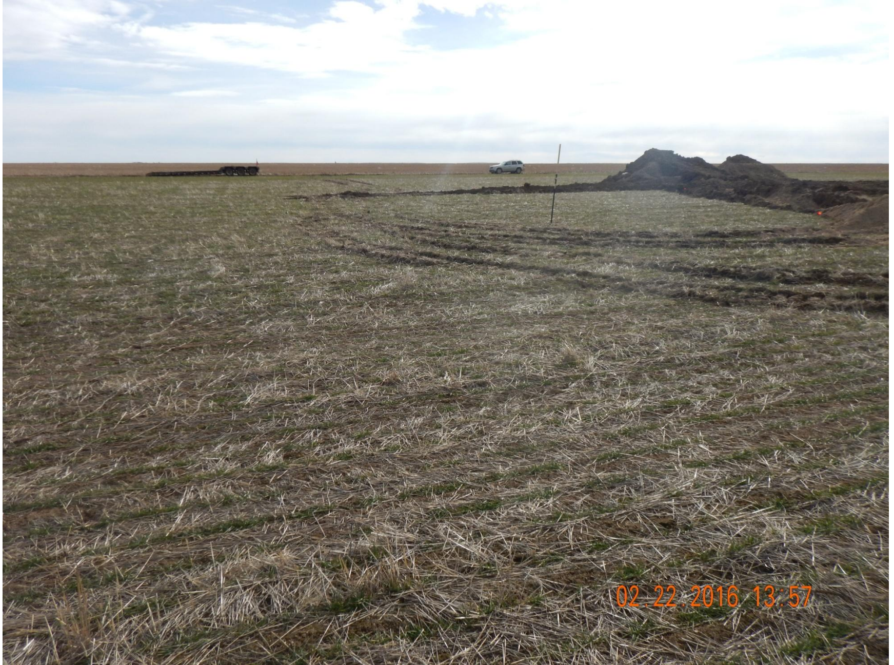
Figure 12: Photo taken from the northeast corner of location, facing south. Photo shows perimeter stormwater and sediment controls have not been installed.
