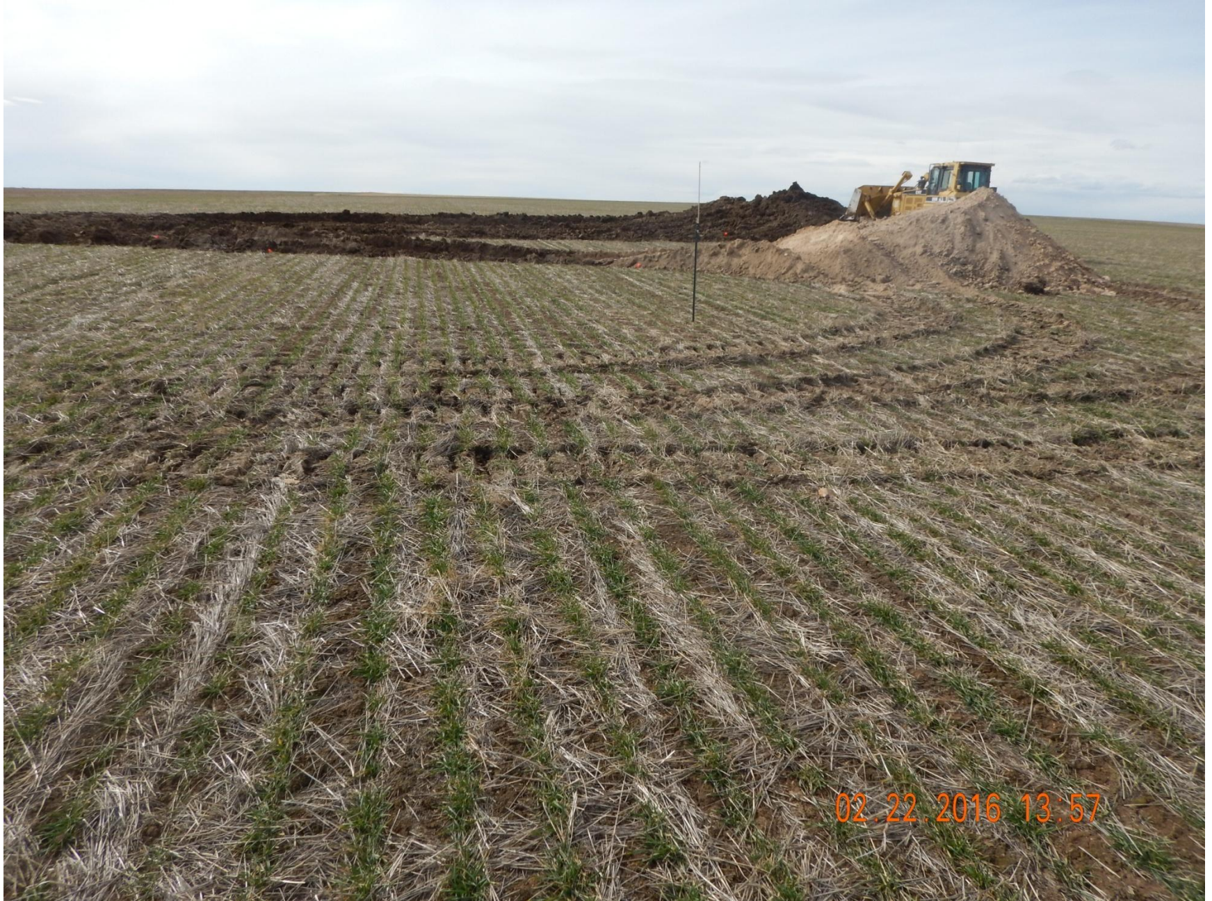
Figure 11: Photo taken from the east end of location, facing west. Photo shows perimeter stormwater and sediment controls have not been installed.
