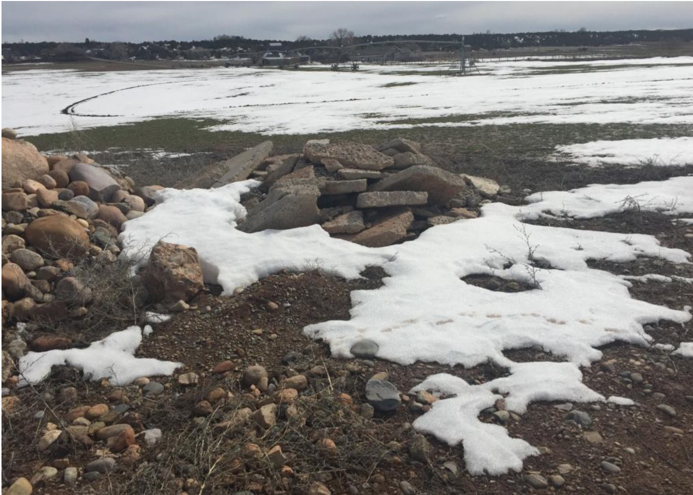
Photo 2. View of cement debris in southeastern portion of the project area.
