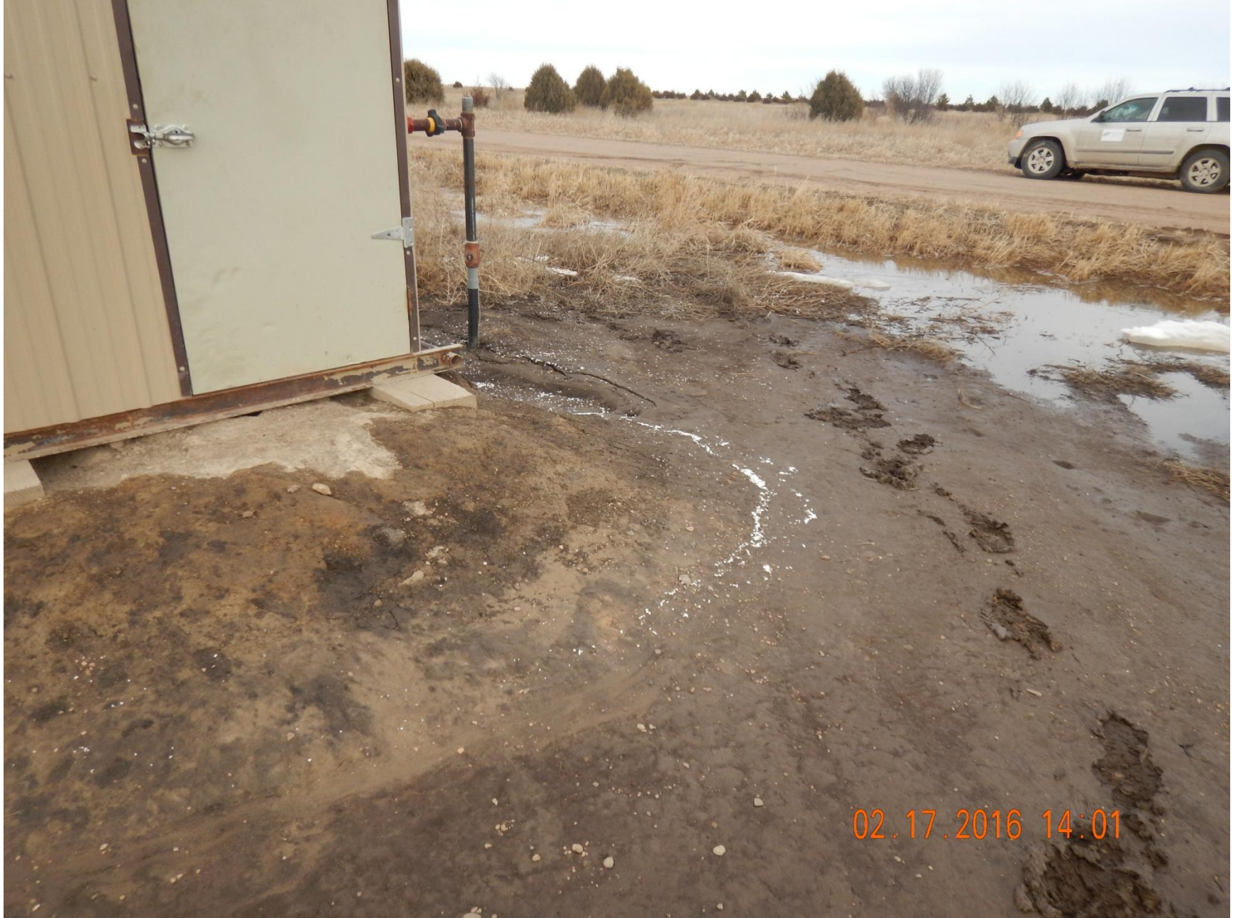
Figure 6: Photo taken from the east end of location, facing northeast. Photo shows erosion at gas meter run. White material appears to be pieces of styrofoam.
