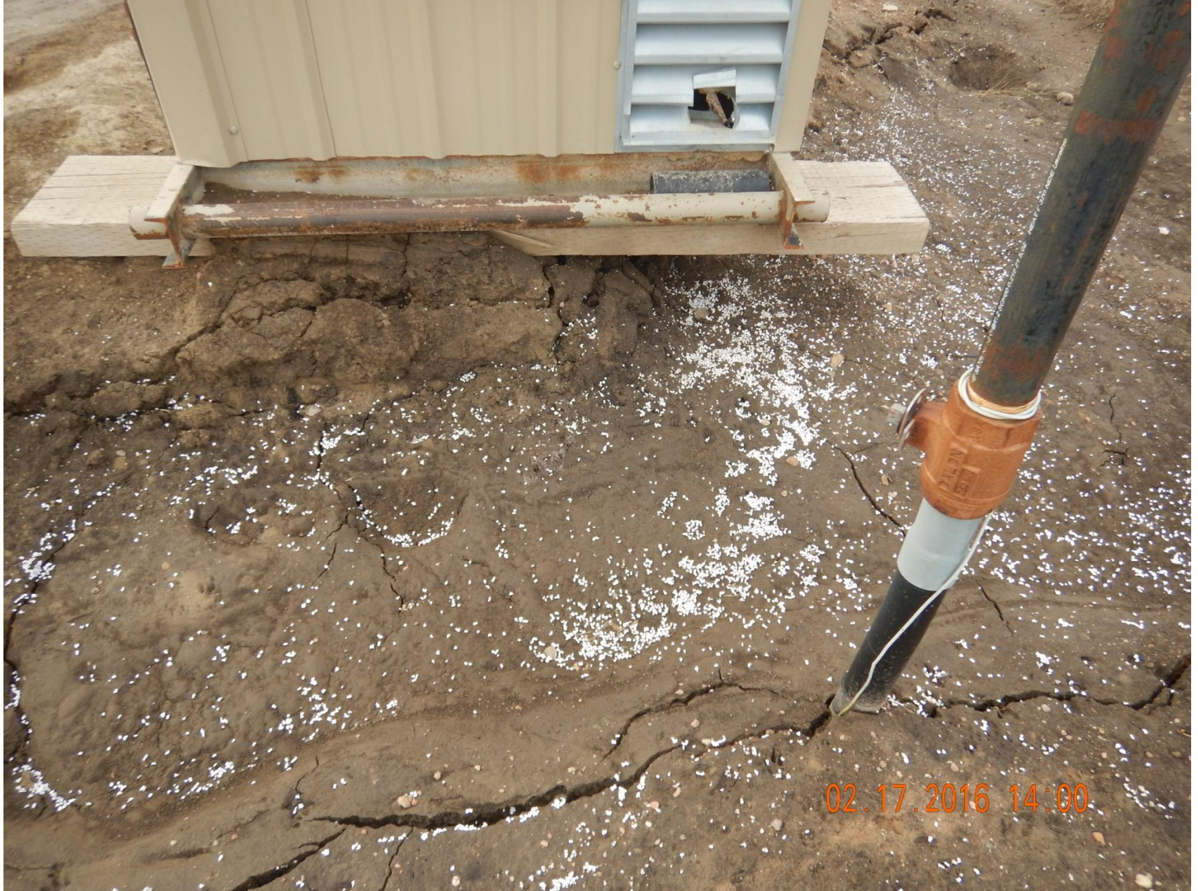
Figure 4: Photo facility on the east end of the location, facing west. Photo shows erosion occurring at gas meter run. White materials at arrow appears to be pieces of styrofoam.
