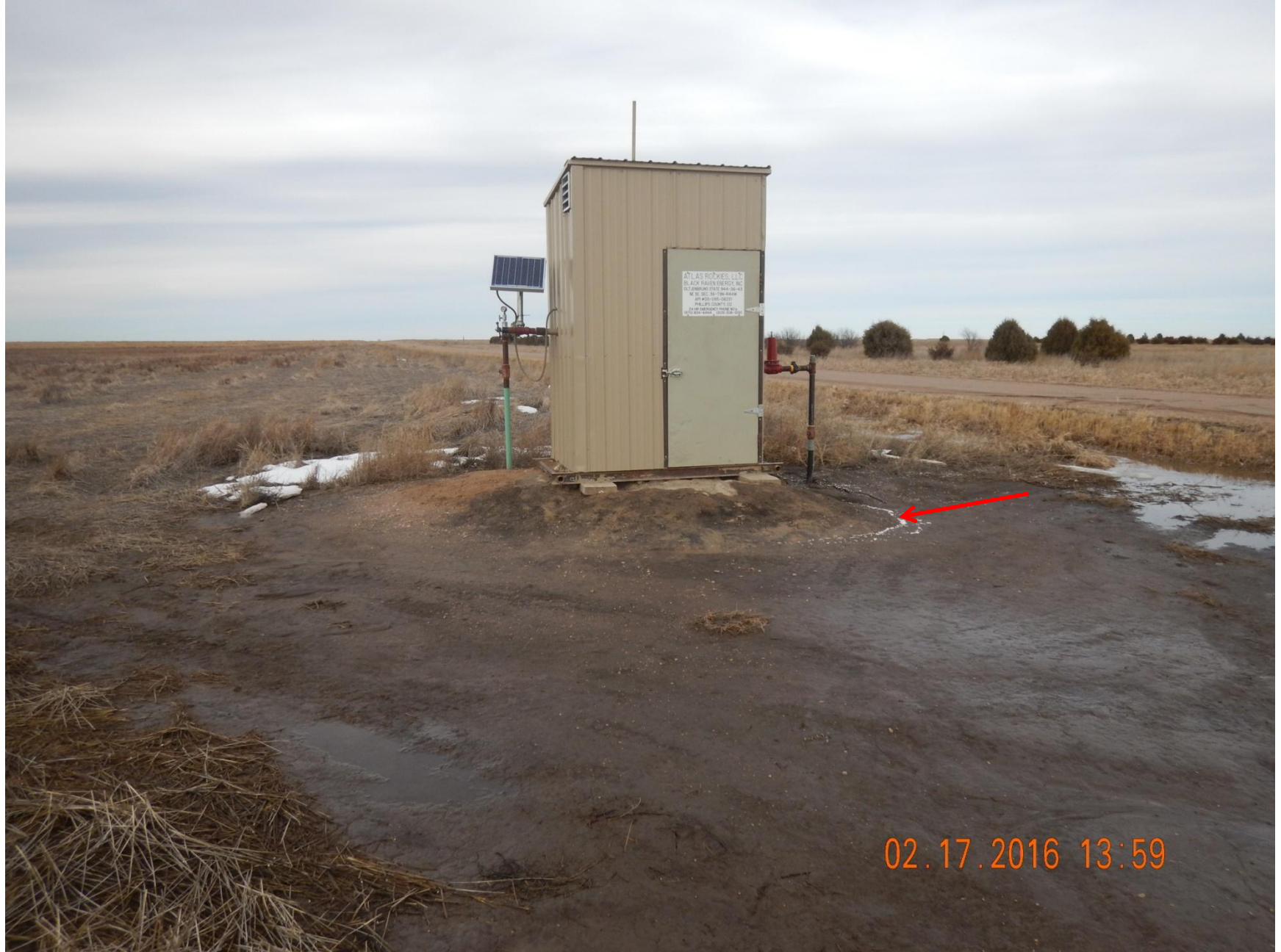
Figure 2: Photo of gas meter run on the east end of the location, facing north. Photo shows location was recently inundated with water. White substance (arrow) appears to be pieces of styrofoam.
