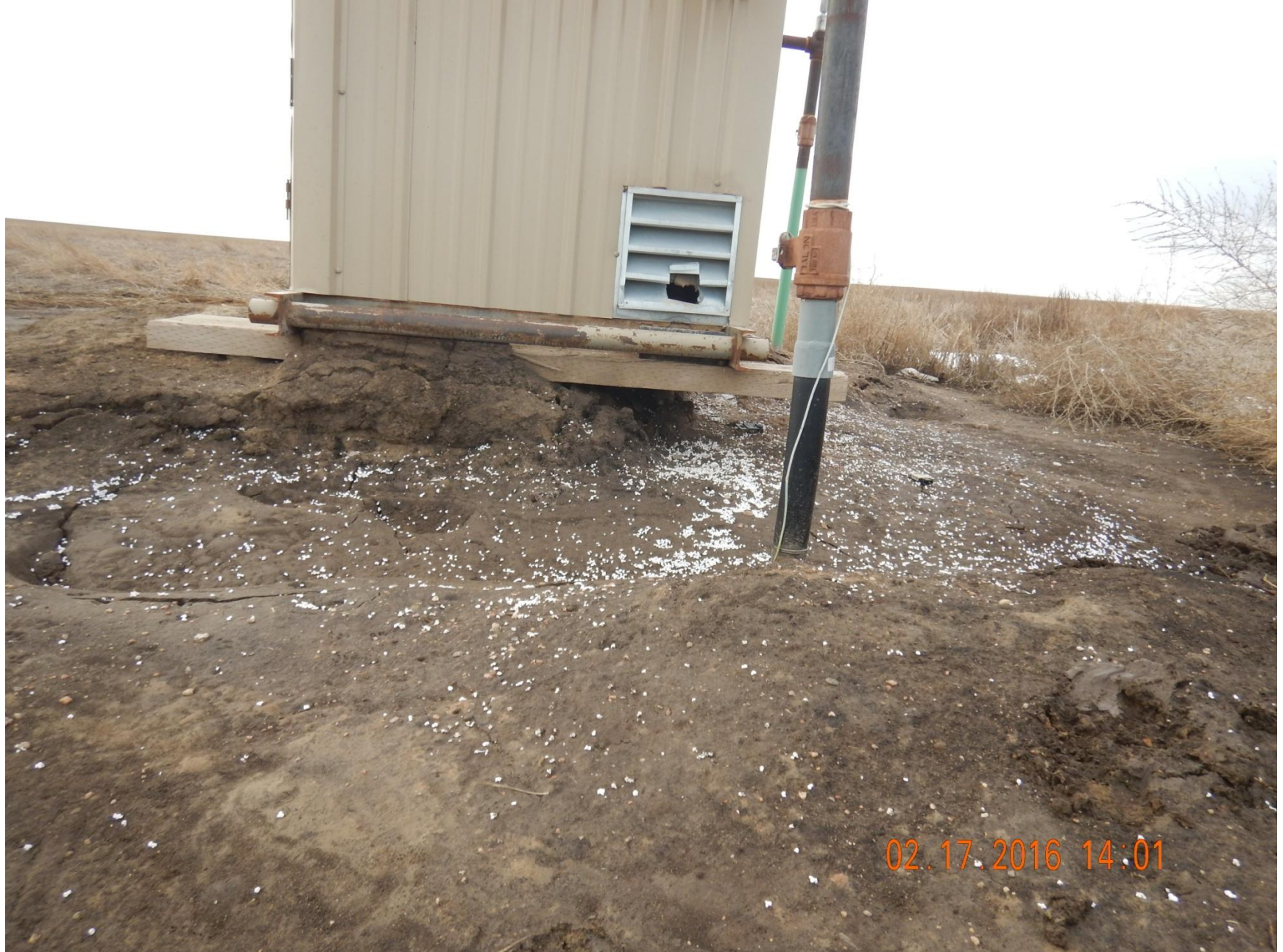
Figure 5: Photo taken from the east end of location, facing west. Photo shows erosion at gas meter run. White materials at arrow appears to be pieces of styrofoam.
