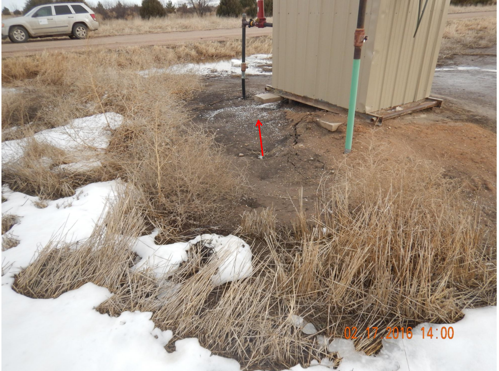
Figure 3: Photo facility on the east end of the location, facing southeast. Photo shows erosion occurring at gas meter run. White substance at arrow appears to be pieces of styrofoam.
