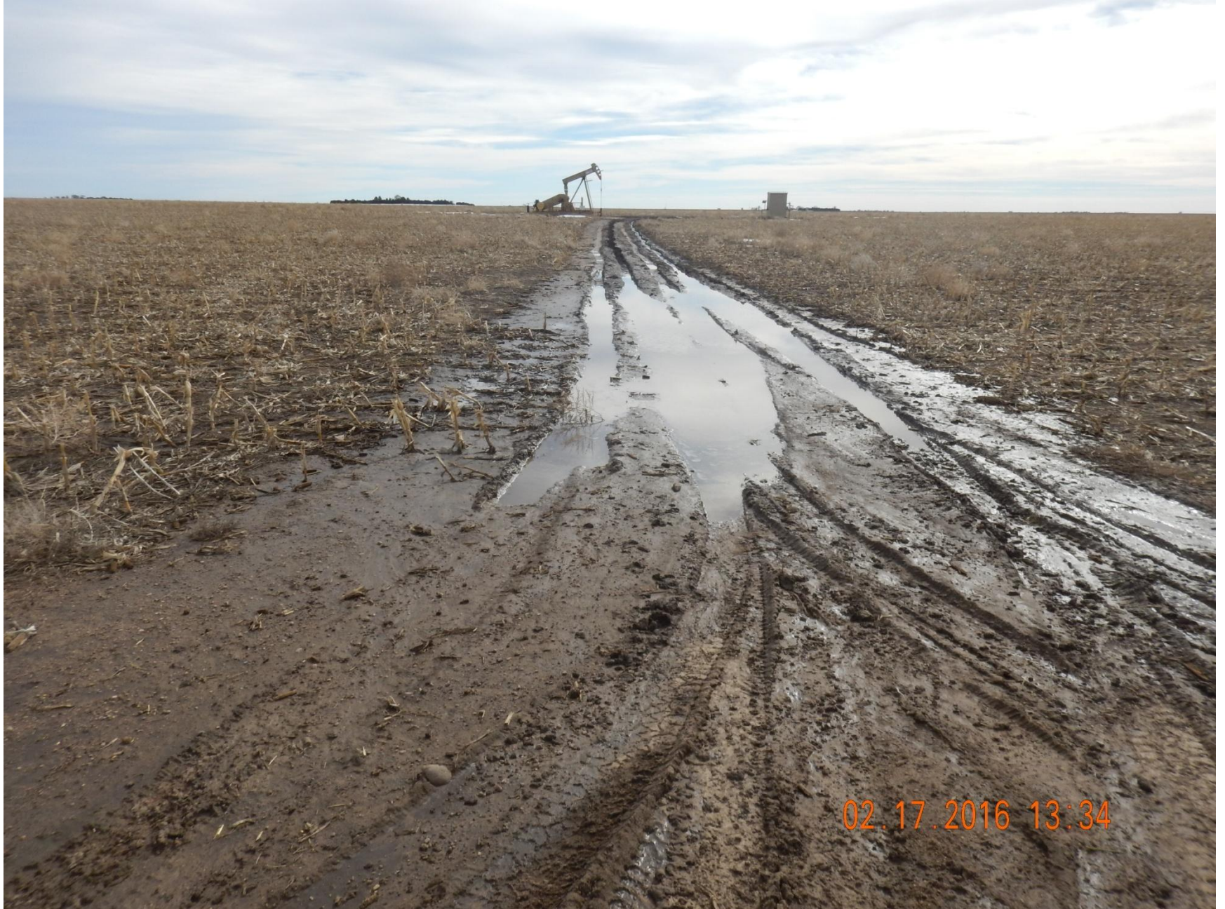
Figure 2: Photo taken from access road, north of location facing south. Photo shows water pooling in access road and vehicle rutting in road.
