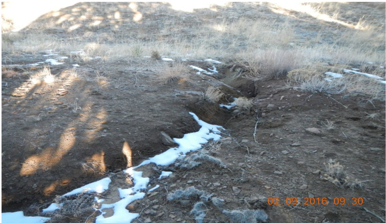
photo 6: Erosion channel formed at the south side of the location.
