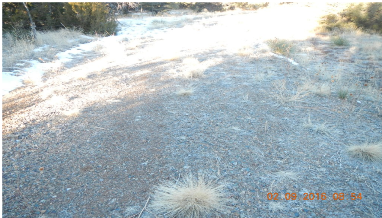
photo 2: The access road has not been recontoured and reclaimed. Gravel remains along the access road.
