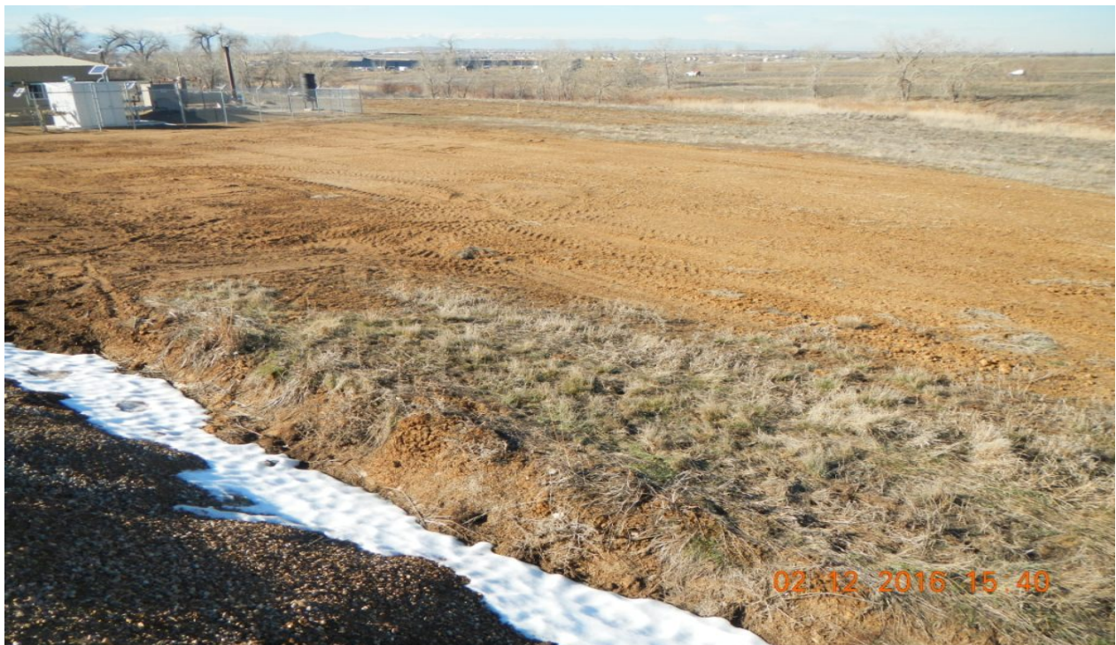
photo 10: Facing northwest at the north side of the location. Disturbance is susceptible to erosion and needs to be reclaimed.
