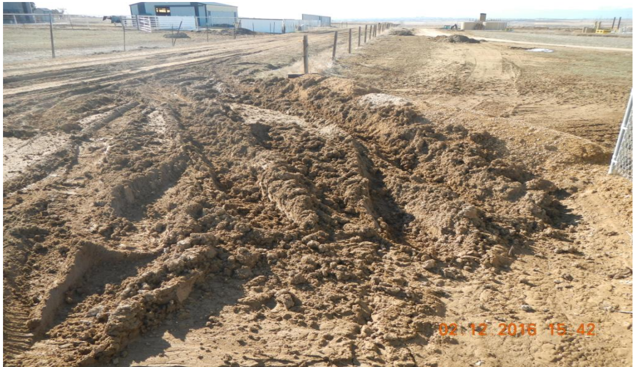
photo 13: Vehicle tracking and rutting occurring near the tank battery and access road.
