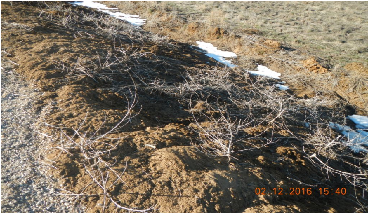
photo 9: Signs of erosion occurring off the north side of the pad which is not adequately stabilized.
