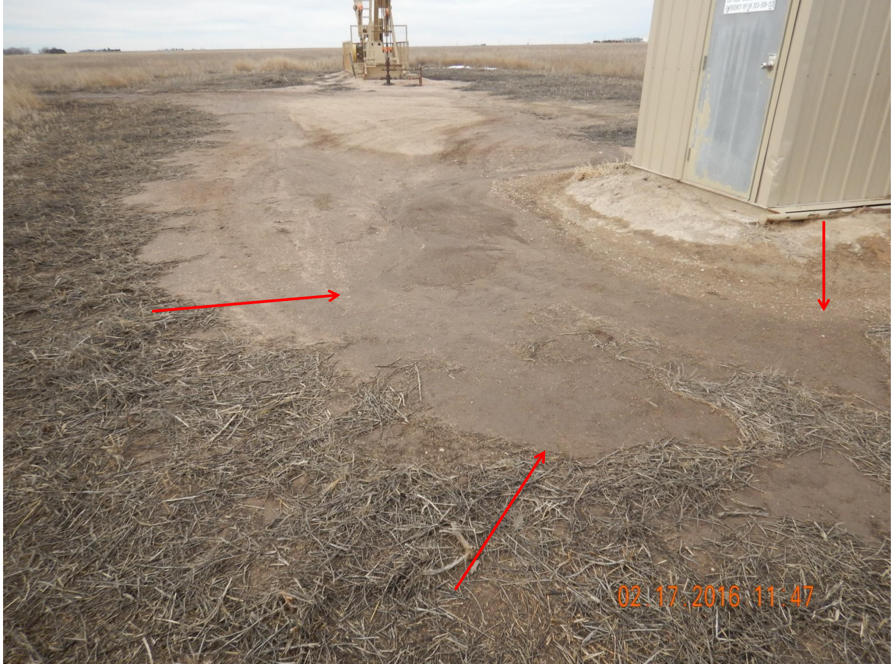
Figure 11: Photo taken from the east end of project area, facing west. Photo shows stormwater erosion on location. Arrows shows water movement patterns and alluvial deposition.
