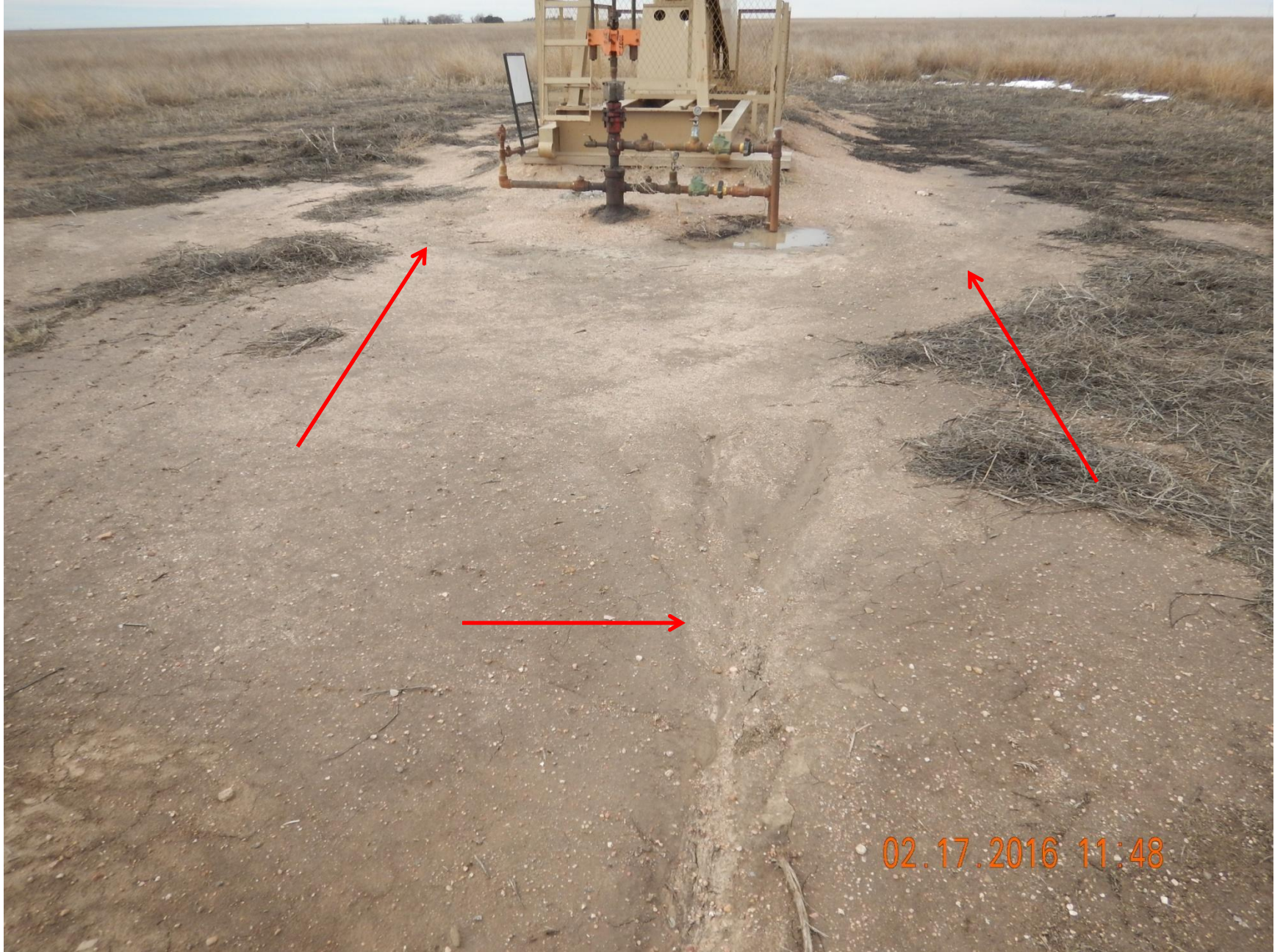
Figure 14: Photo taken from the central portion of the location, facing west. Photo shows erosion patterns on location.
