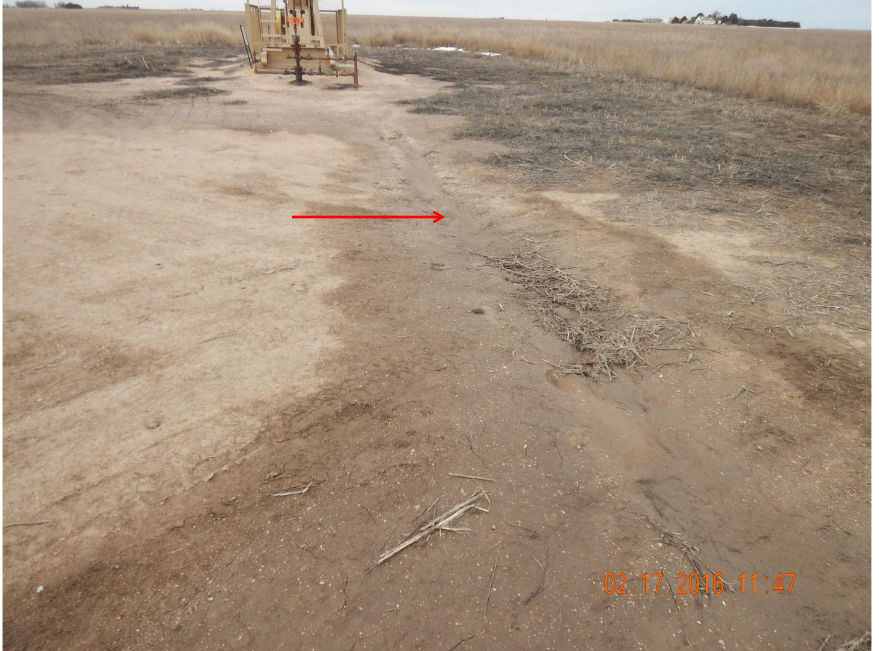
Figure 13: Photo taken from eastern end of the project area, facing west. Photo shows erosion patterns on location.
