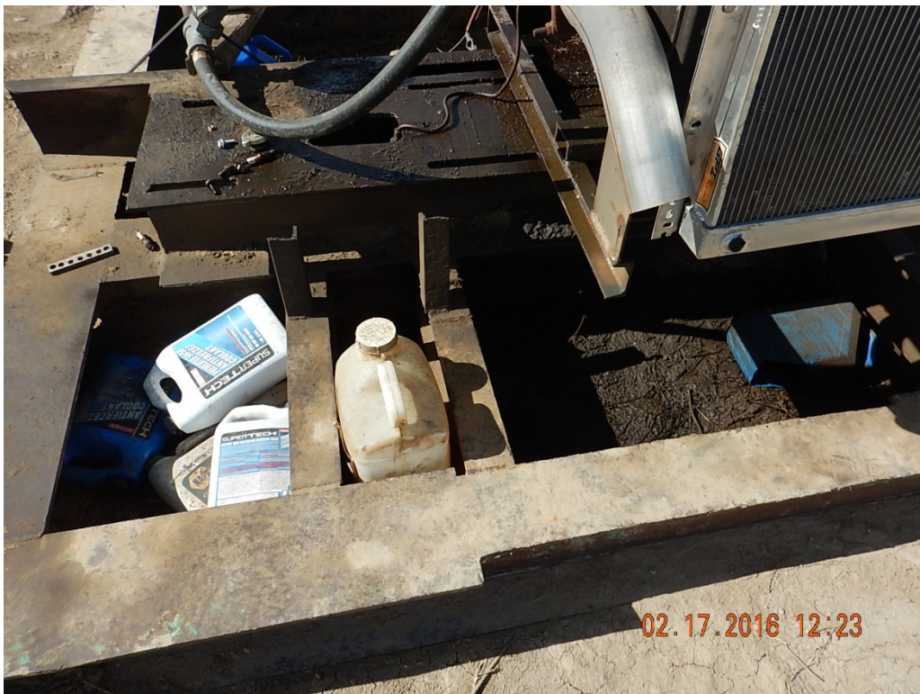
Figure 4 – Stained soil under generator, oil covered equipment and trash left on site.
