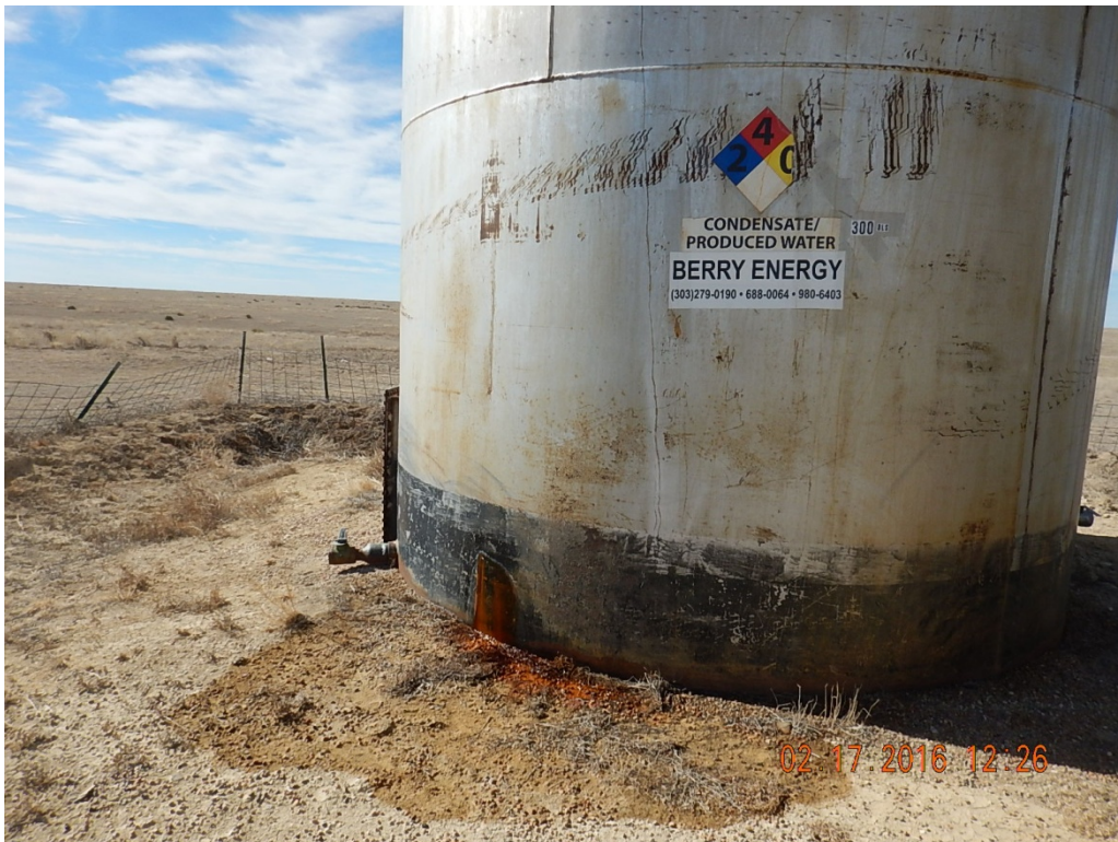
Figure 5 – Produced water tank actively leaking.
