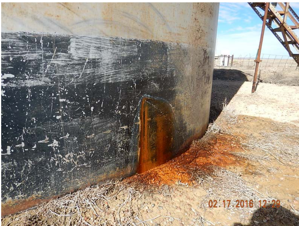
Figure 6 – Produced water tank actively leaking.
