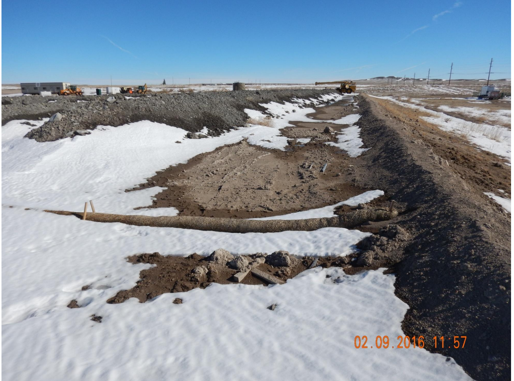
Figure 18: Photo taken from southern end of location, facing east. Photo of drill cuttings and waddles.
